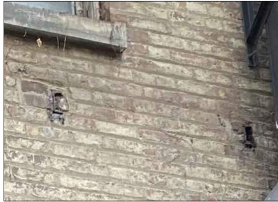
EXISTING BRICK L1 - L5
