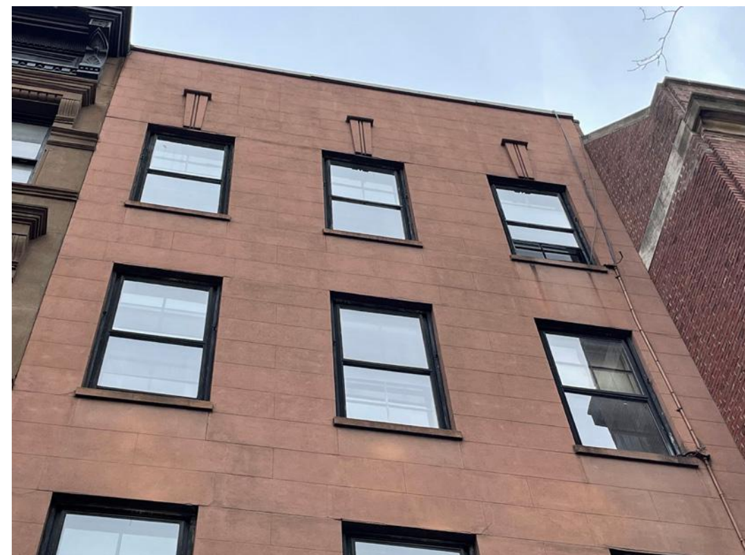
Detail view of the upper stories.
