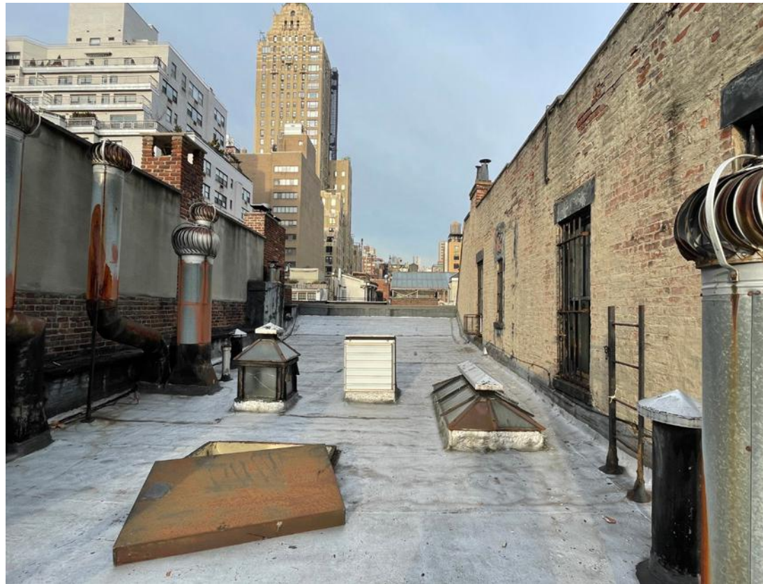
View of the roof looking north, towards the front facade.
