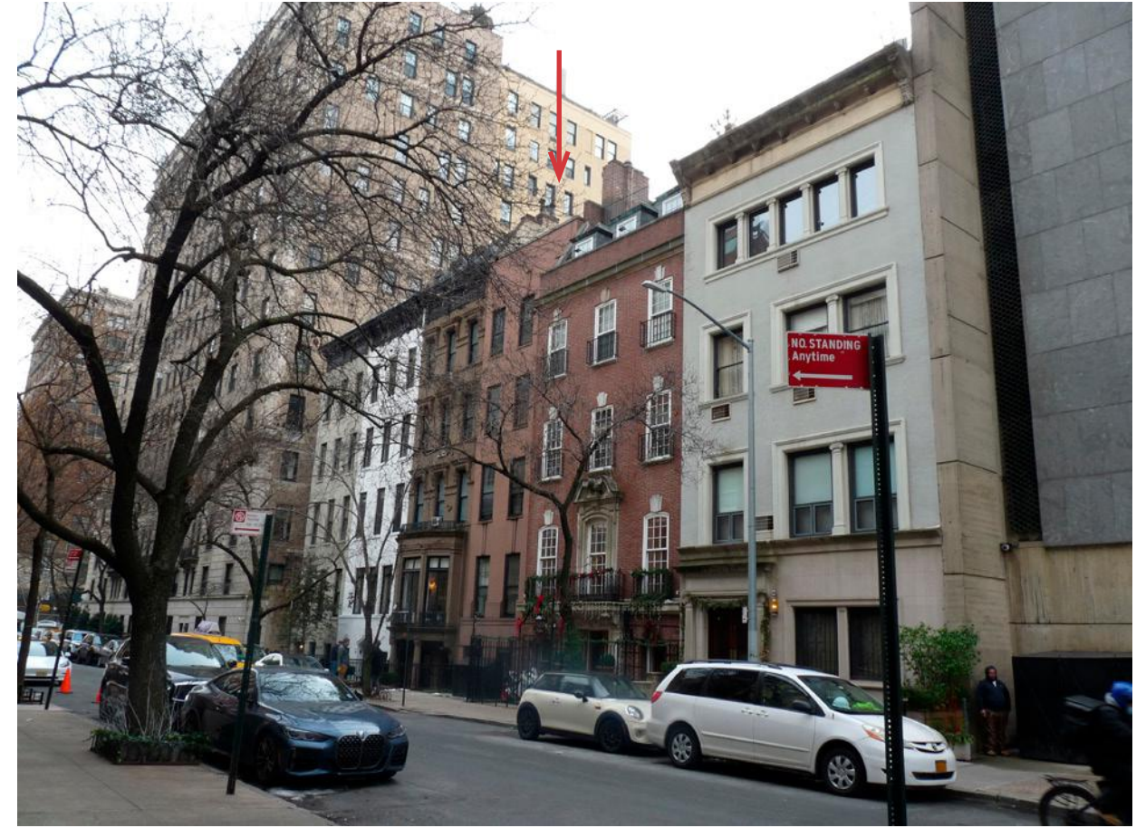
View of the north side of East 75th Street between Park Ave. and Madison Ave. looking east.
