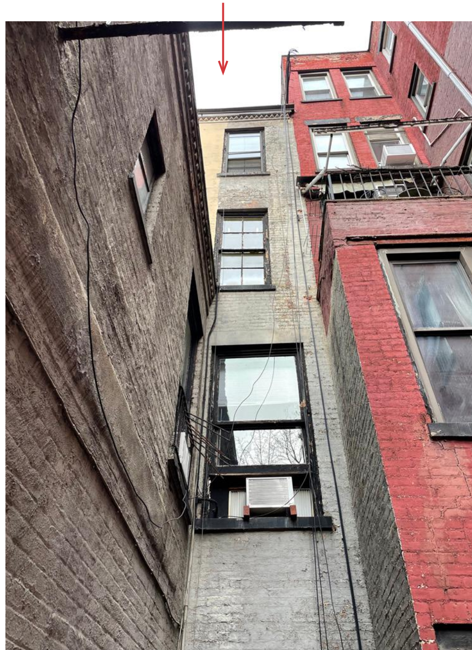
View of the rear elevation from the roof of the one-story rear extension.
