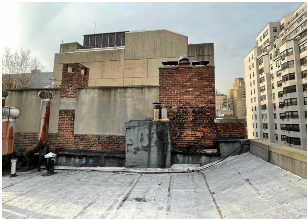
View of the roof looking west, showing Marcel Breuer's Whitney Museum in the background.
