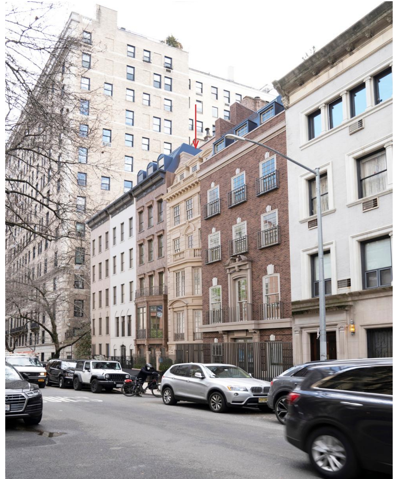
View of the north side of East 75th Street between Park Ave. and Madison Ave. looking east.
