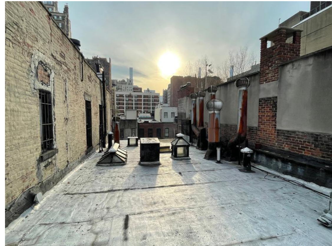
View of the roof looking south, towards the rear.
