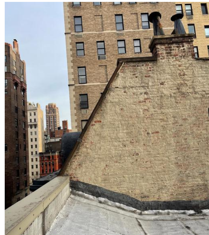
View of the roof looking east.
