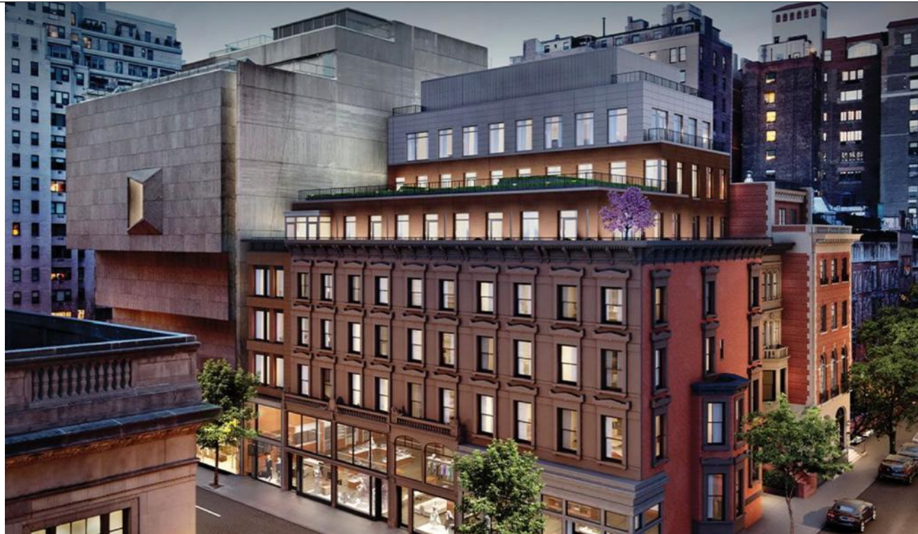
1) 933 MADISON AVENUE AND 33 EAST 74TH STREET: Rooftop addition approved in 2012.
