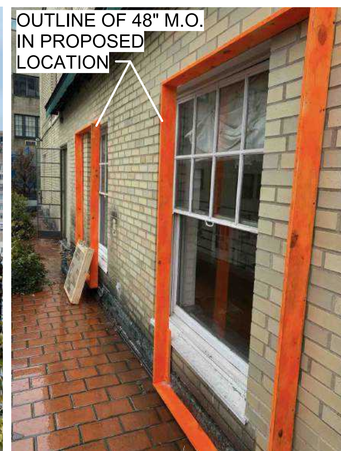
C PHOTO CLOSE UP RED FRAMES - LOOKING SOUTH NOTE: RED FRAMES REPRESENT OUTLINE OF NEW TERRACE DOORS
