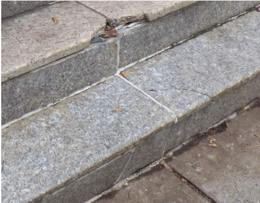
granite steps showing cracking, spalls and previous replacement
