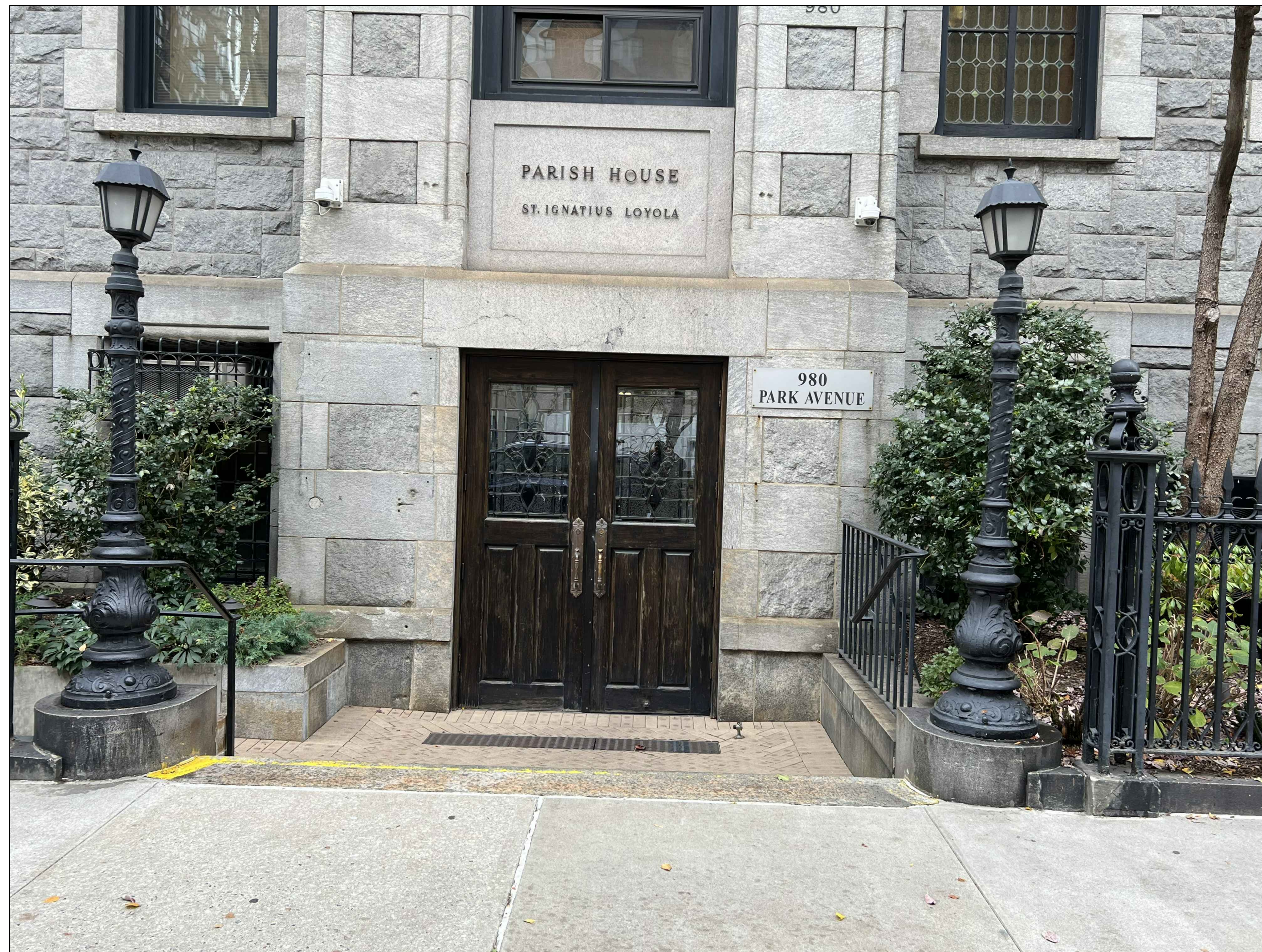
EXISTING ENTRANCE DOOR
