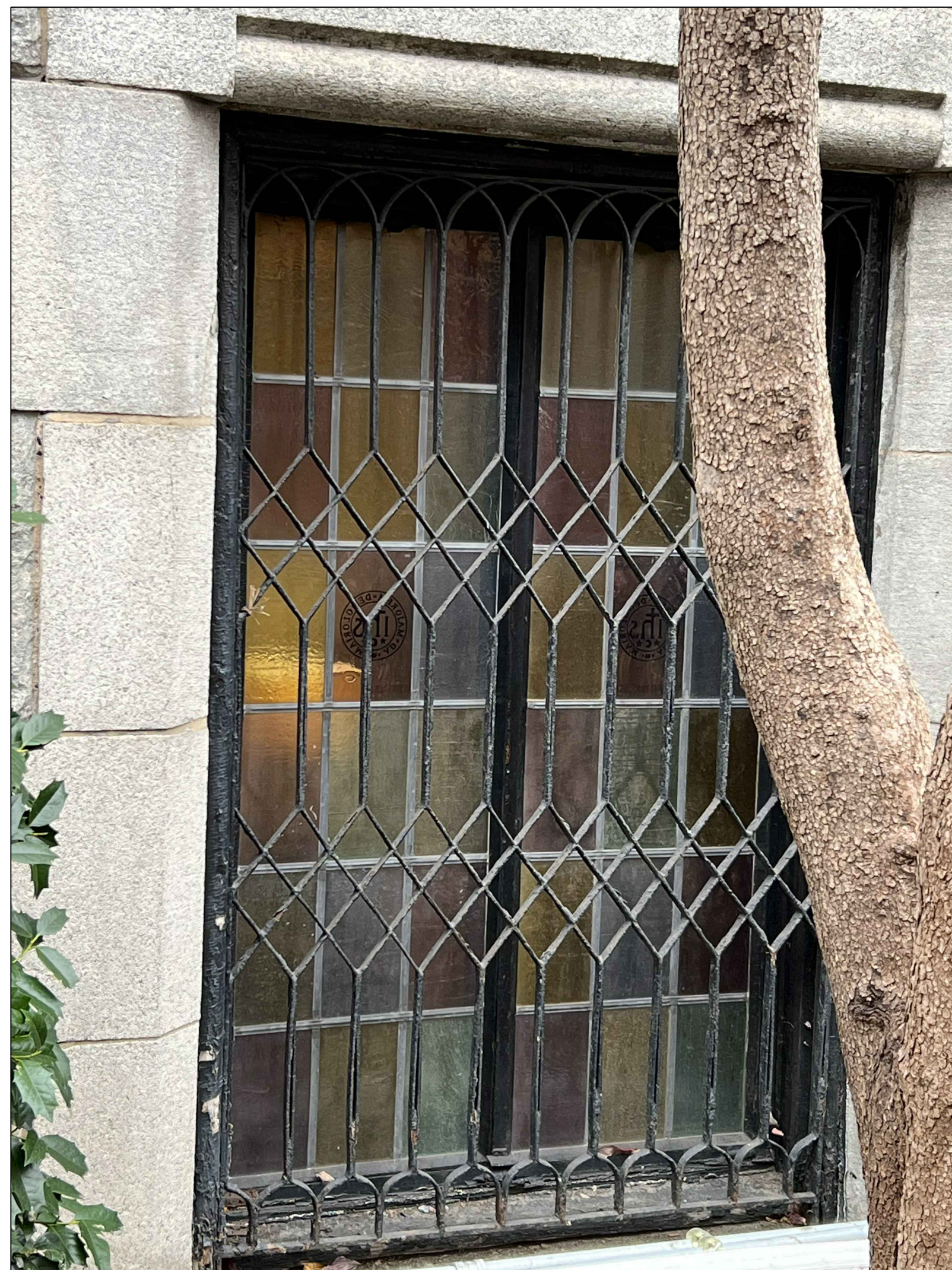
EXISTING WINDOW GRILLE
