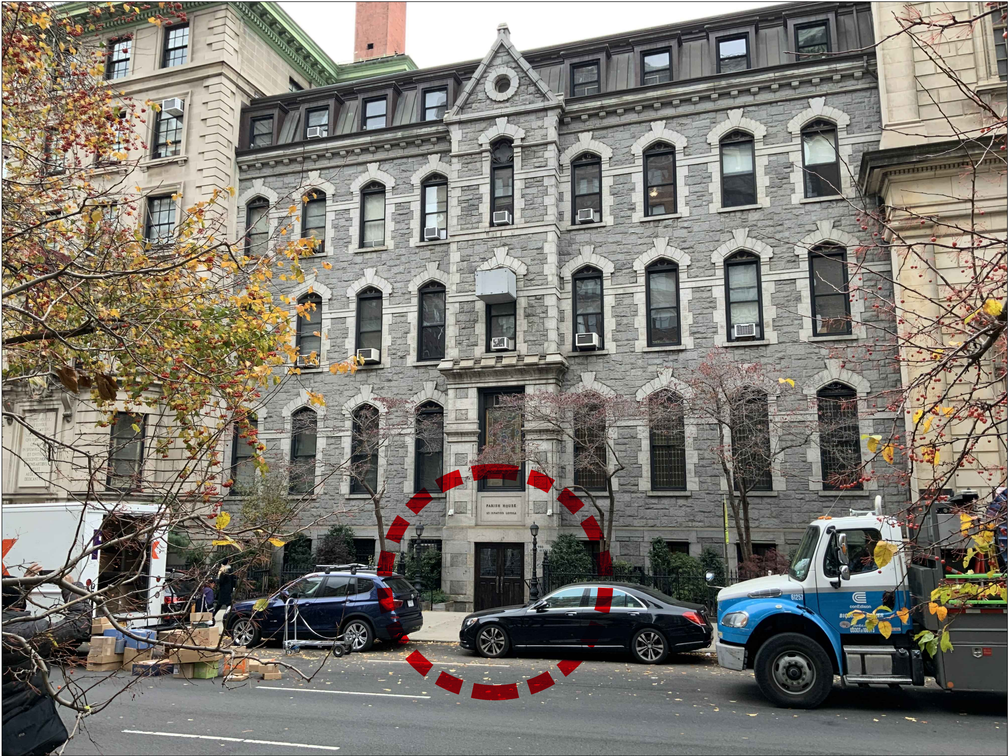
EXISTING OVERALL BUILDING PHOTO
