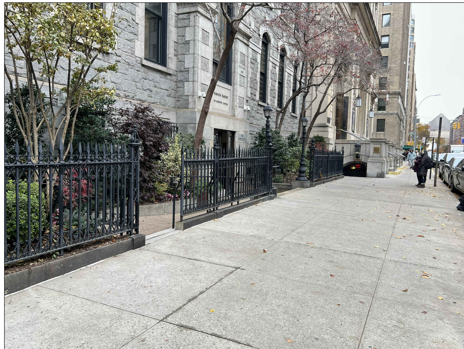
EXISTING GROUND LEVEL - LOOKING NORTH
