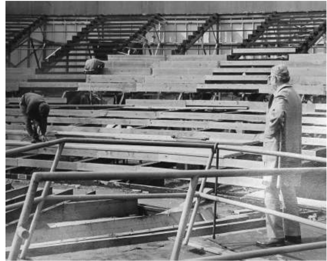
View of Stands during Rehabilitation, 1976 (NYPL) 1976
