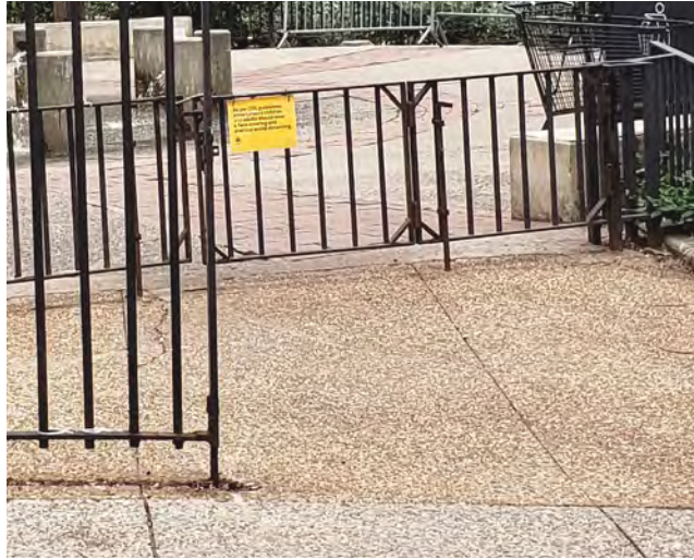
EXISTING - EXPOSED AGGREGATE CONCRETE PAVEMENT
