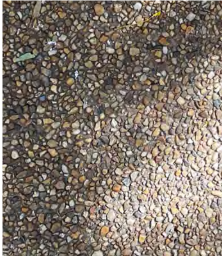
EXISTING - EXPOSED AGGREGATE CONCRETE PAVEMENT
