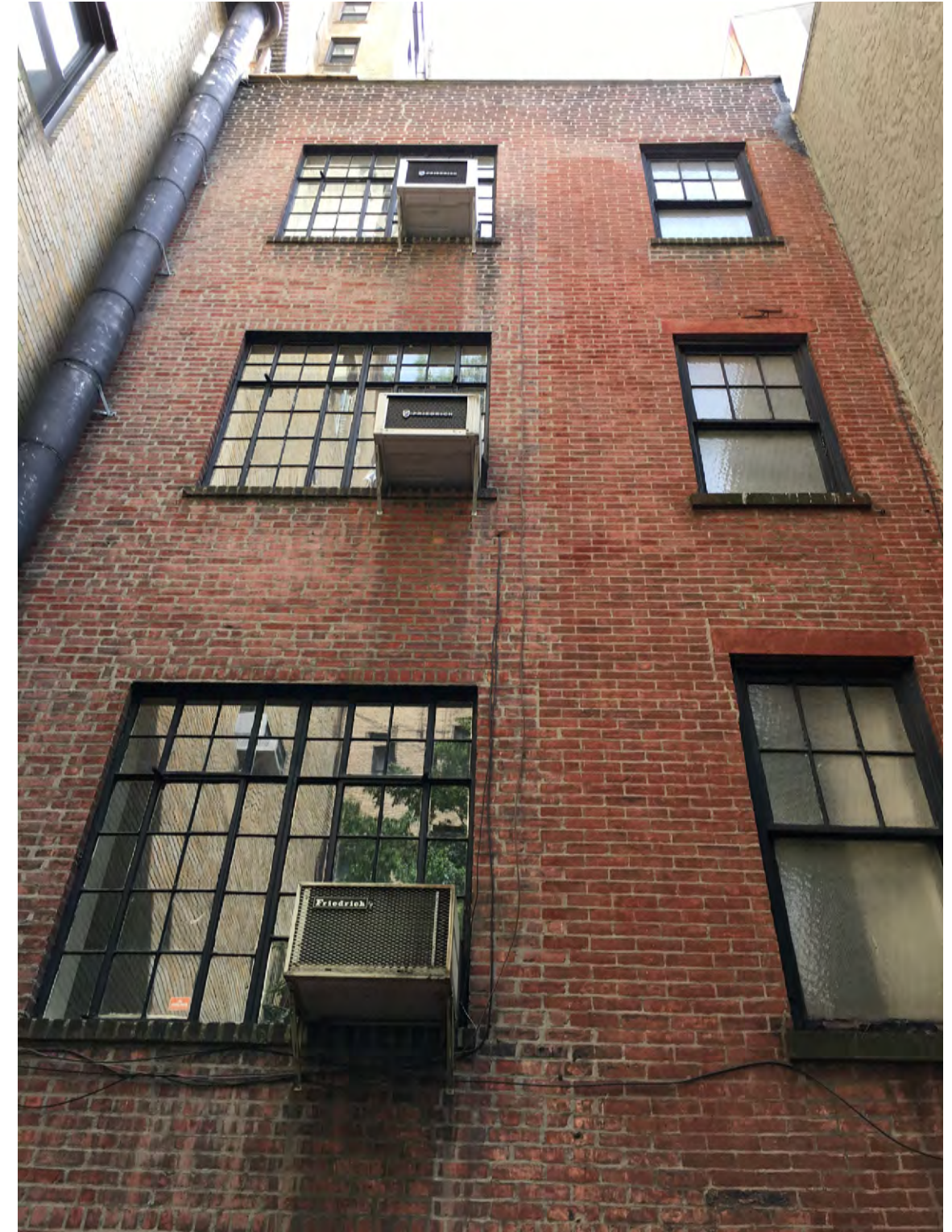
Existing Rear Facade - Third, Fourth, and Fifth Floors
