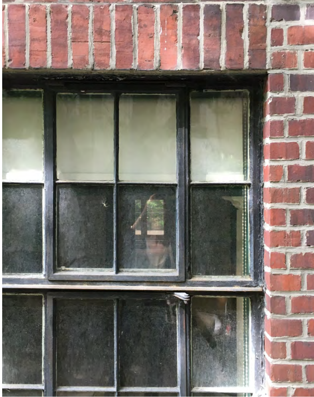
Existing Front Windows - Exterior
