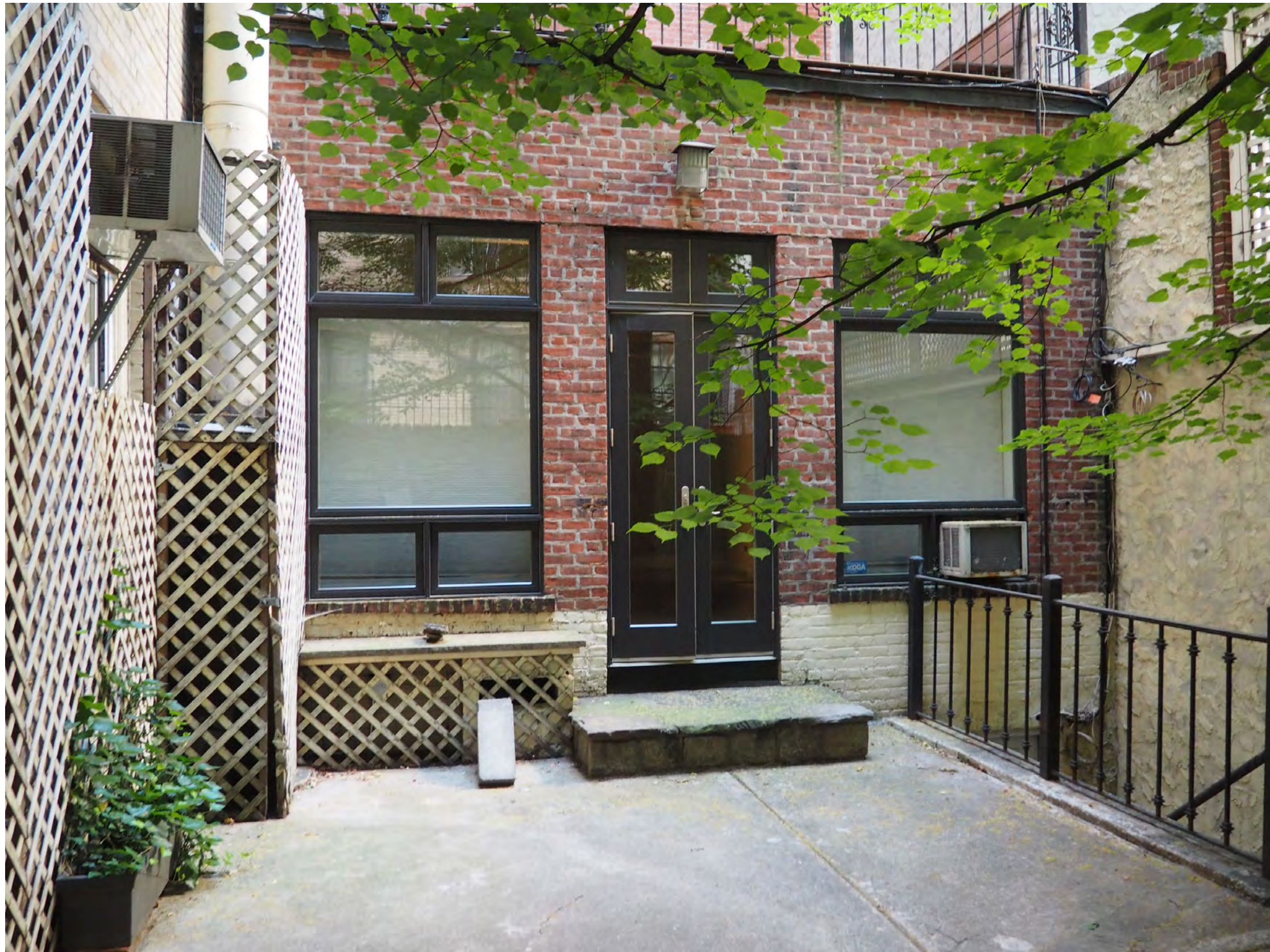
Existing Rear Ground Floor
