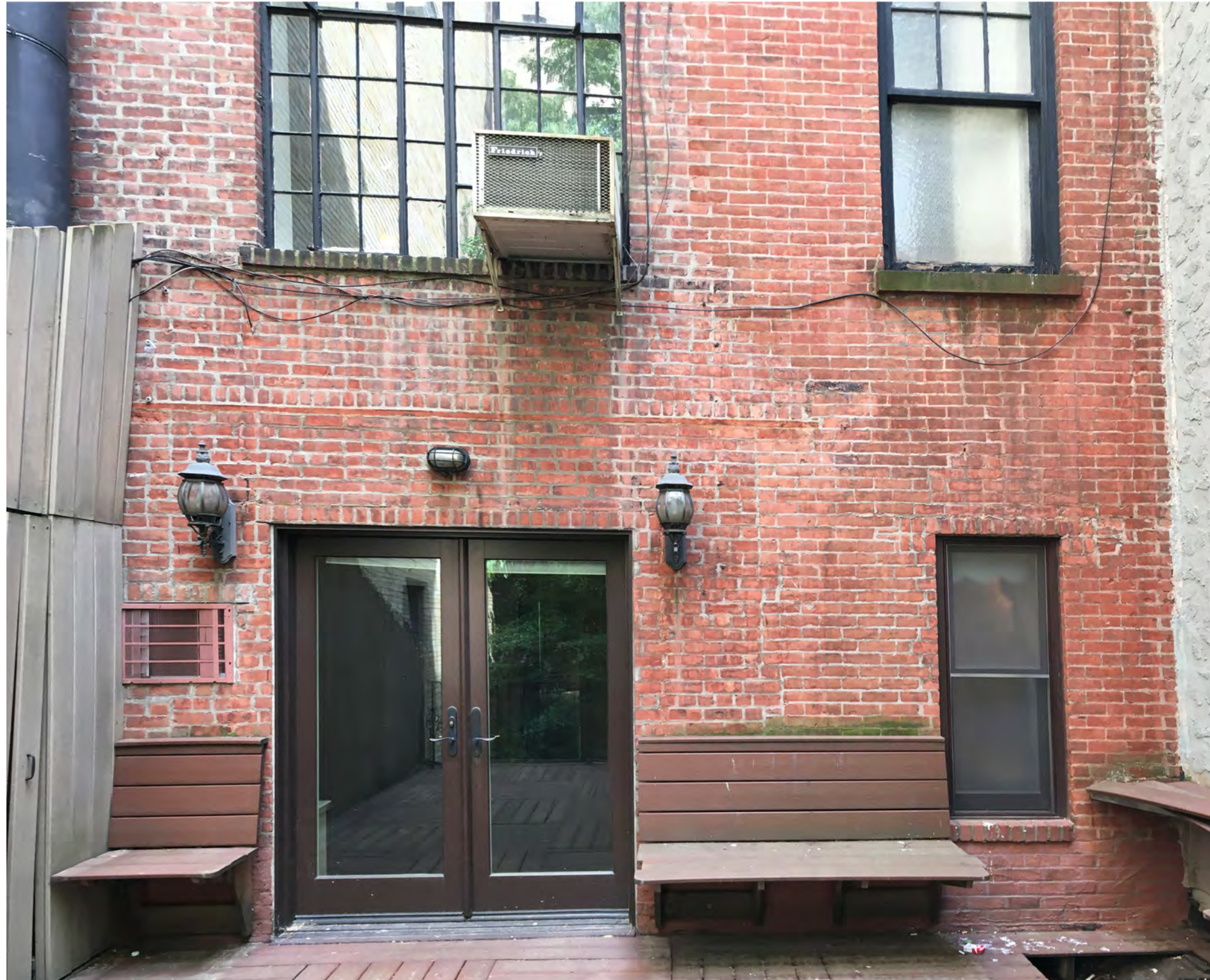
Existing Rear Terrace - Second Floor
