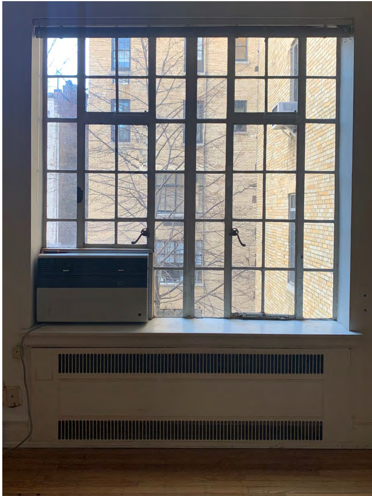
Existing Rear Windows - Interior
