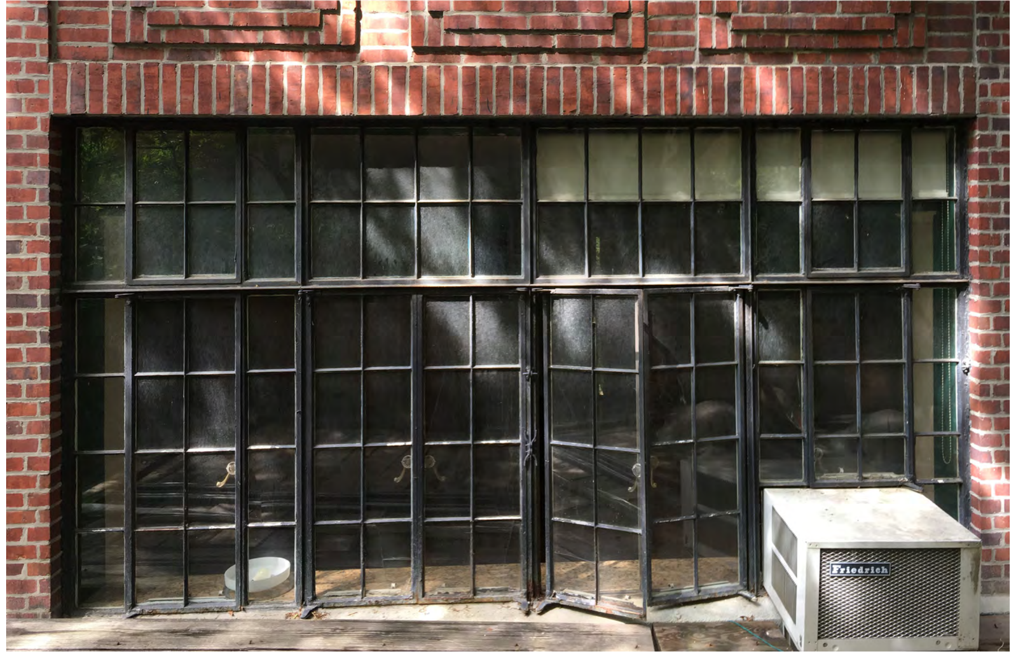
Existing Front Windows - Exterior
