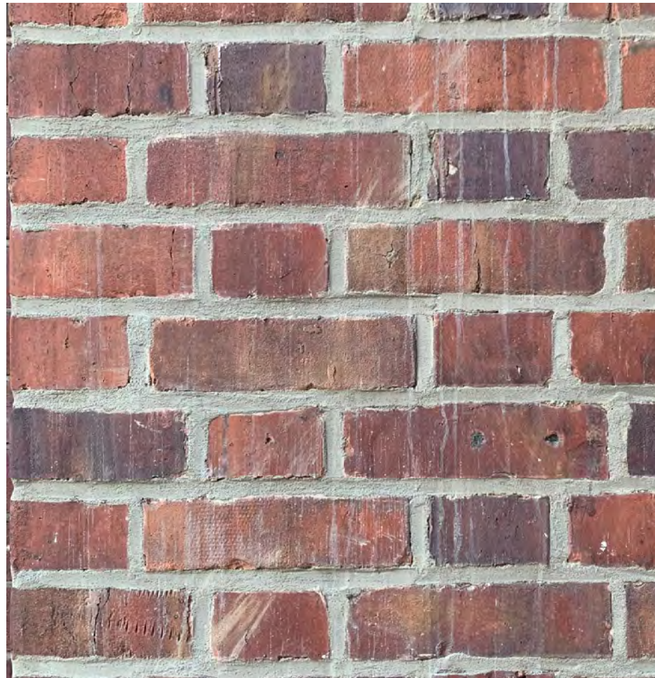
Existing Street Facade Masonry
