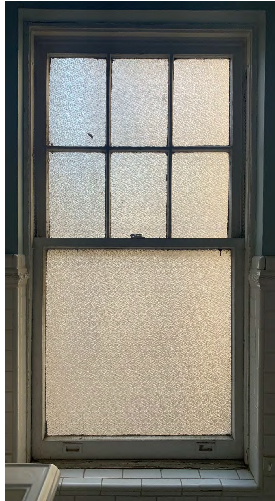
Existing Rear Windows - Interior
