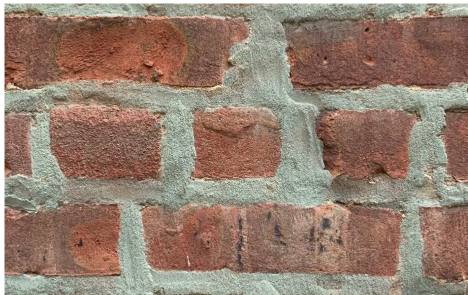
Existing Rear Facade Masonry
