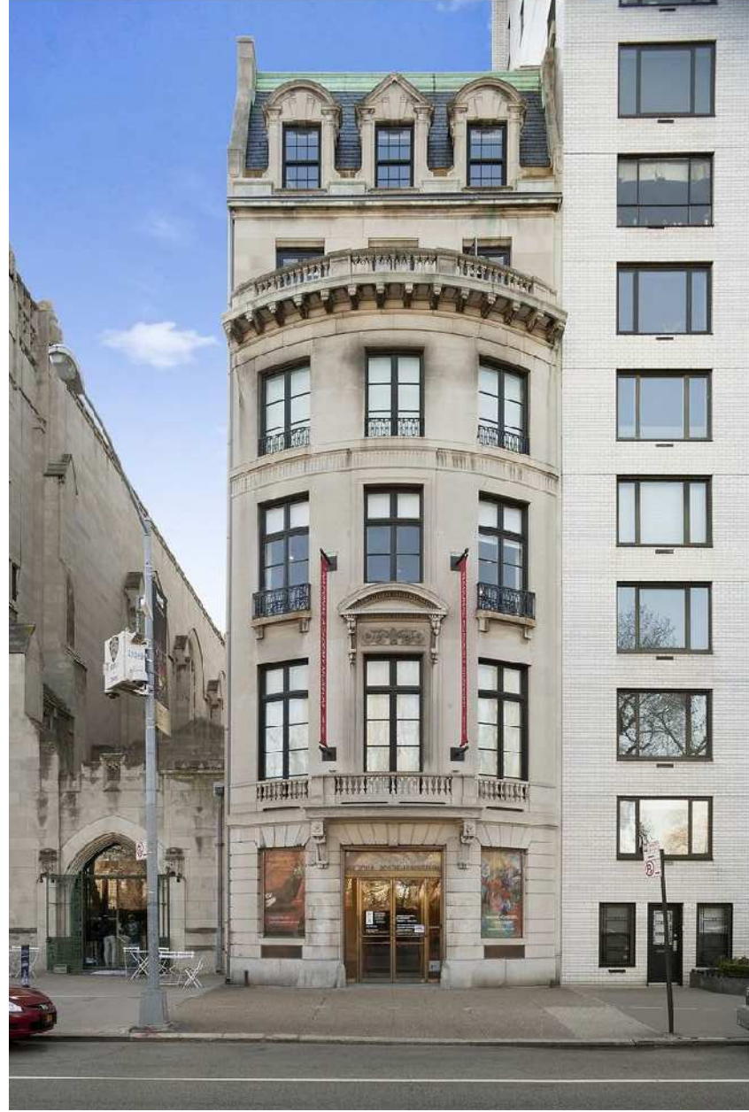
B EXISTING VIEW B EXISTING STAIR/ELEVATOR BULKHEAD NOT VISIBLE
