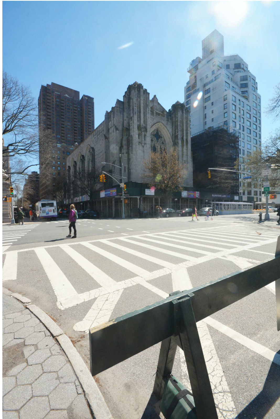
2 VIEW FROM NORTH SIDE OF ENGINEER'S GATE MOCK-UP IS NOT VISIBLE
