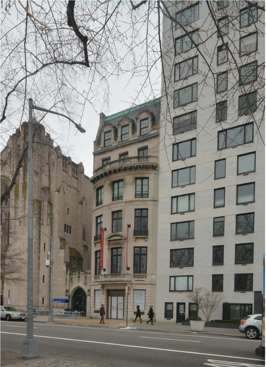
C EXISTING VIEW C EXISTING STAIR/ ELEVATOR BULKHEAD NOT VISIBLE
