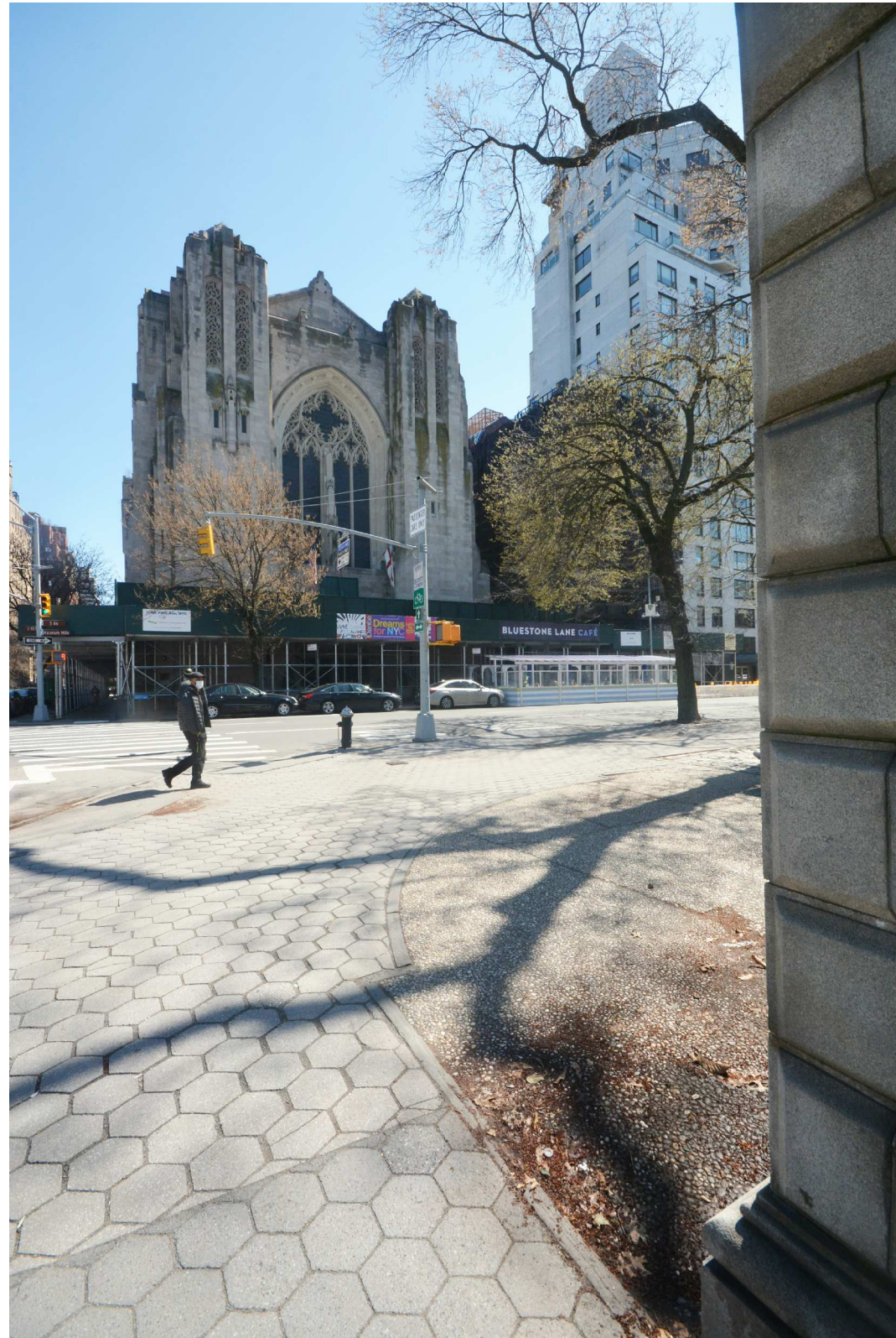
3 VIEW FROM SOUTH SIDE OF ENGINEER'S GATE MOCK-UP IS PARTIALLY VISIBLE OVER SECONDARY FACADE
