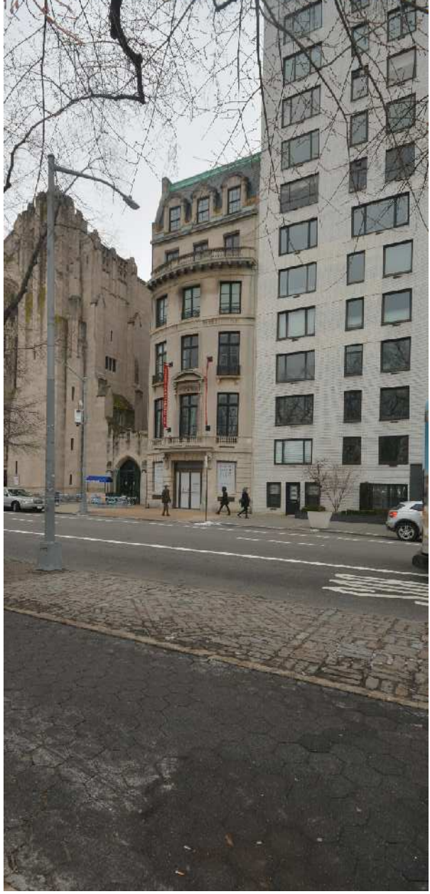
C VIEW C EXISTING STAIR/ ELEVATOR ROOF BULKHEAD NOT VISIBLE
