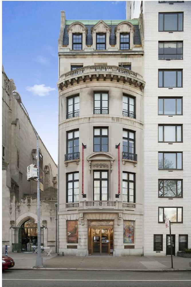
Current View of Existing Facade
