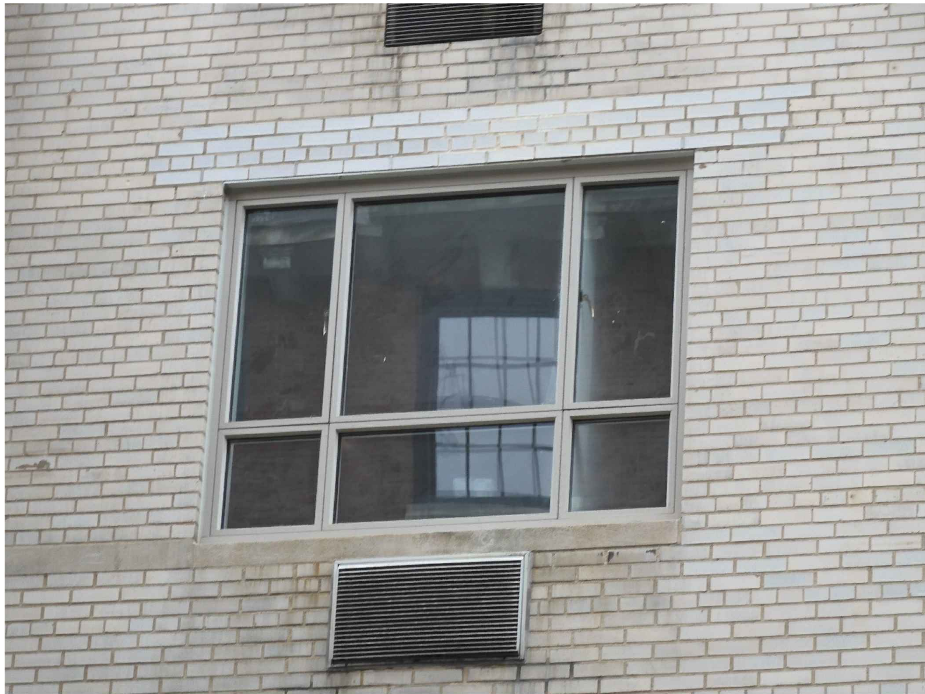
WEST WINDOW SHOWING NO VISIBILITY OF WALL MOCKUP
