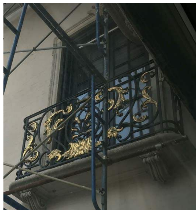
NEW WROUGHT IRON RAILING AND CAST LIMESTONE BALCONY TO MATCH ADJACENT BALCONIES ON FLOOR ABOVE
