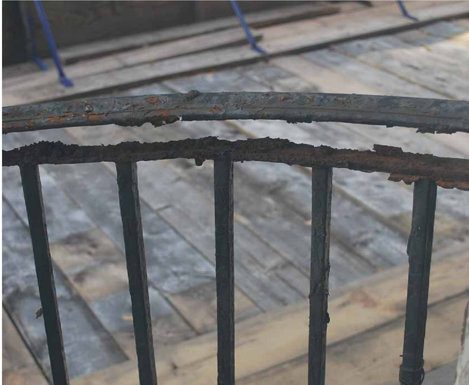
EXISTING WROUGH IRON CONDITION
