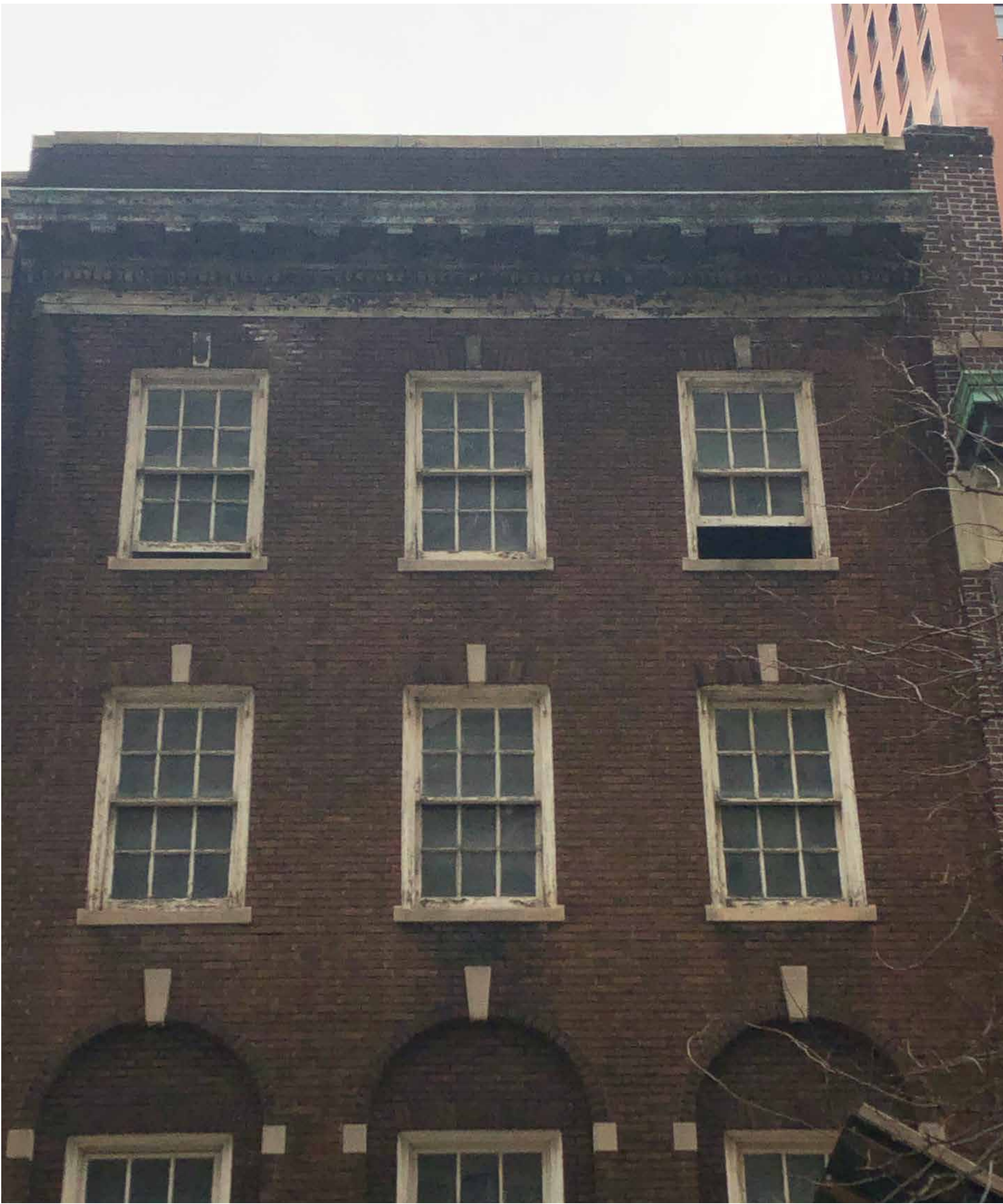
DETERIORATION OF CORNICE AND DOUBLE HUNG WINDOWS
