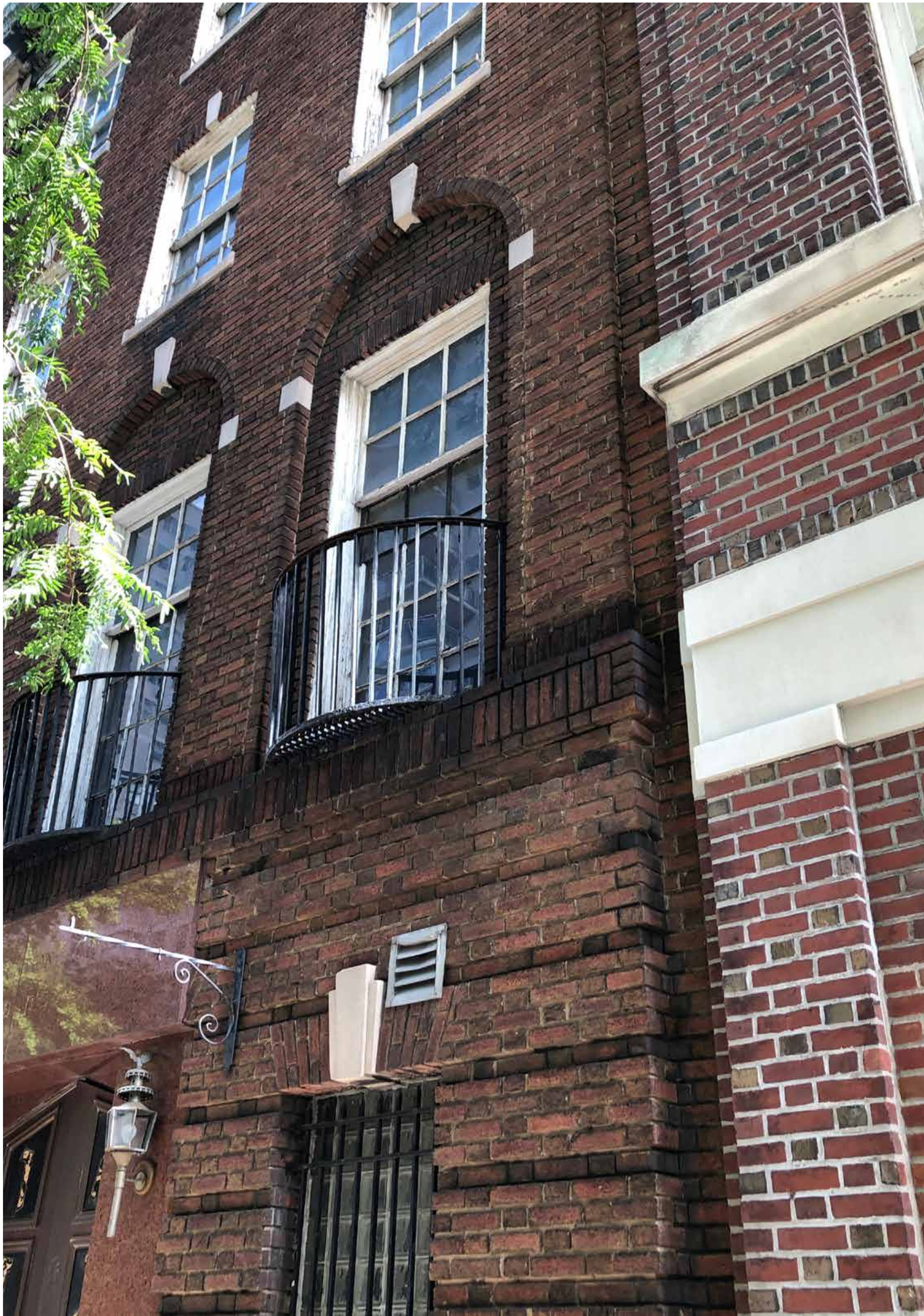
EXISTING CONDITIONS OF 163 EAST 69TH STREET BRICK WORK DETAIL AND WROUGHT IRON RAILING
