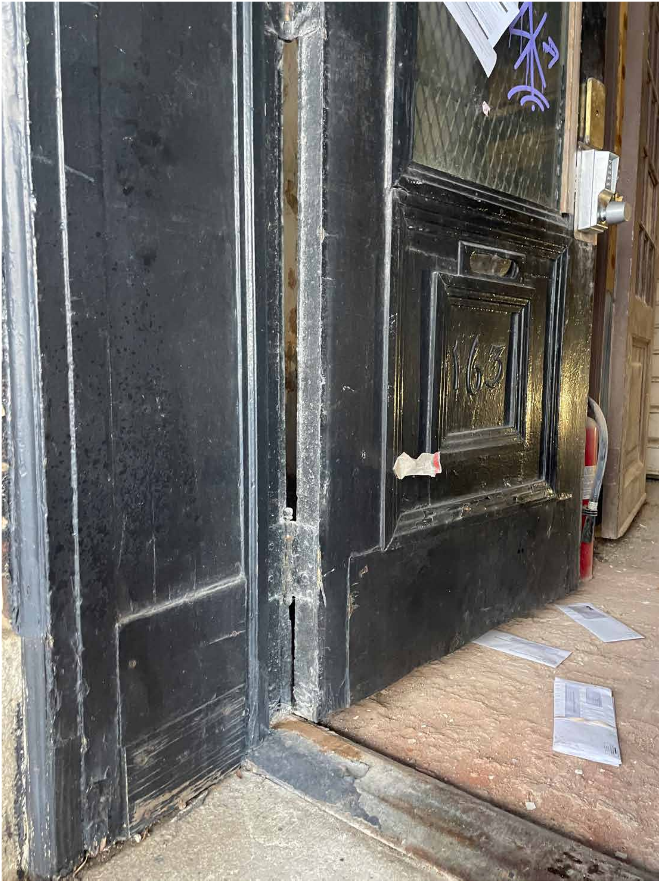
EXISTING CONDITIONS OF MAIN ENTRY WOOD DOOR.
