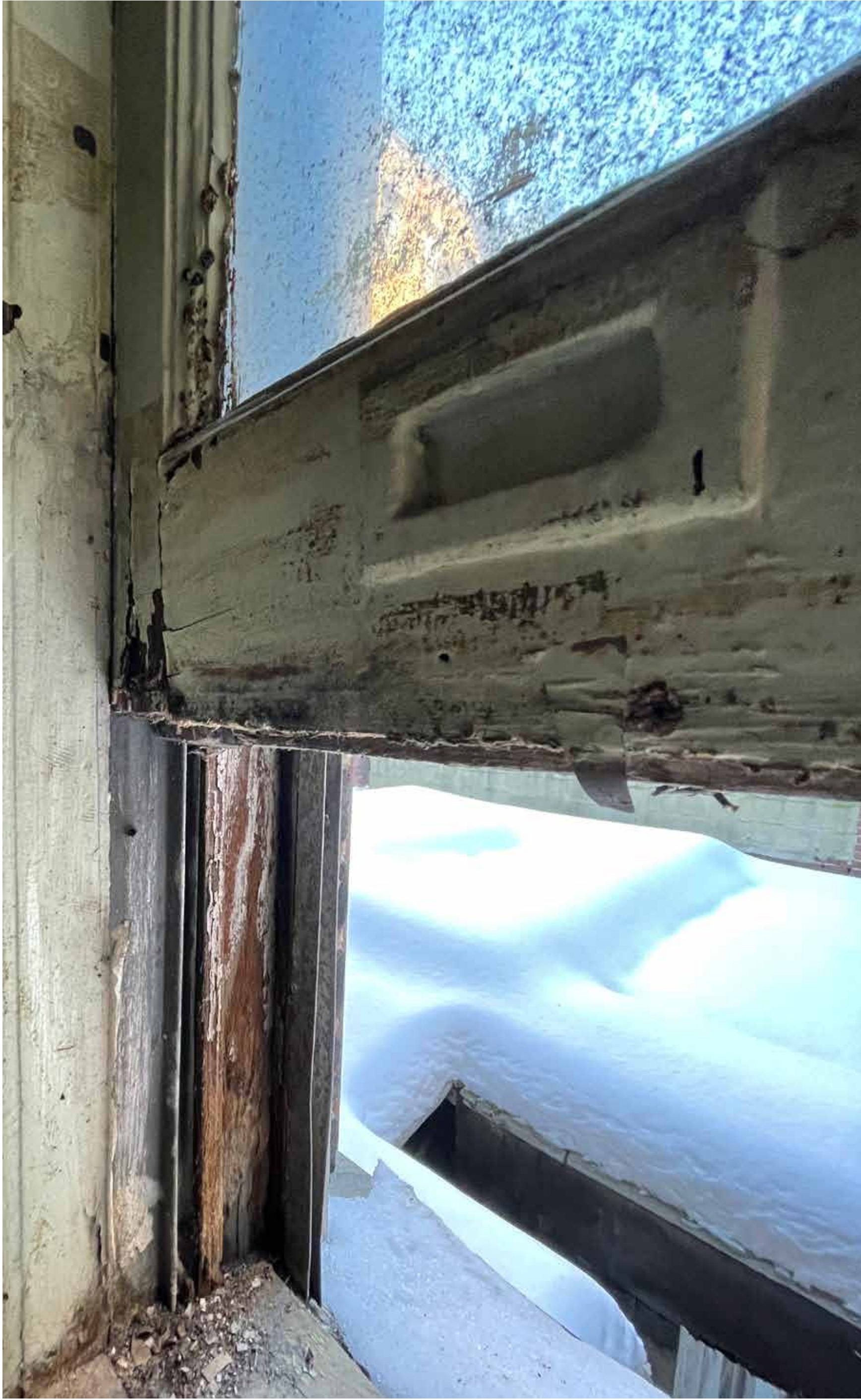
EXISTING TYPICAL CONDITIONS OF STREET FRONTING WINDOWS.
