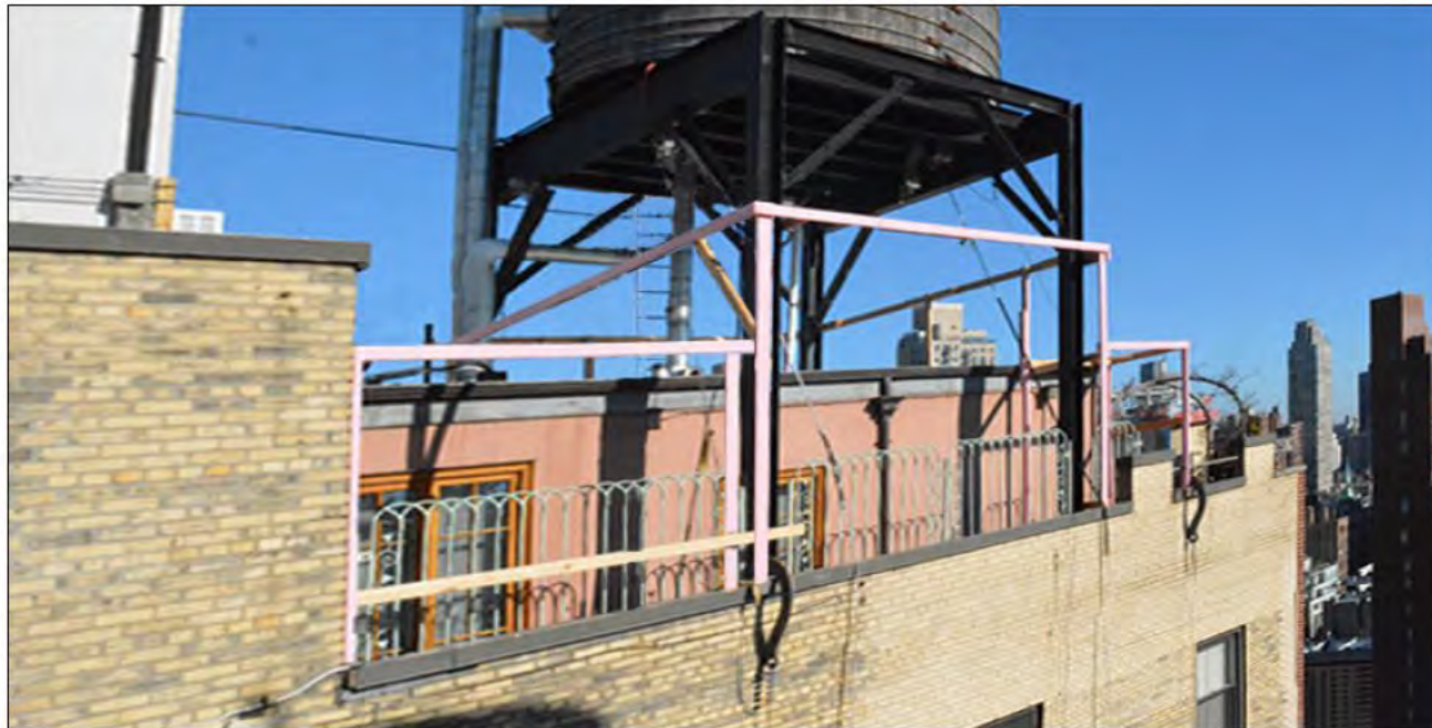
Existing view of penthouse and mock-up from the South East
