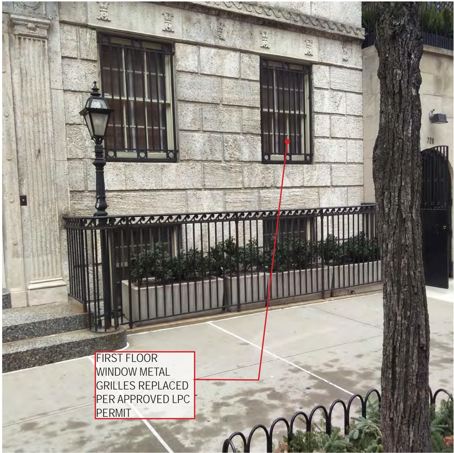
FIRST FLOOR WINDOWS CURRENT CONDITION
