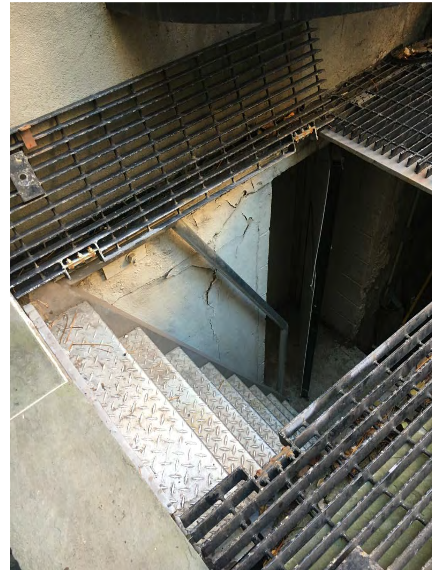
EXISTING METAL HATCH AND STAIR
