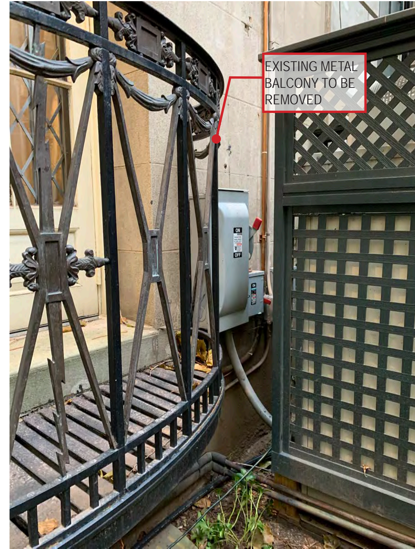
EXISTING HVAC CONTROL PANELS
