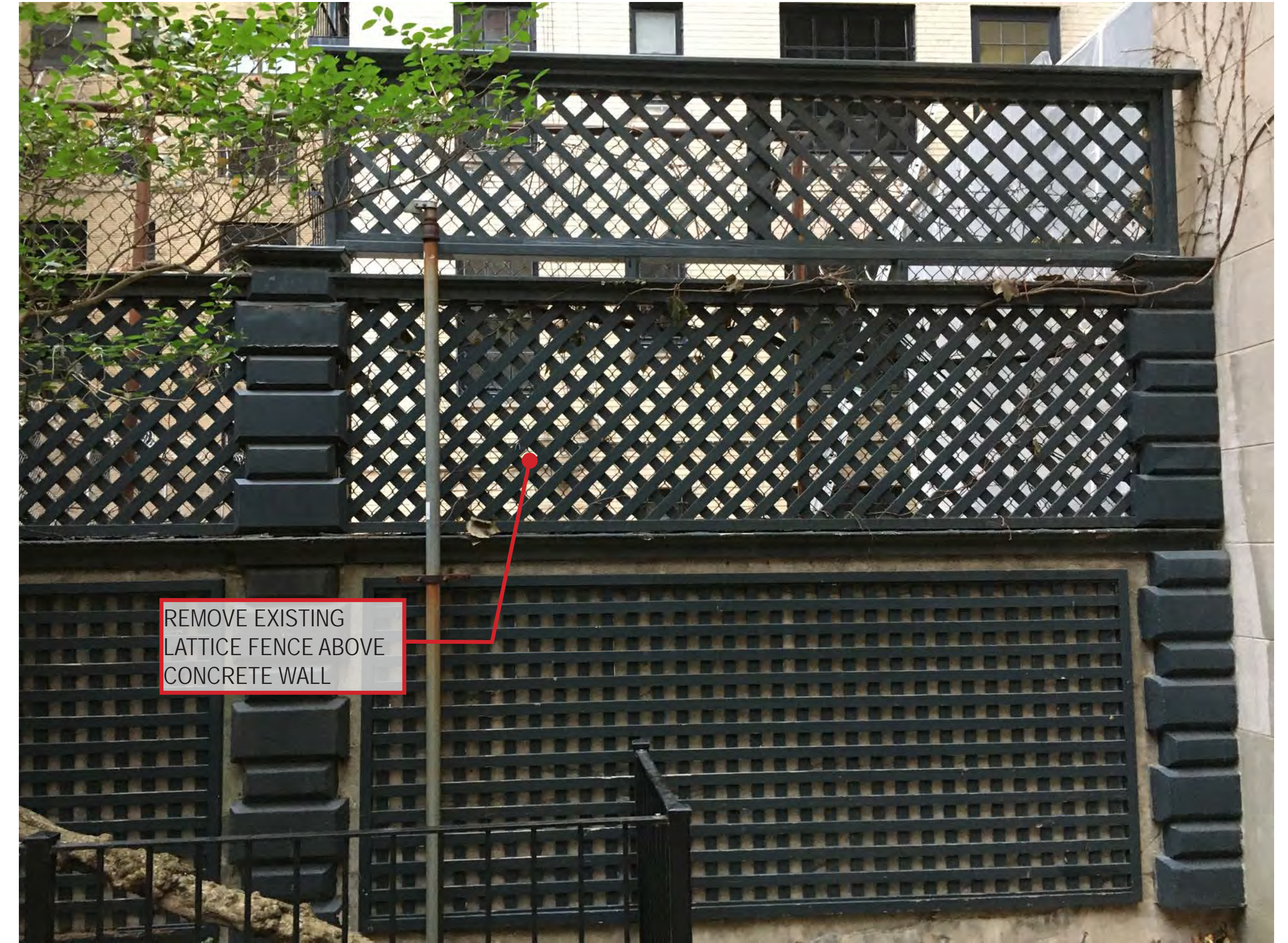
EXISTING REAR YARD WEST LATTICE FENCE CLOSE-UP
