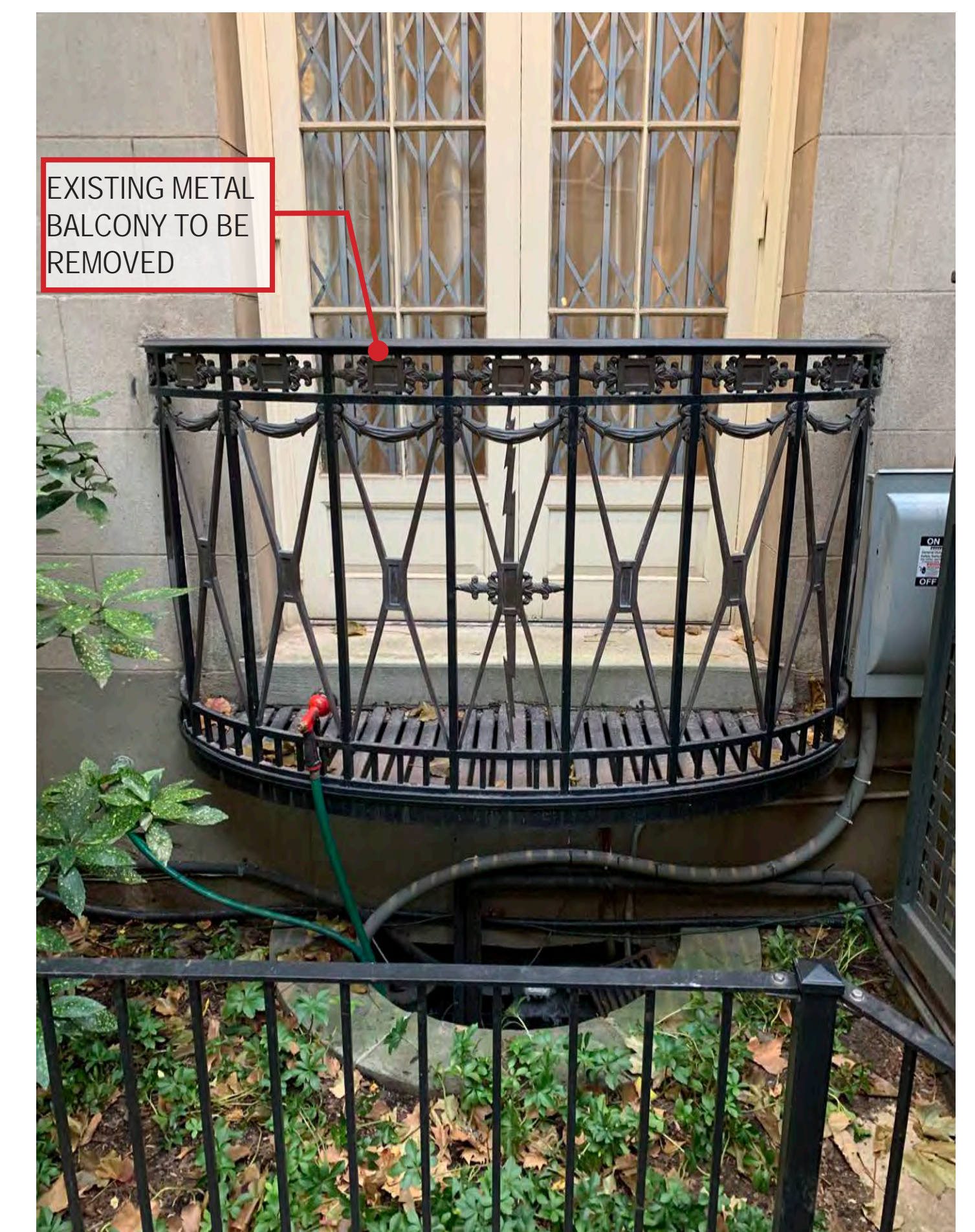
EXISTING TYPICAL METAL BALCONY
