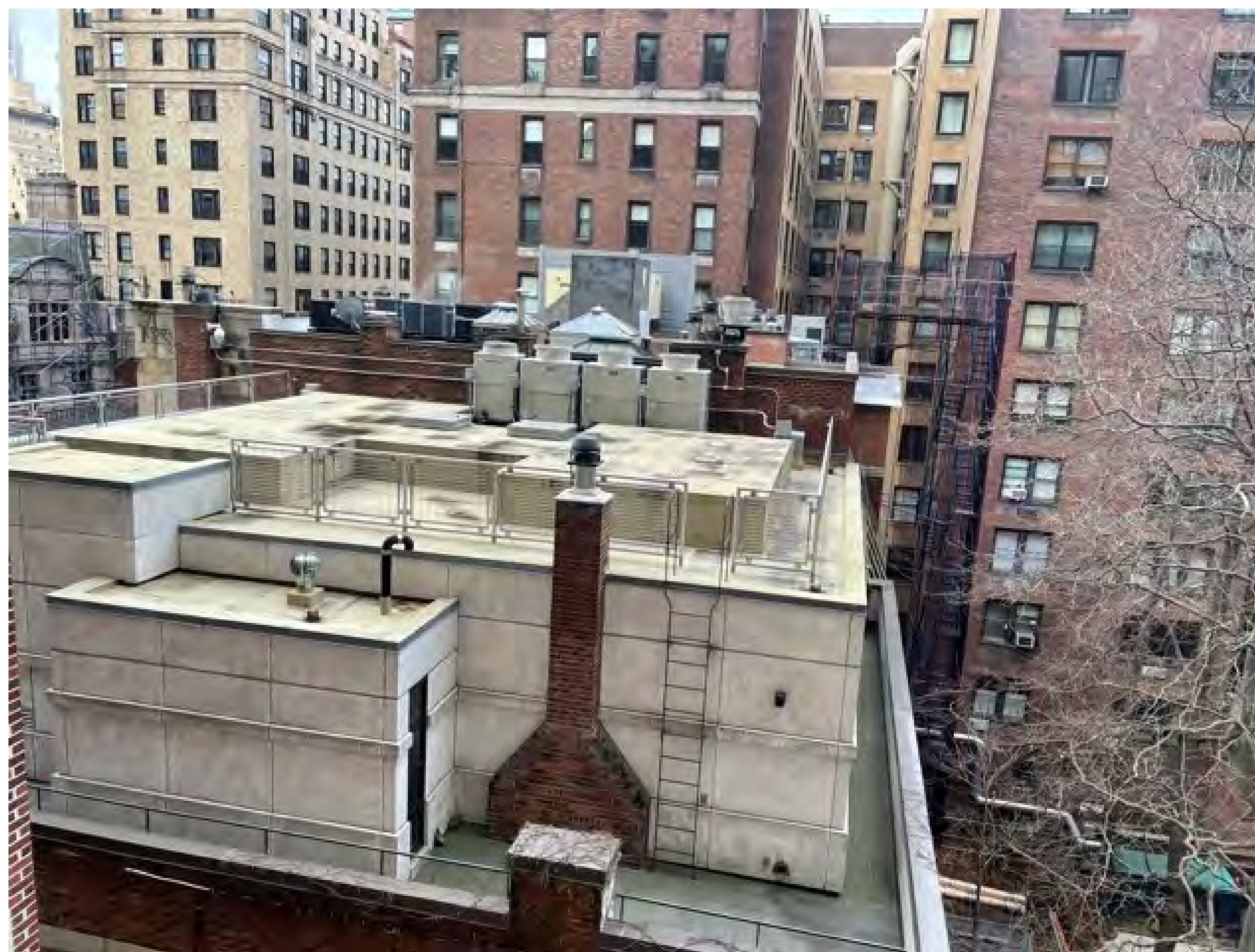
PENTHOUSE ROOF ADDITION CLOSE-UP
