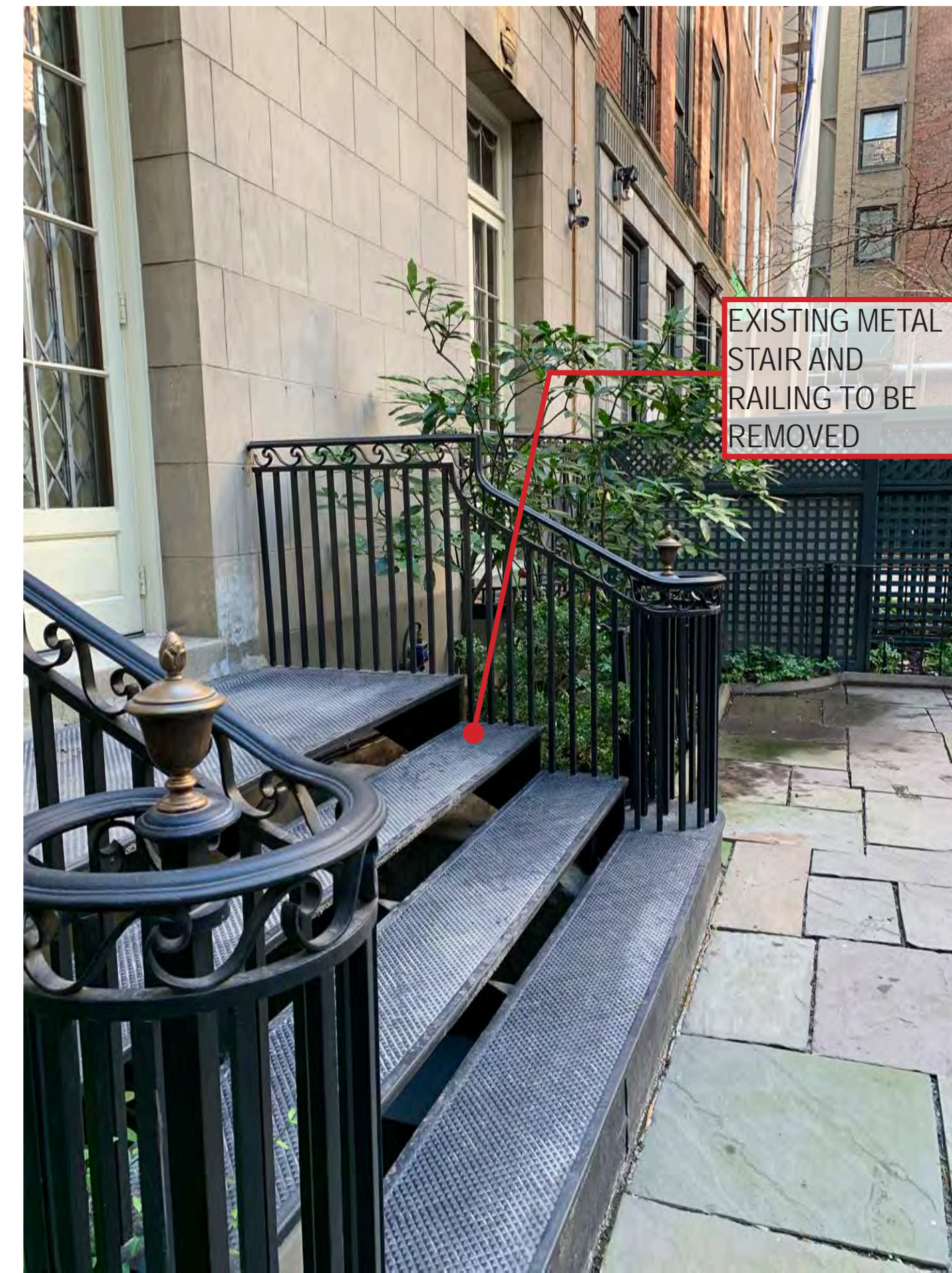
EXISTING METAL STAIR AND RAILING
