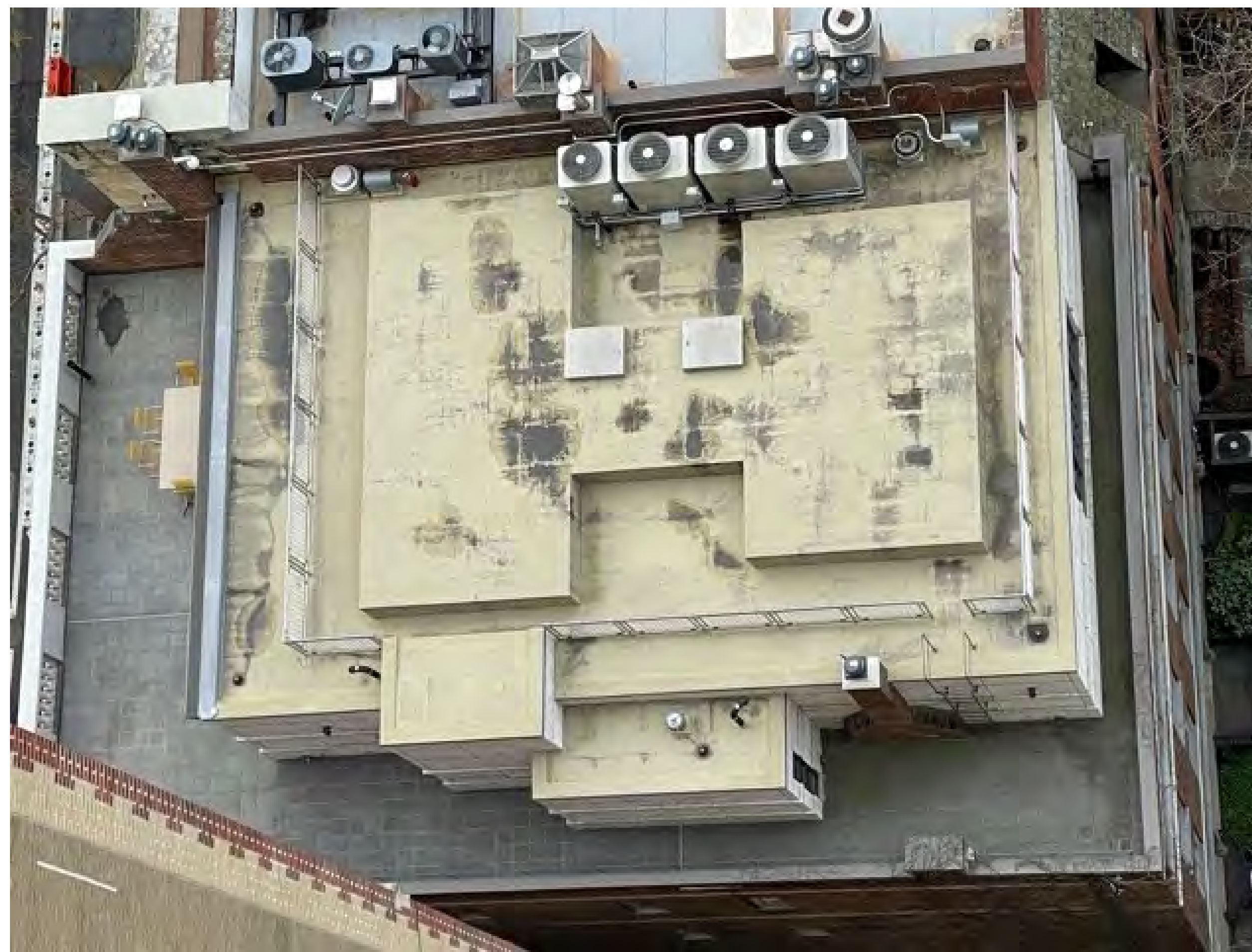
BIRDSEYE VIEW OF PENTHOUSE ROOF ADDITION
