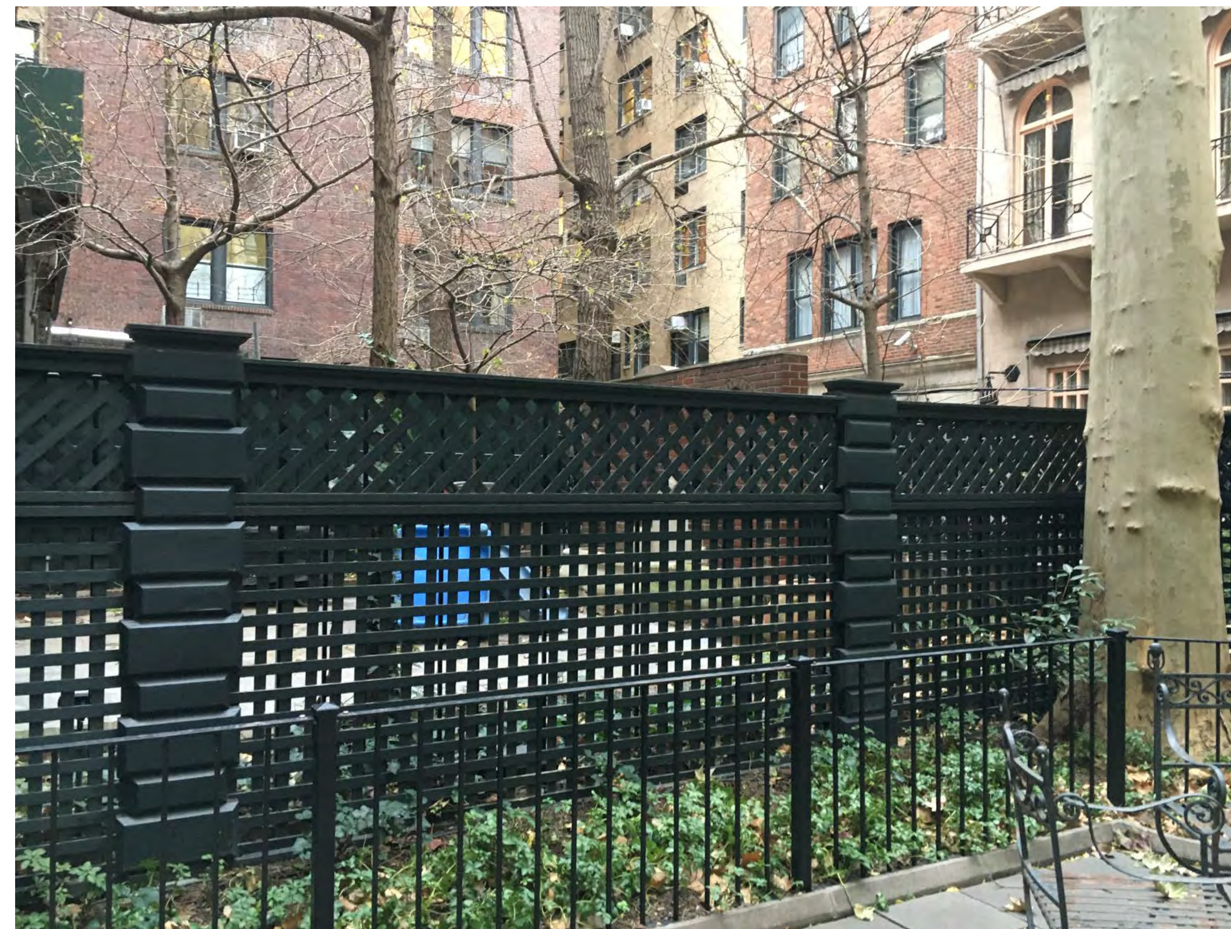
EXISTING REAR YARD NORTHWEST FENCE CLOSE-UP
