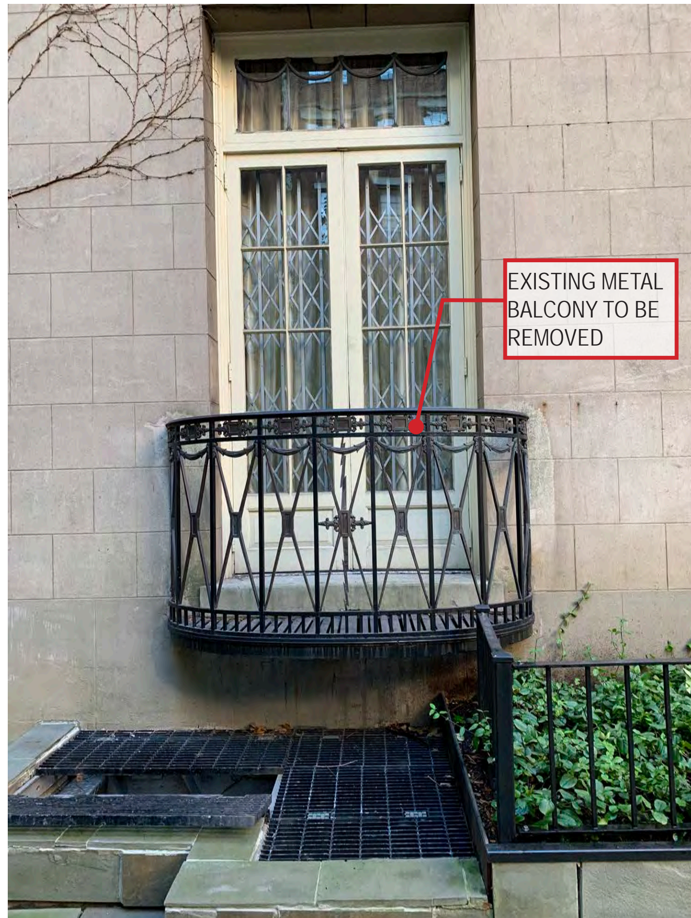
EXISTING METAL GRATE AND HATCH
