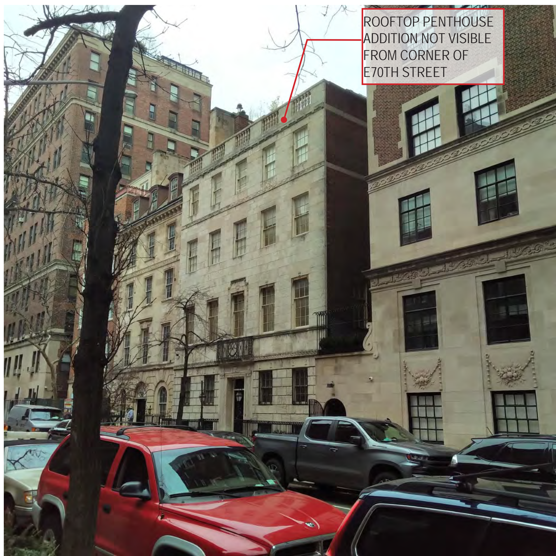
FRONT FACADE OF BUILDING FROM ACROSS THE STREET
