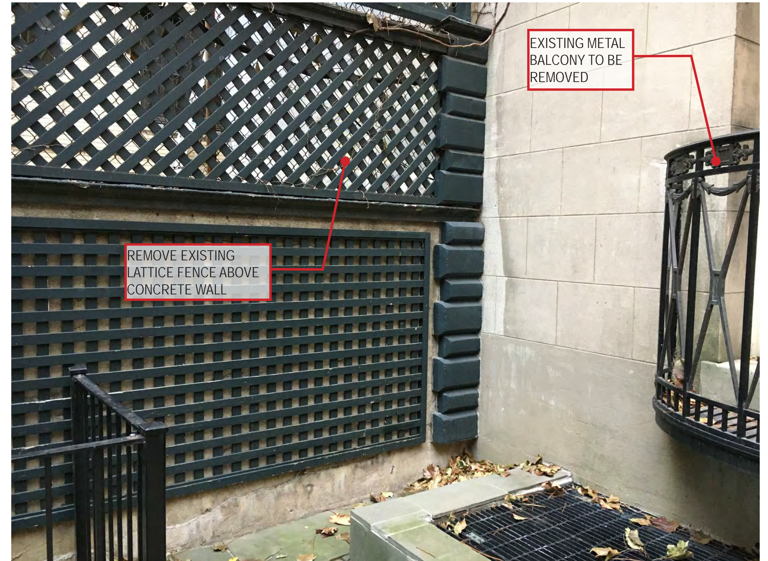
EXISTING REAR YARD SOUTHWEST WALL CLOSE-UP
