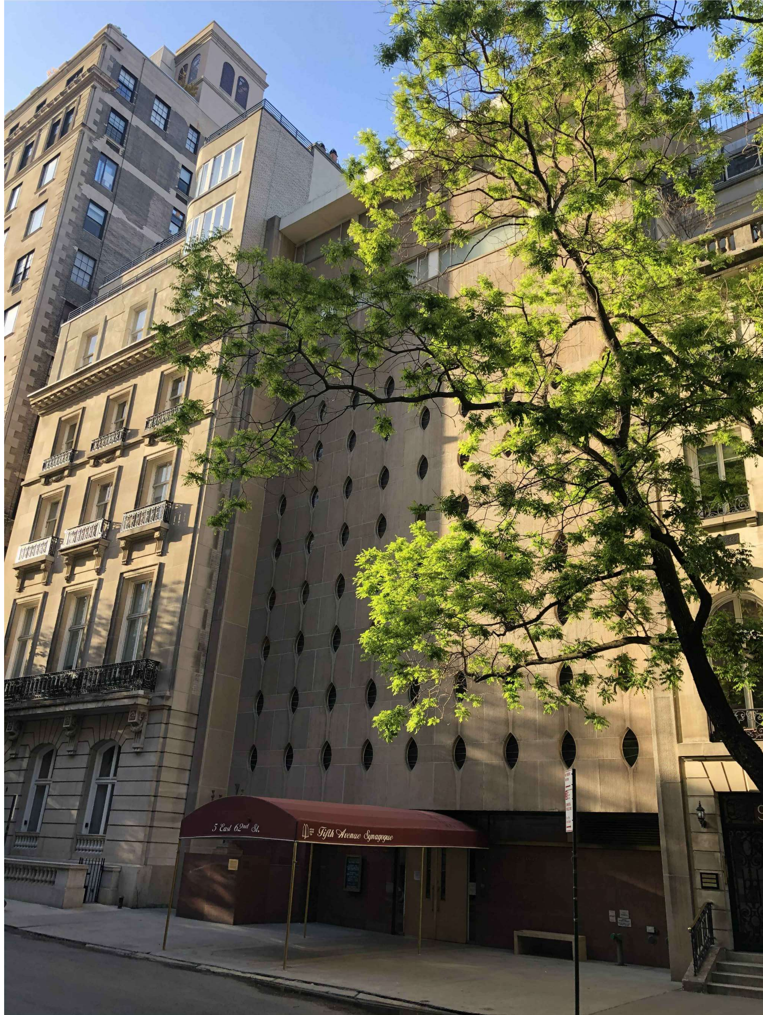
Existing Facade - North West View
