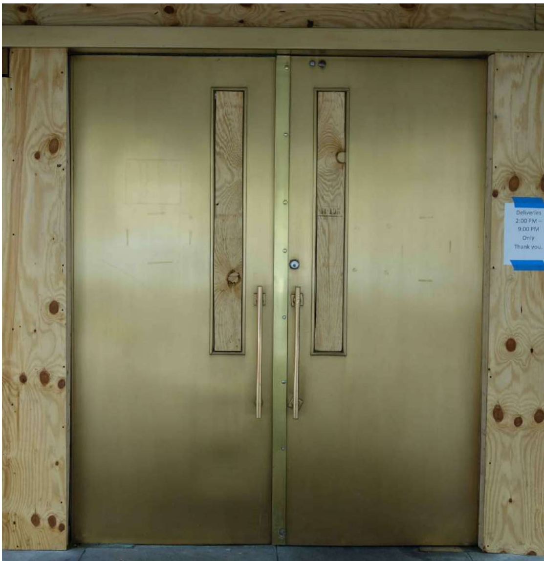
Existing Bronze Entry Door
