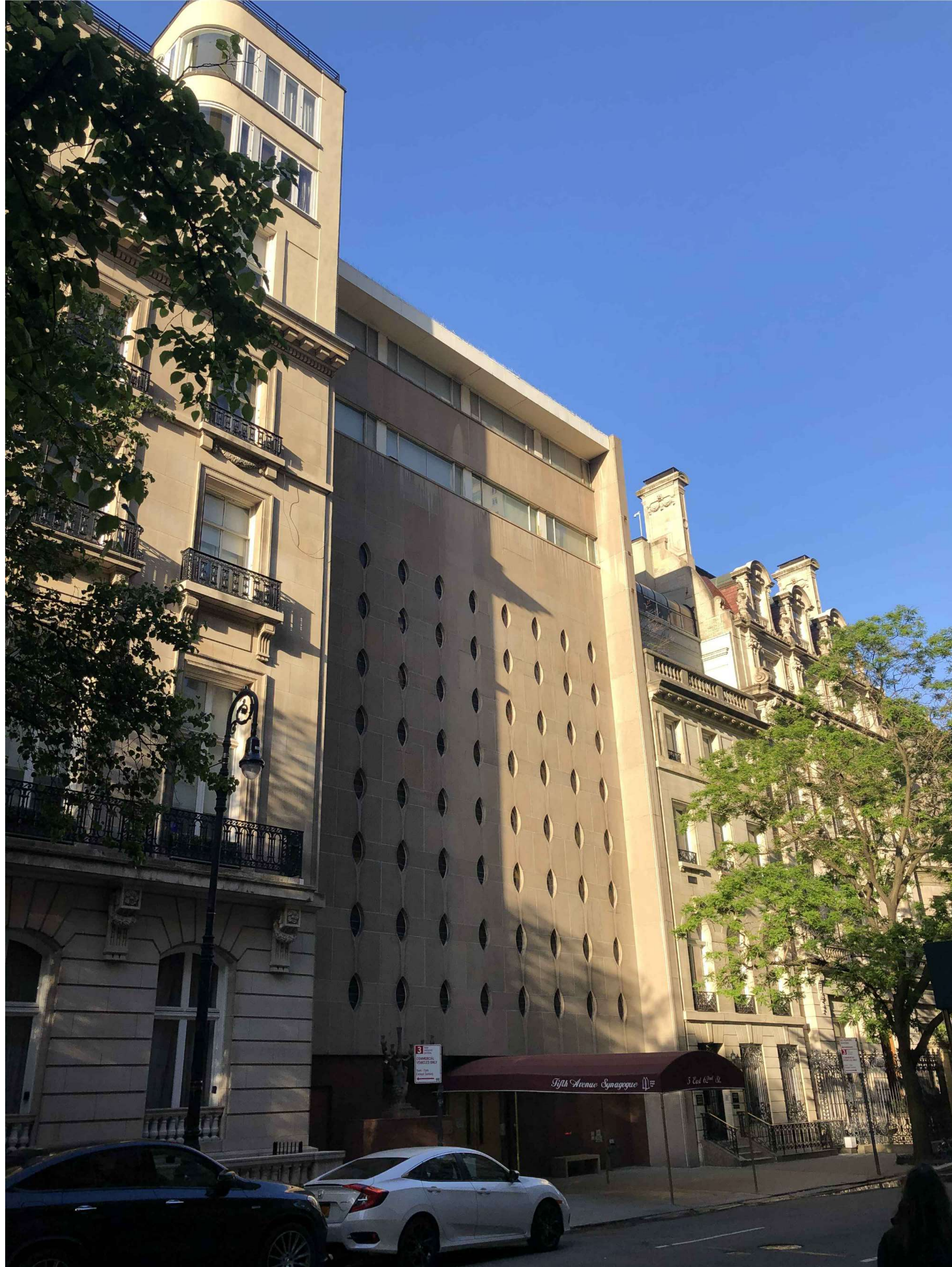
Existing Facade - North East View
