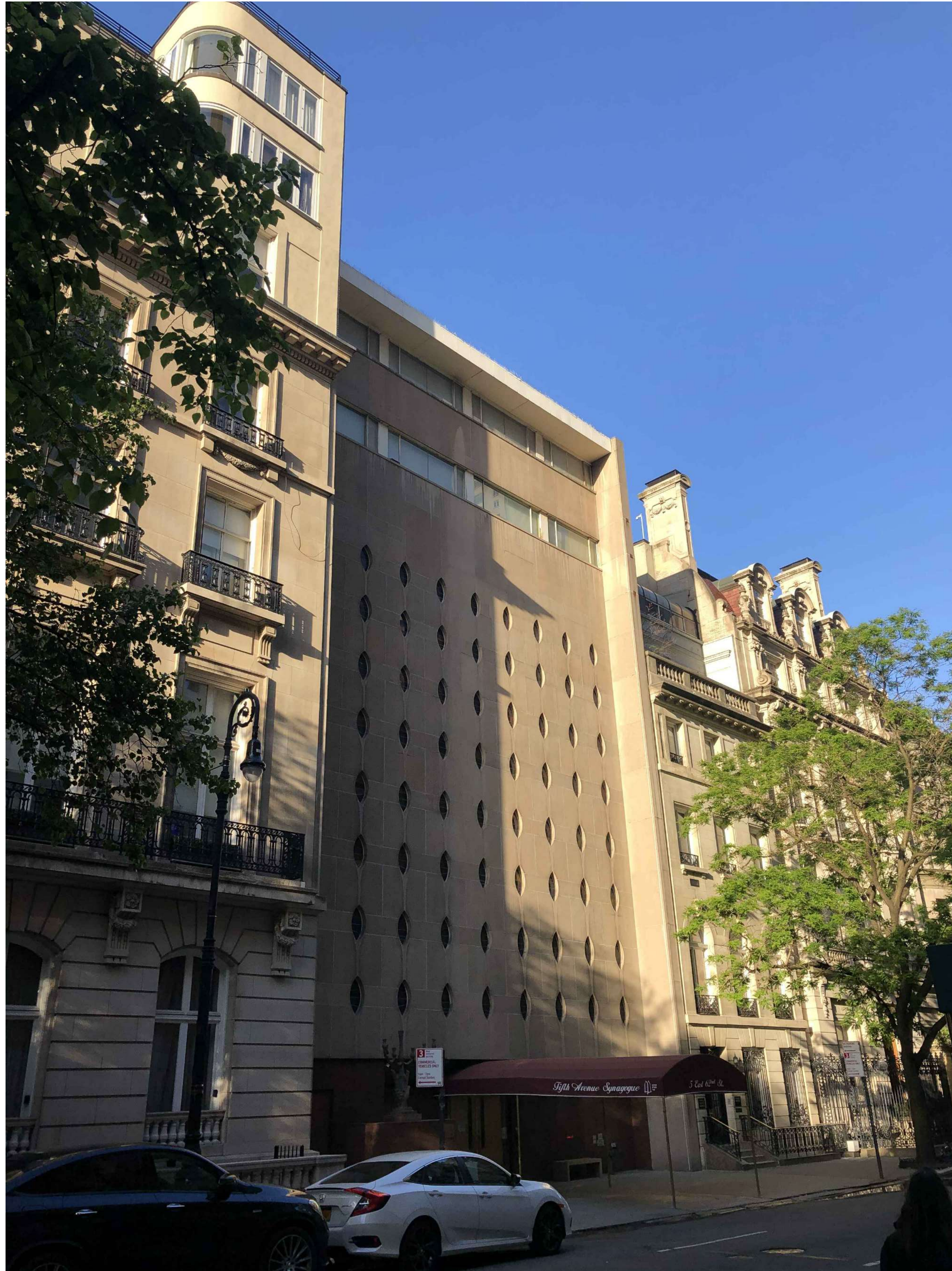
Existing Facade - North East View
