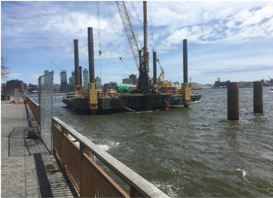
Barge mounted drill rig
