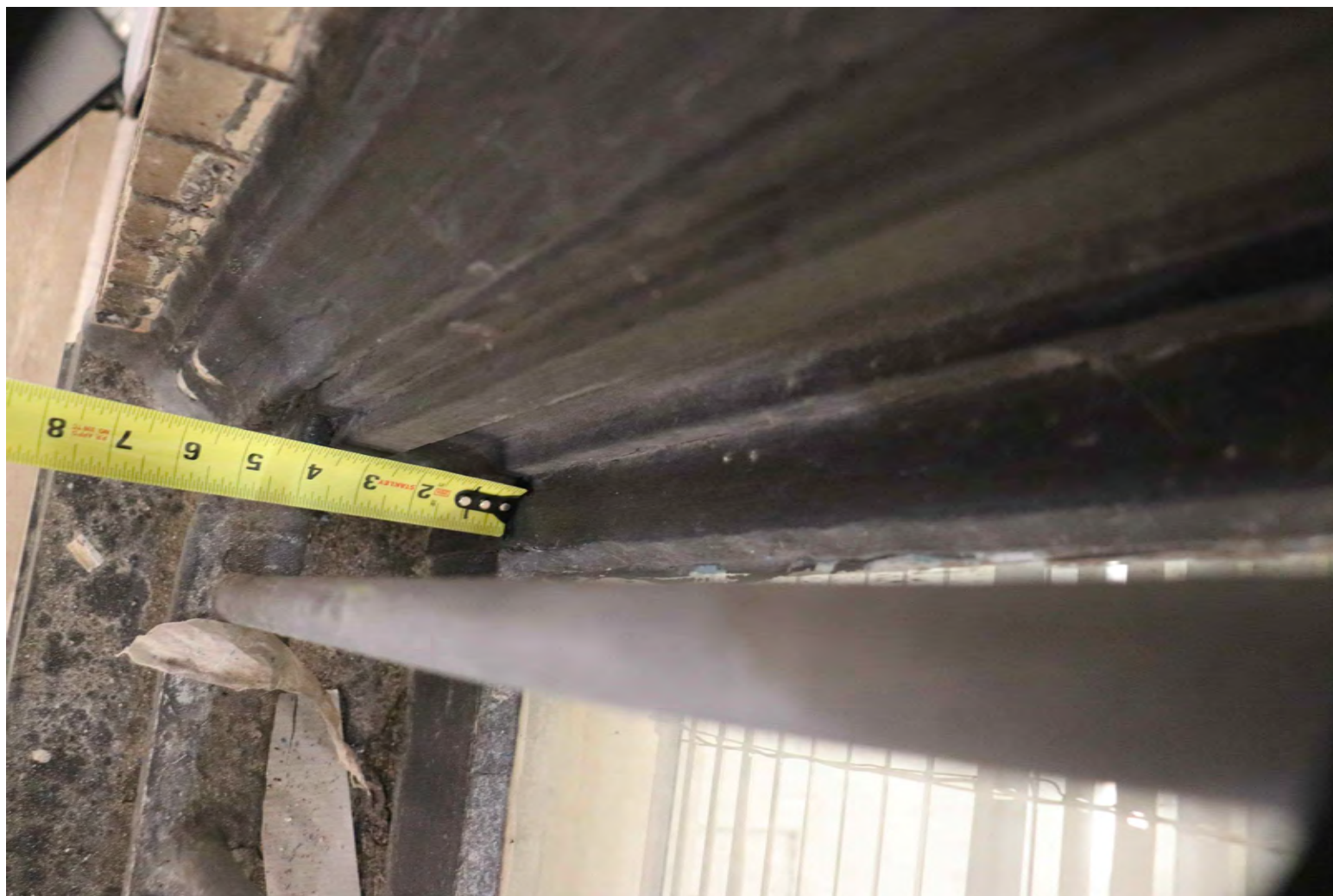
3 Existing / Original Wood Brickmould - Window Left Jamb
