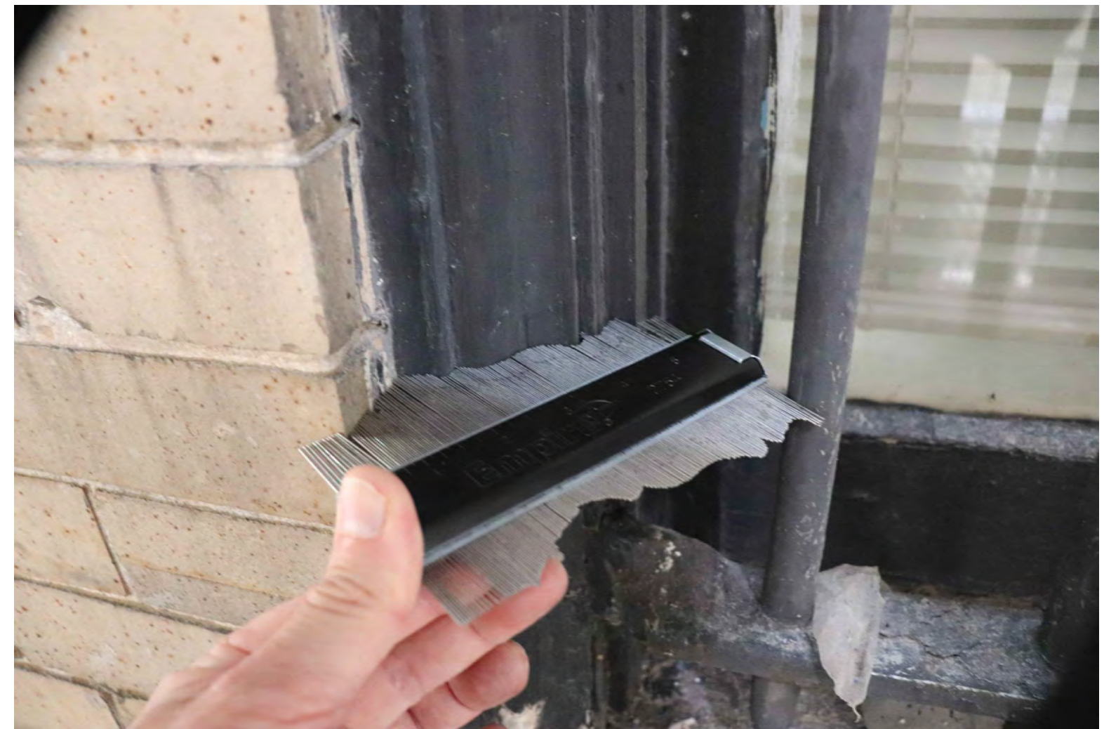
4 Existing / Original Wood Brickmould - Window Left Jamb
