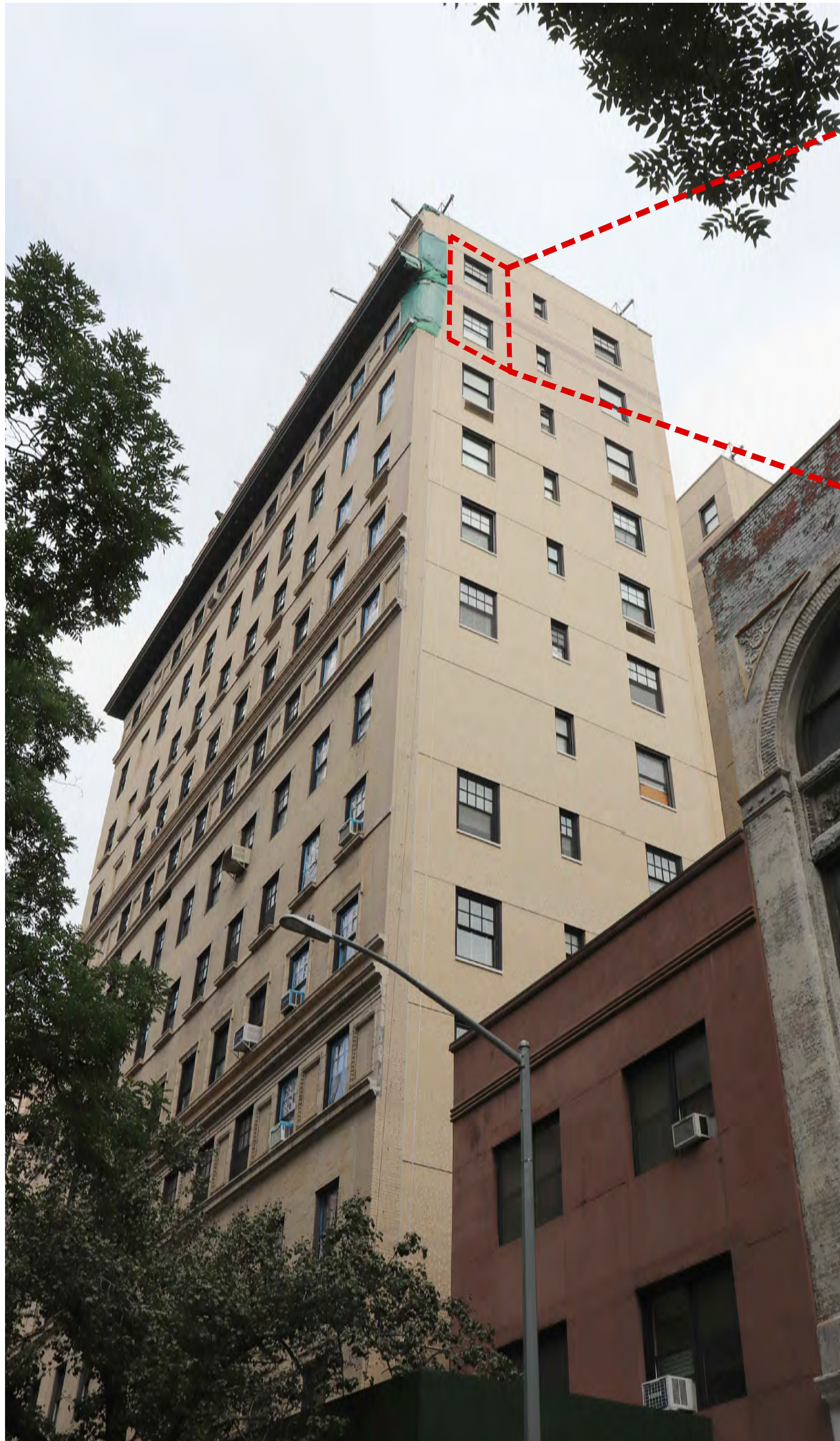
1 Existing Building Condition - Partial East Facade
