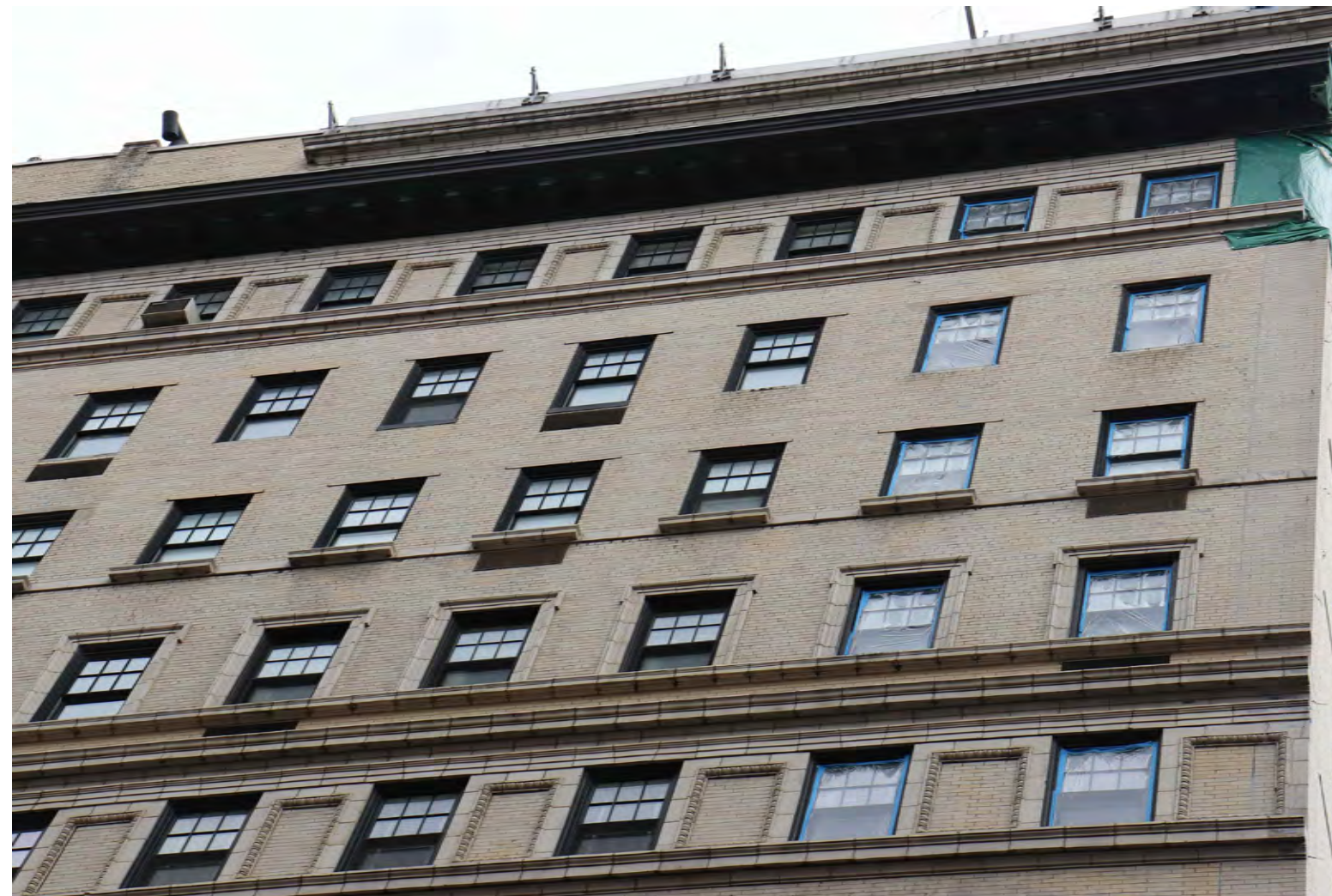
2 Close-up photo of the South / East Building Corner @ 82nd St., Top Floors
