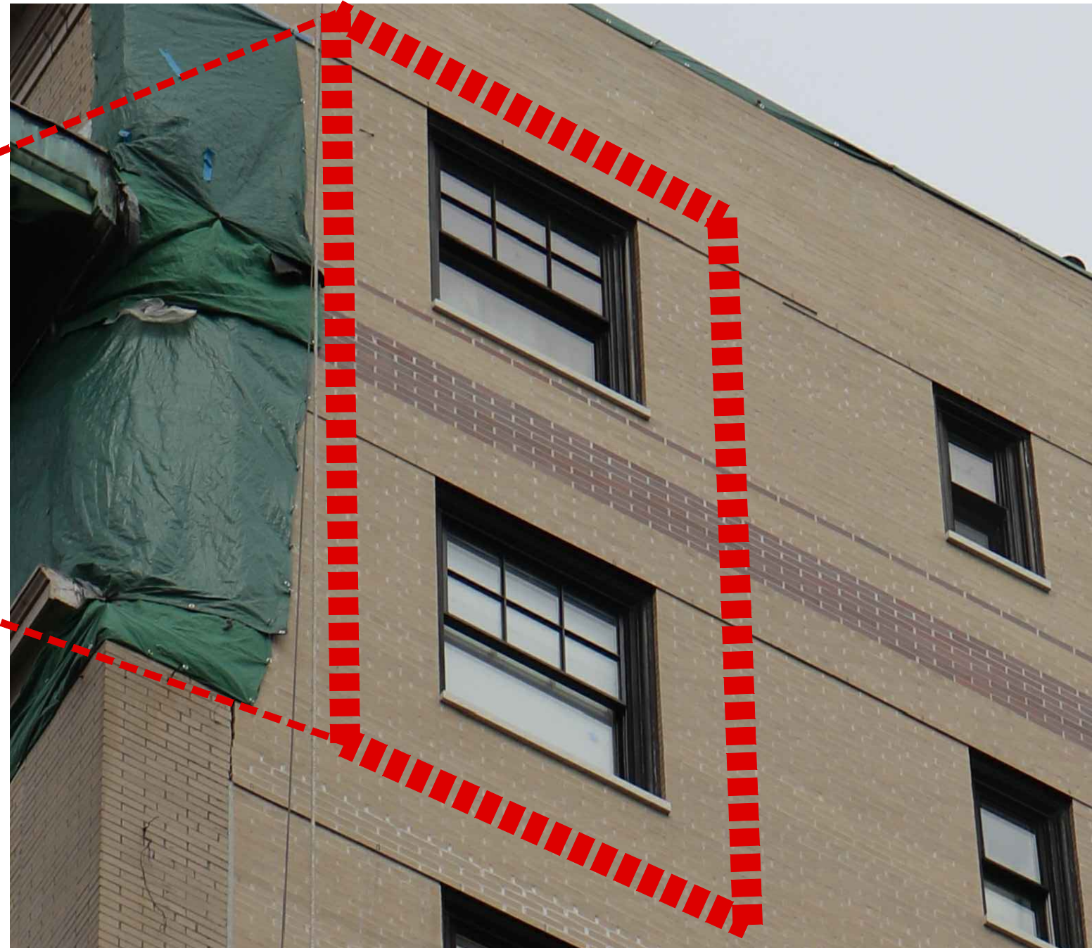
Existing 6 OVER 1 TYPICAL CONFIGURATION ACROSS THE ENTIRE BUILDING.
