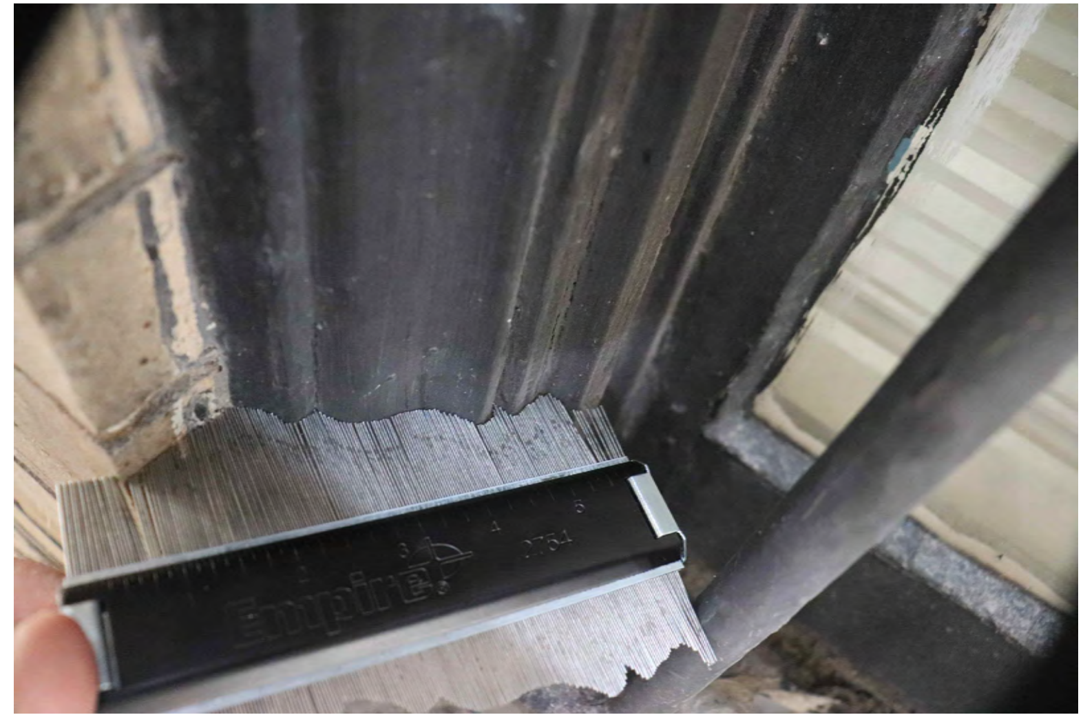
2 Existing / Original Wood Brickmould - Window Left Jamb / Sill
