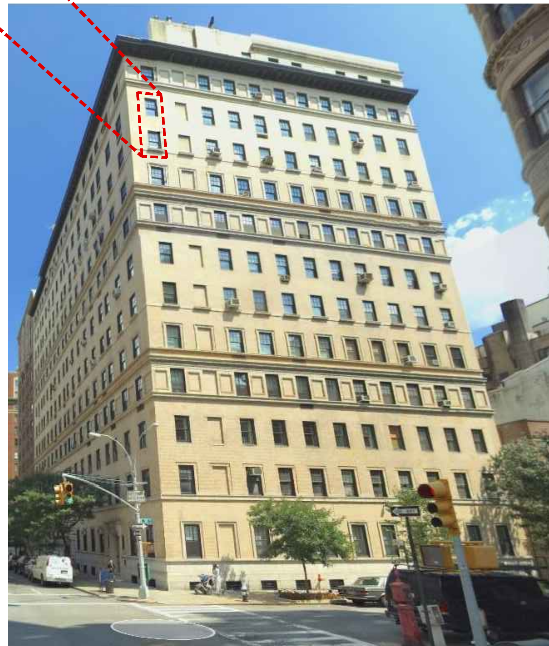
2 Existing Building Condition - South Facade
