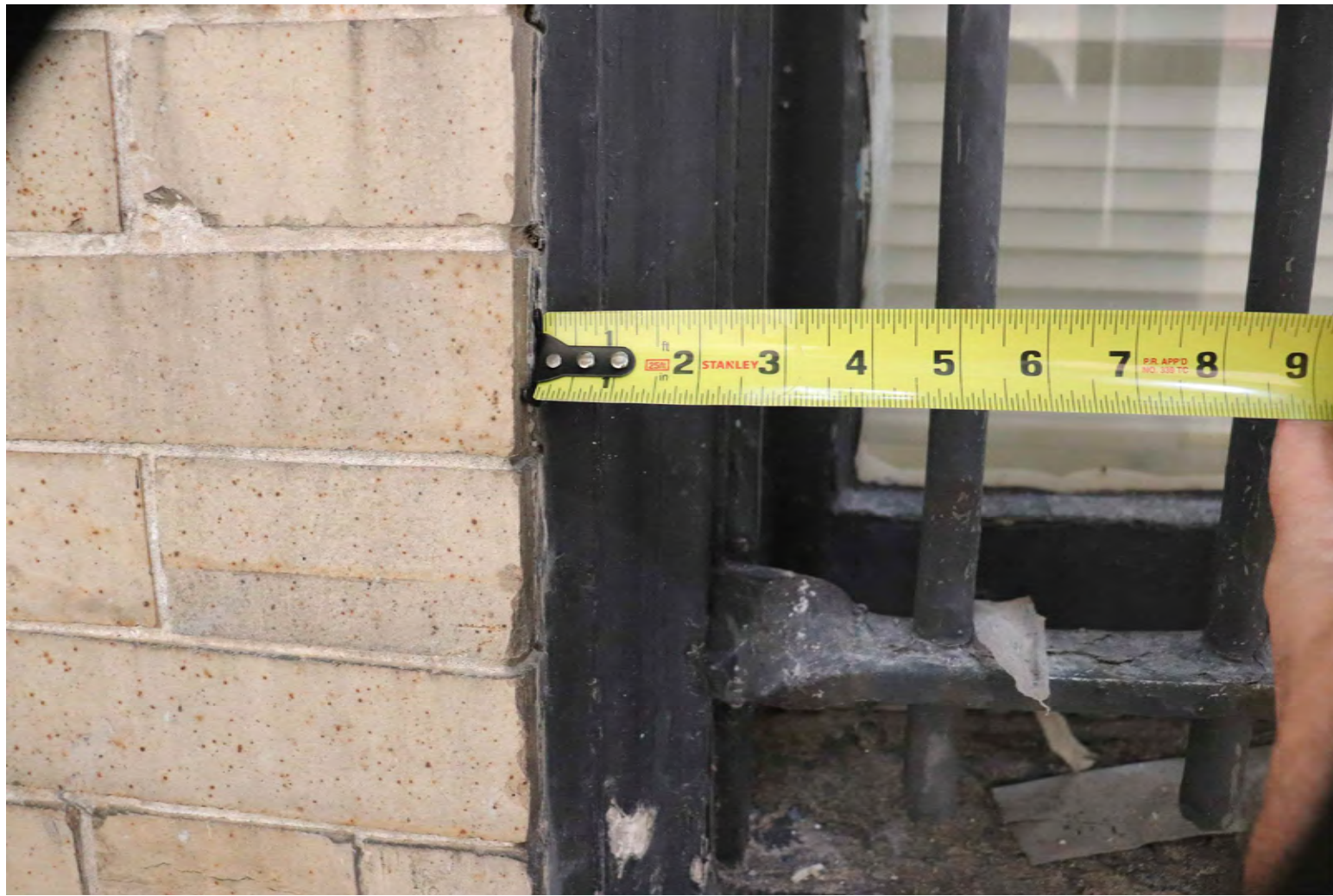
1 Existing / Original Wood Brickmould - Window Left Jamb
