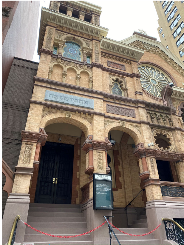
1 ST FLOOR ENTRANCE
