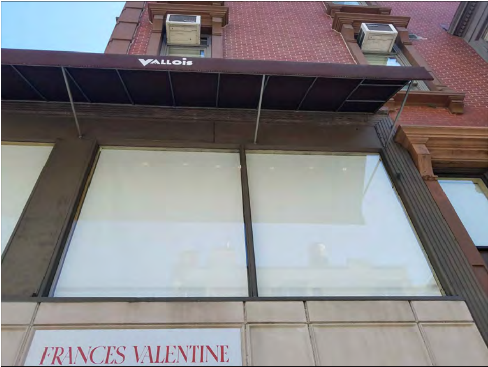
DETAIL OF UPPER PLASTIC PILASTER AND "HISTORIC" FRAME
