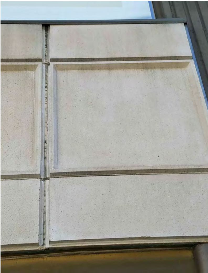
DETAIL OF STOREFRONT SPANDREL WITH TRAVERTINE PIECES
