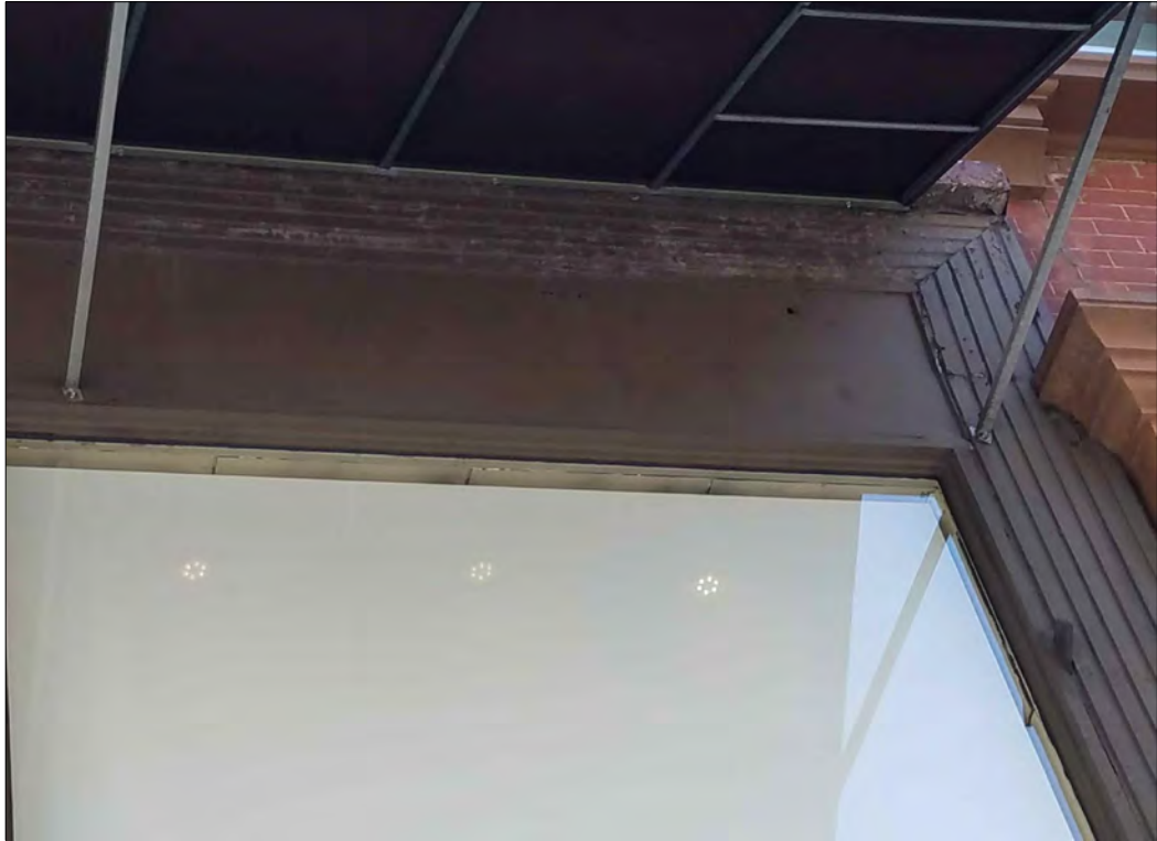
DETAIL OF UPPER PLASTIC PILASTER, SHOWING HORIZONTAL PART
