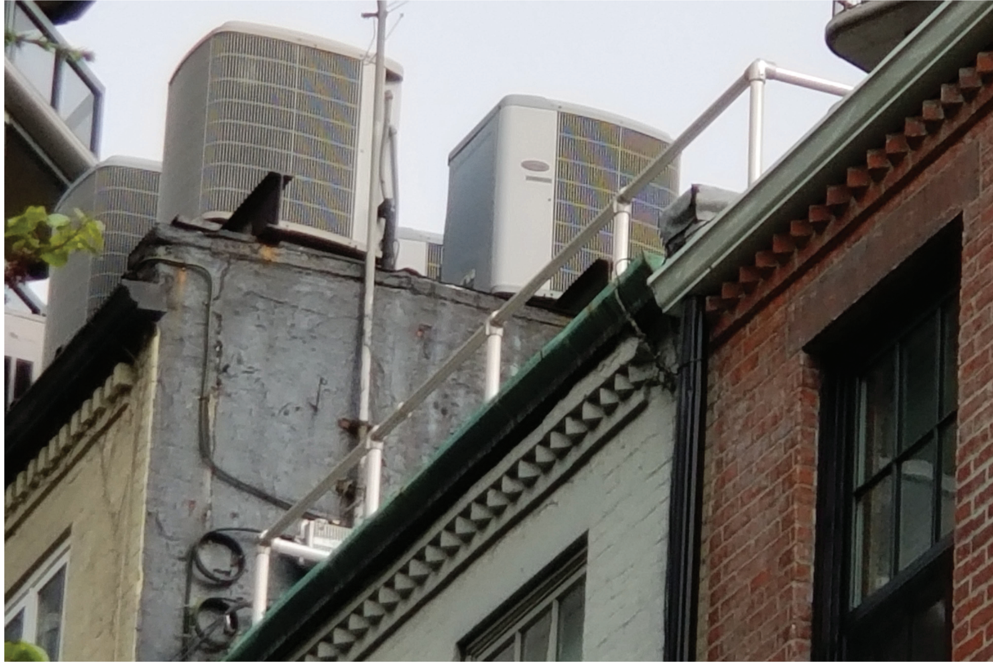
PHOTOGRAPH: ADJACENT BUILDINGS TO THE WEST OF THE PROPERTY, NOTE UNEVEN BUILDING HEIGHTS, MECHANICAL EQUIPMENT AT BUILDING REAR WALL EDGE, RAILINGS AT EDGE, AND DIFFERENT CORBEL TYPES
