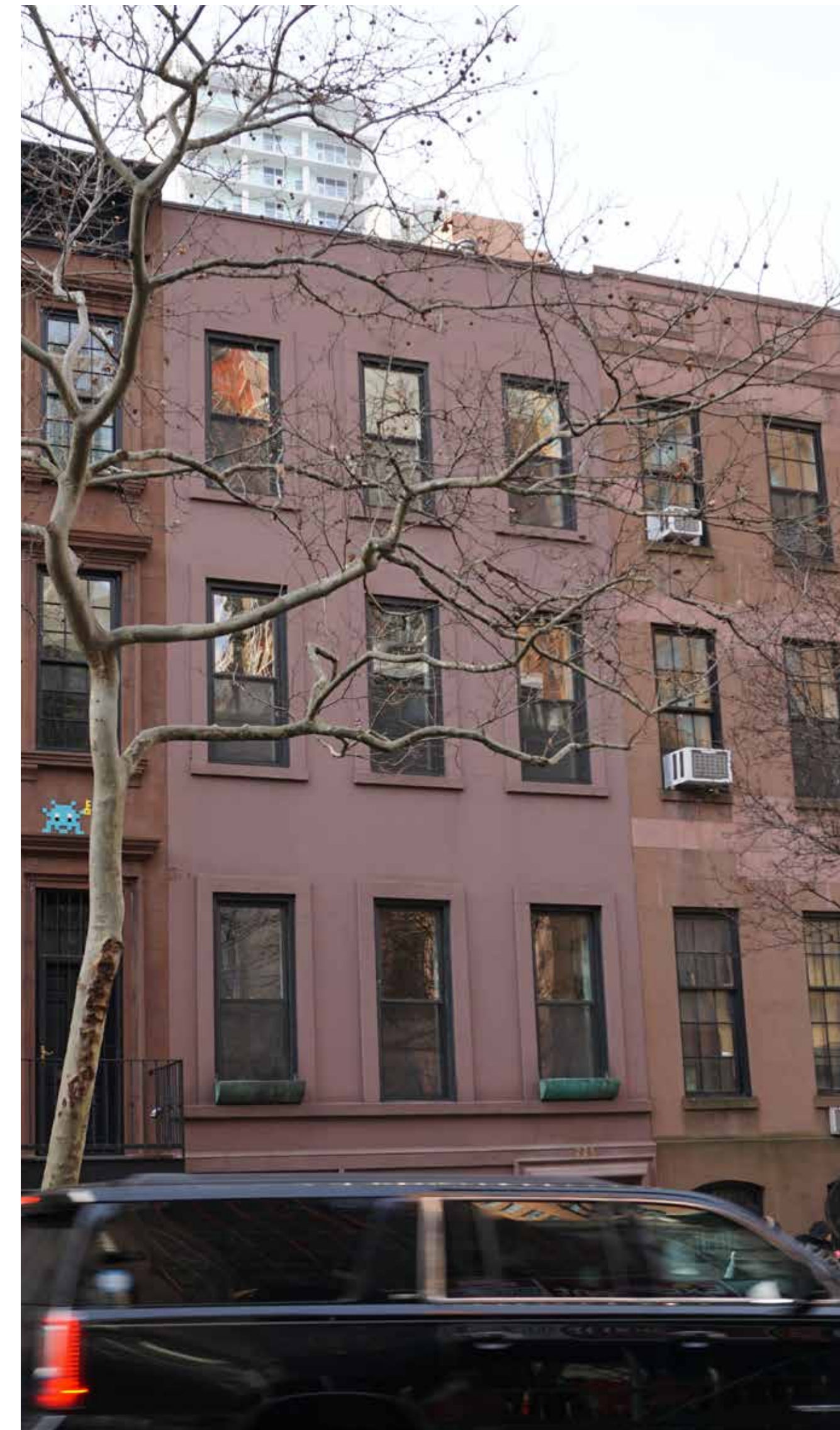
PHOTOGRAPH OF 220 EAST 61ST STREET NORTH (FRONT) FACADE
