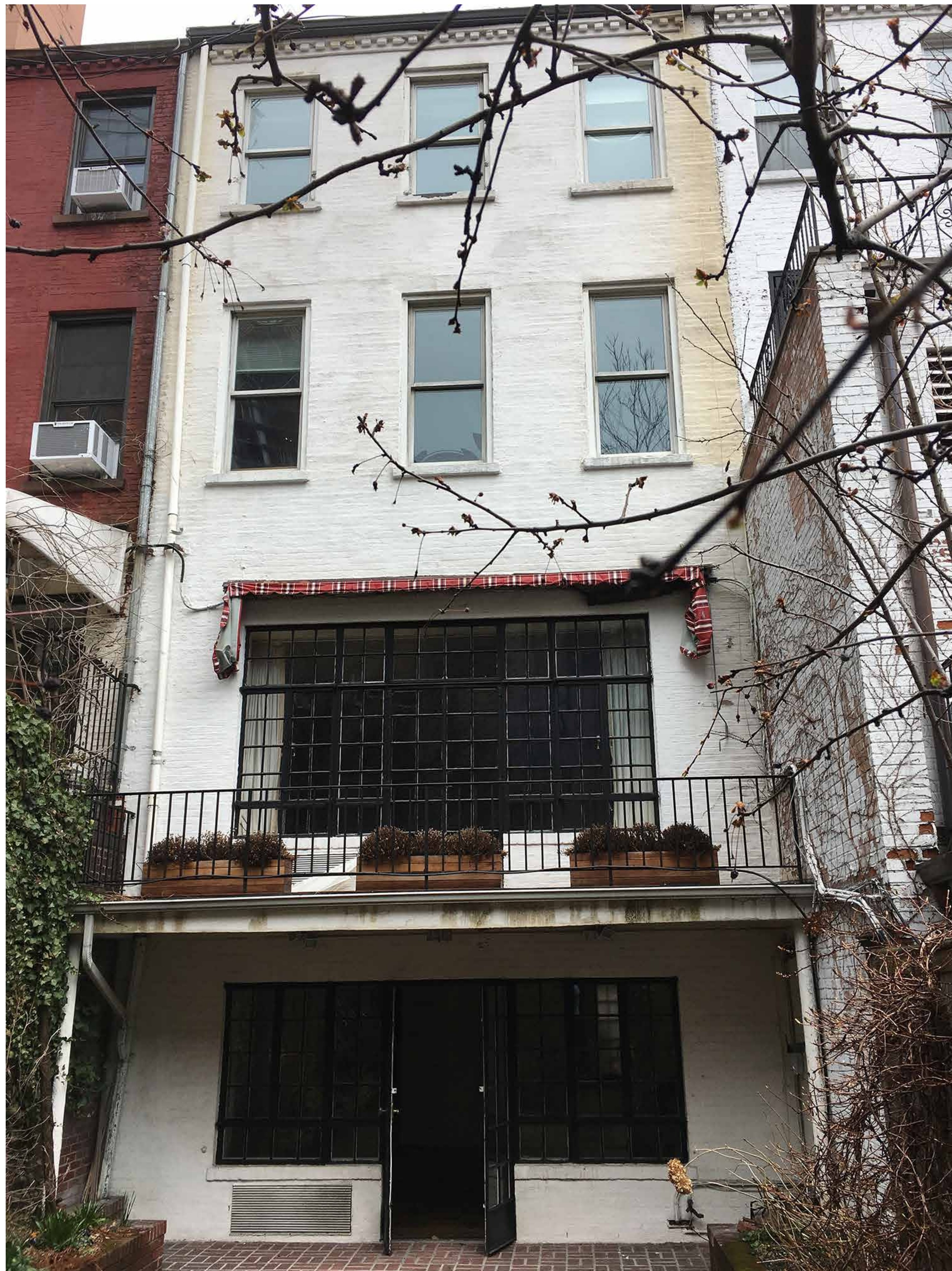
EXISTING CONDITION - PRE-CONSTRUCTION OF ROOFTOP ADDITION
