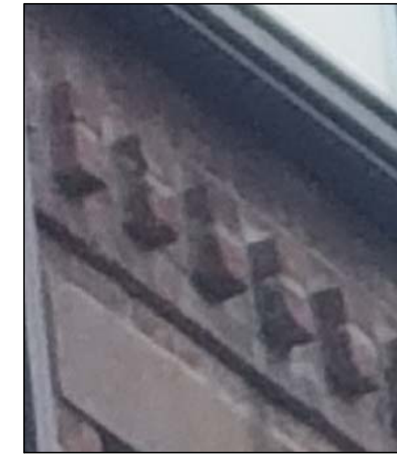
CORBEL TYPE 1A SOLDIER BRICK EXTRUSION BRICKS STACKED TO RESEMBLE SOLDIER COURSE
