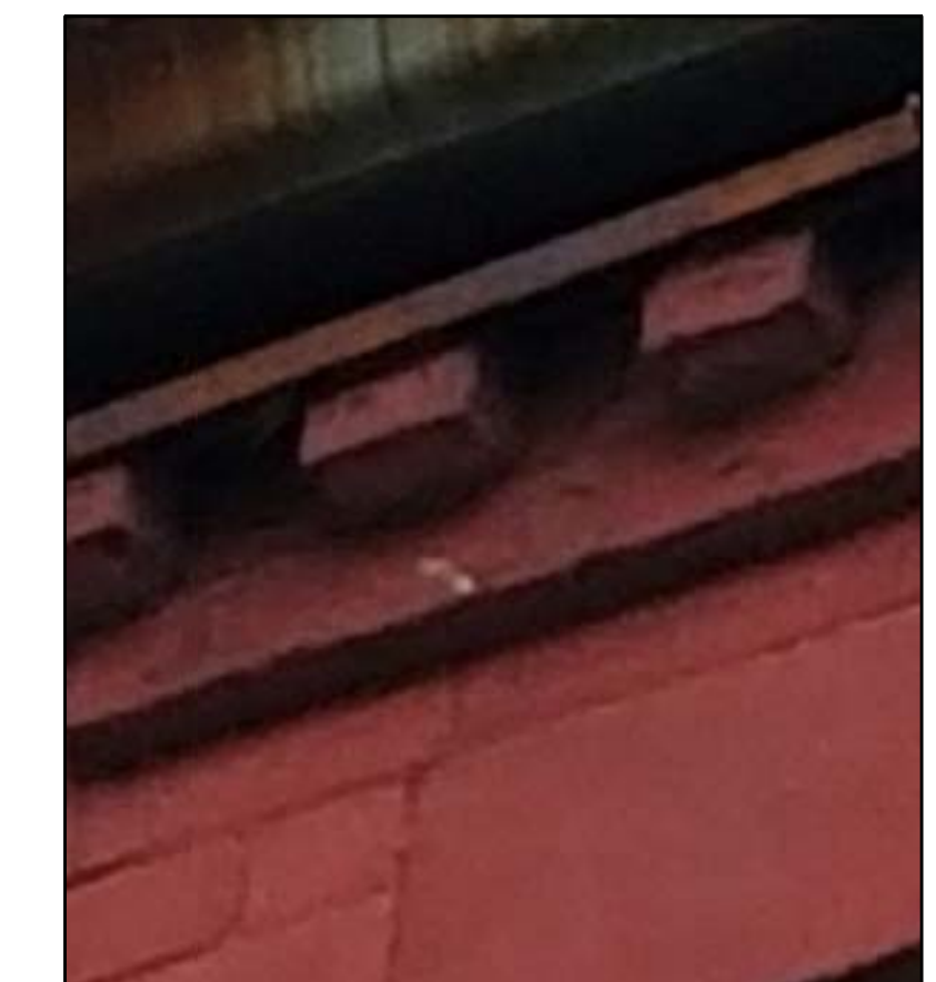
CORBEL TYPE 2B SQUARE BRICK EXTRUSION THIN BRICK LEDGE ON TOP
