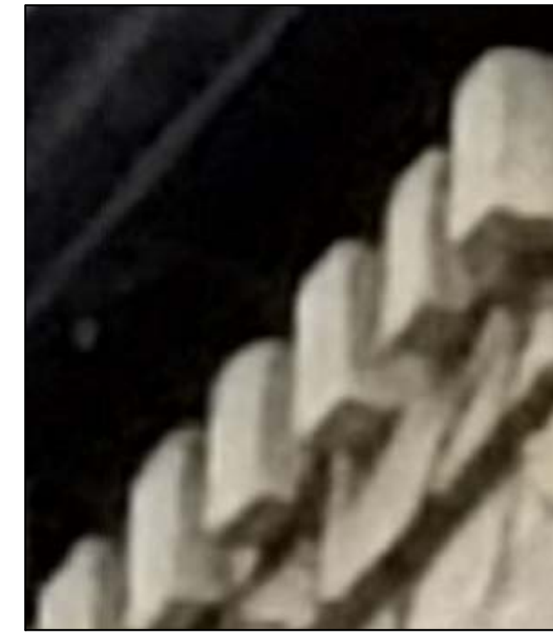
CORBEL TYPE 1 SOLDIER BRICK EXTRUSION
