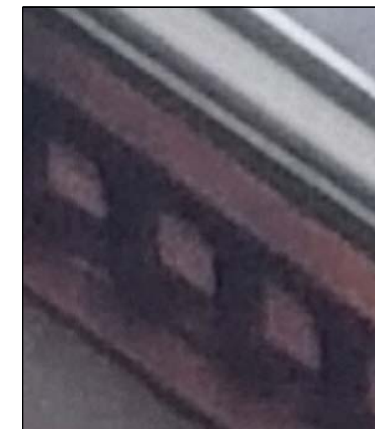
CORBEL TYPE 2A SQUARE BRICK EXTRUSION BRICK LEDGE ON TOP
