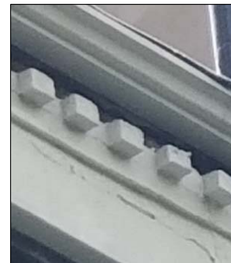
CORBEL TYPE 2 SQUARE BRICK EXTRUSION
