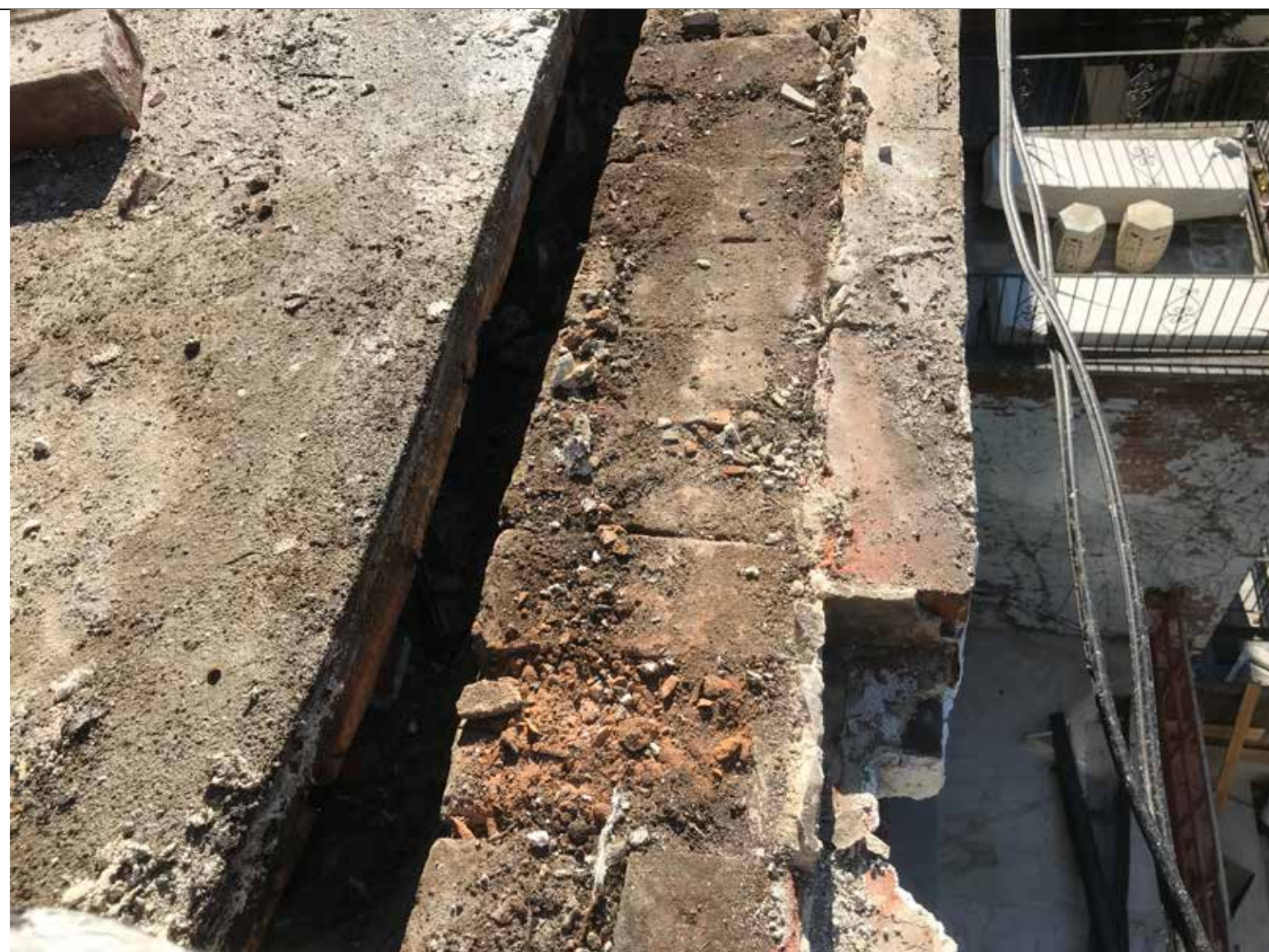
PHOTOGRAPH 01: REAR PARAPET WALL AT BRICK CORBEL, NOTE SEPARATION BETWEEN ROOF SLAB AND WALL AND LOSS OF BRICK CORBEL. SEPTEMBER 4, 2018
