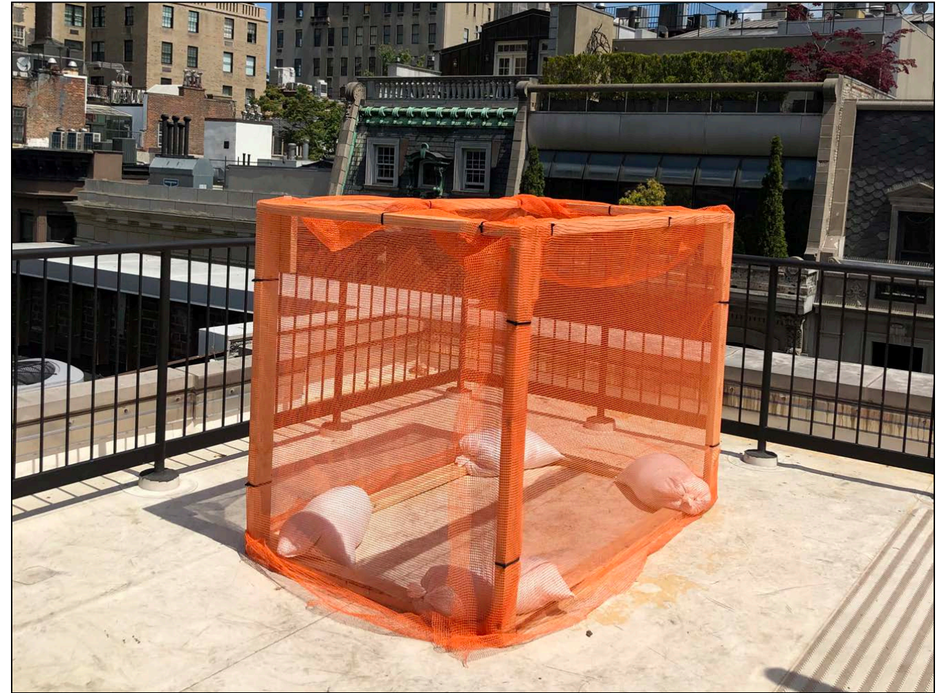
Mockup Roof View 7: Looking North
