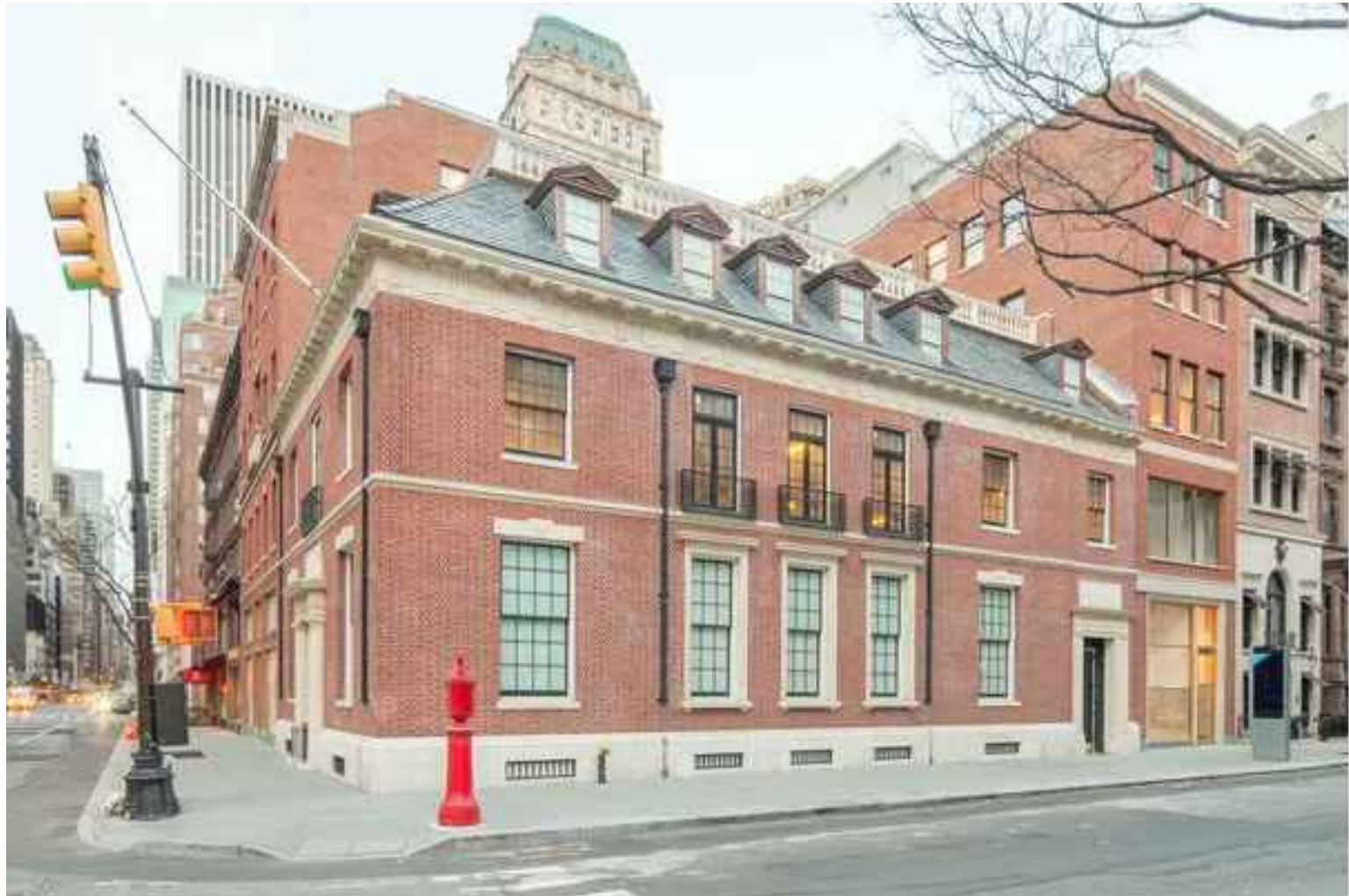
2 EXISTING PHOTO - E 63RD STREET NTS
