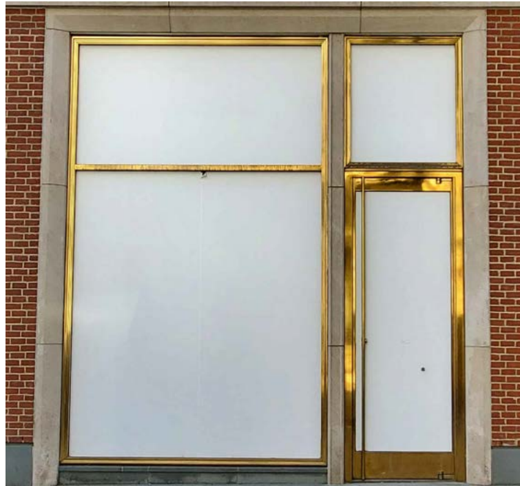
7 BUILDING C ENTRANCE EXISTING PHOTO 1/4"=1'-0"
