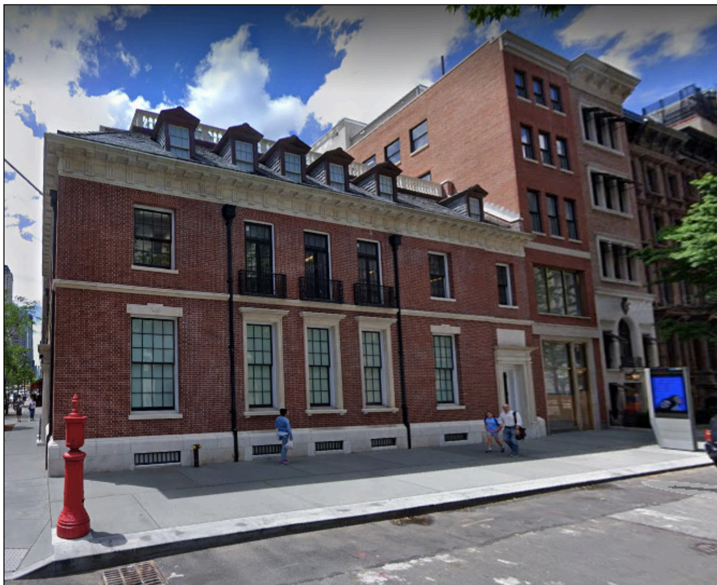
2019 Existing Condition Photo, View West on East 63rd Street
