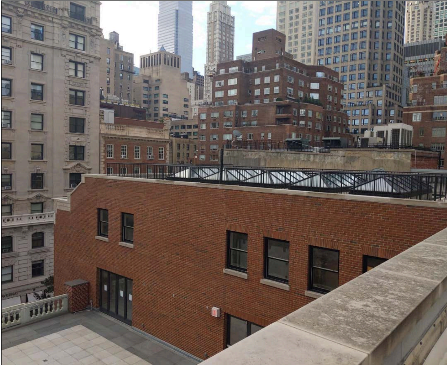
Roof View 1: Looking Southeast
