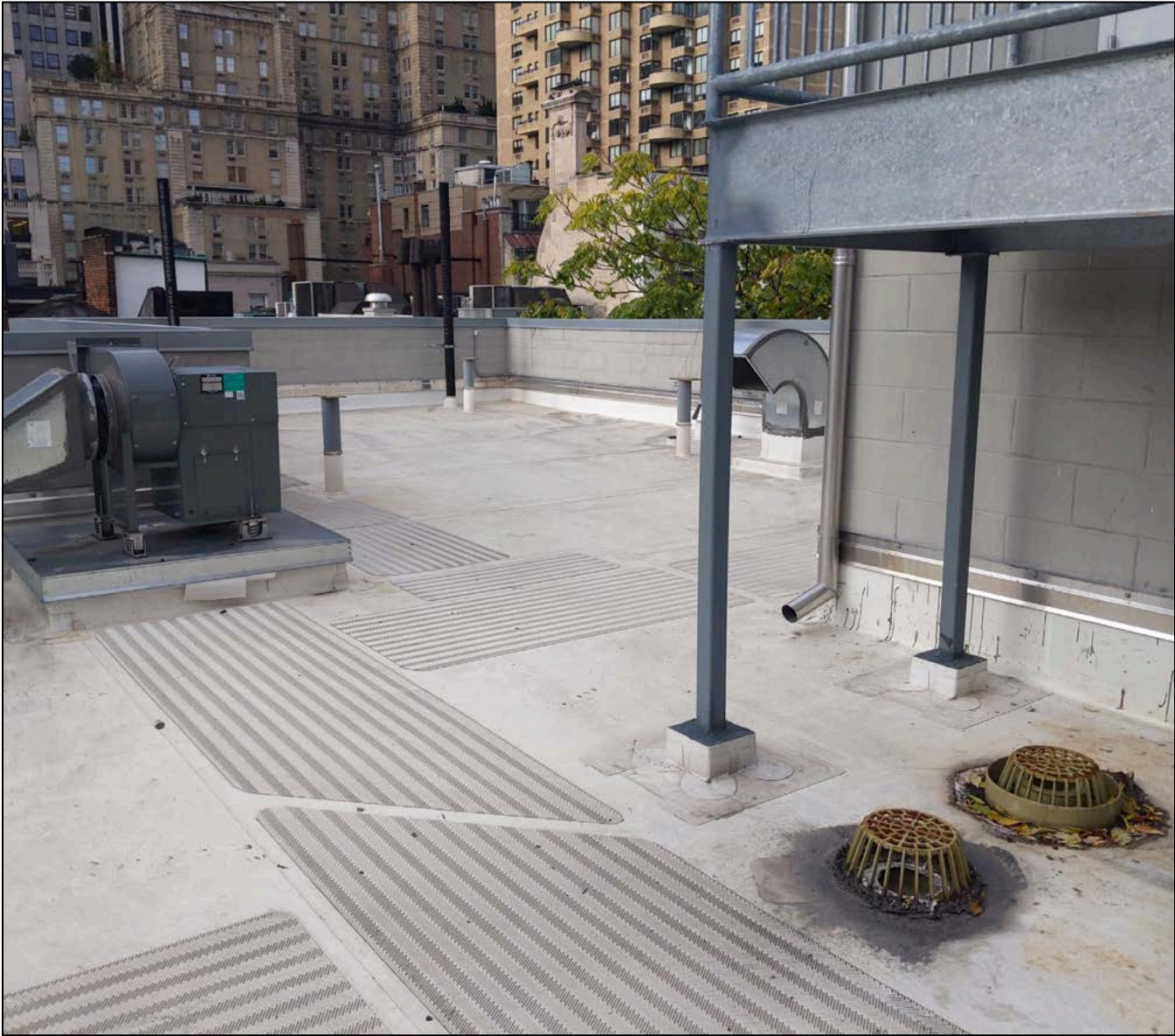
Roof View 8: Looking Southwest
