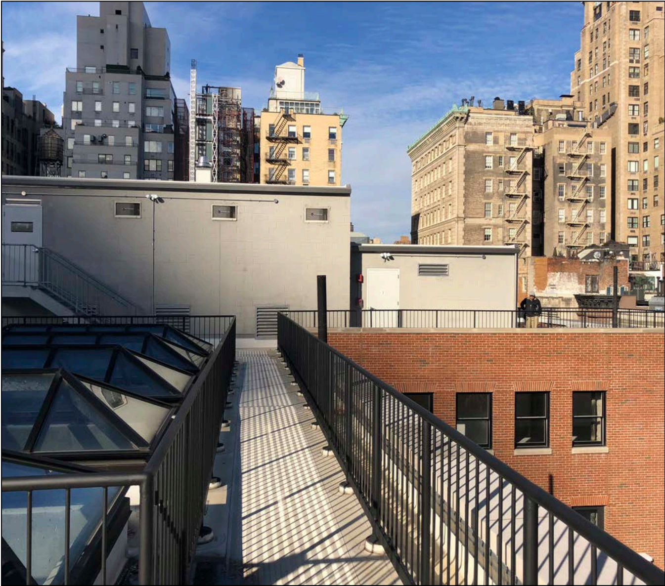
Roof View 4: Looking West
