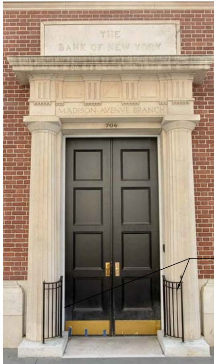
5 BUILDING A ENTRANCE EXISTING PHOTO NTS
