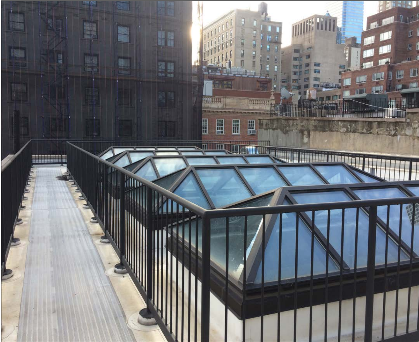
Roof View 3: Looking East
