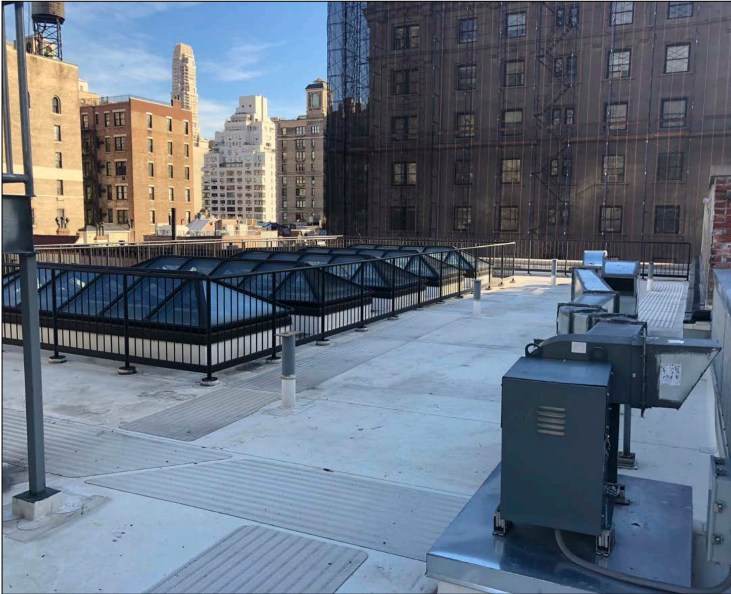
Roof View 7: Looking Northeast
