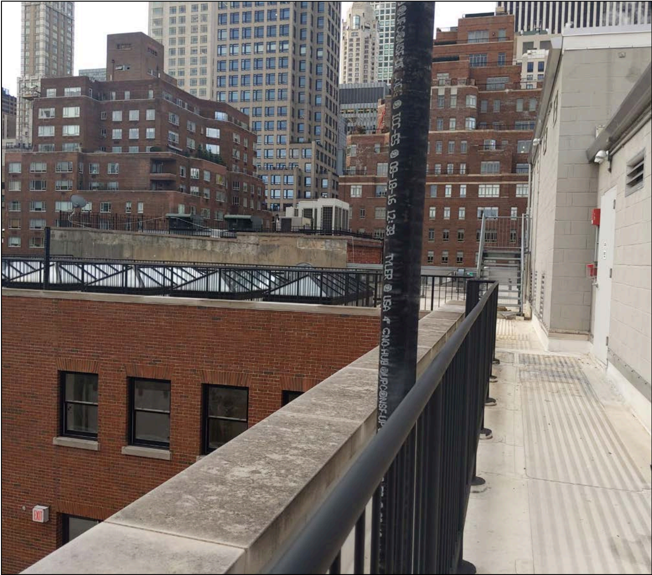
Roof View 2: Looking South
