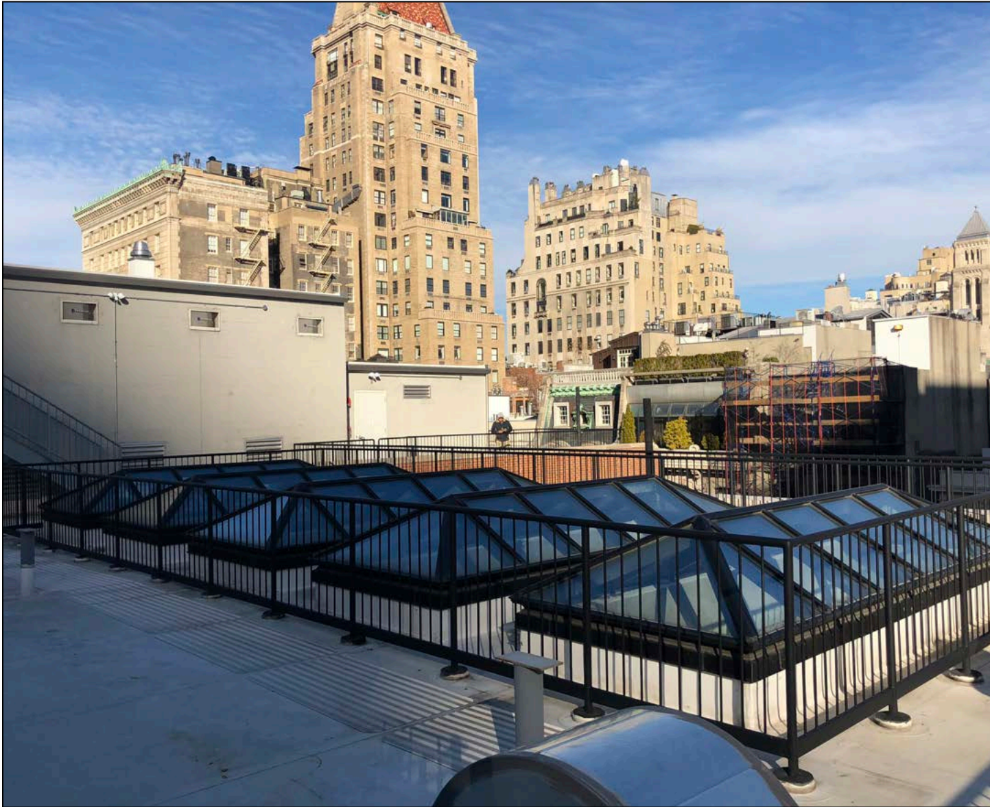
Roof View 5: Looking Northwest
