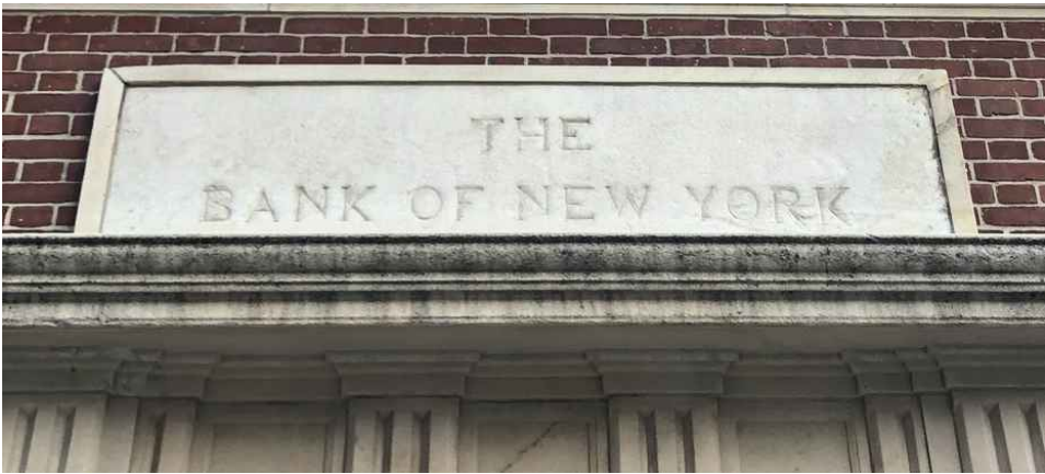
6 EXISTING PHOTO - SIGNAGE L1 @ EXIT D NTS
