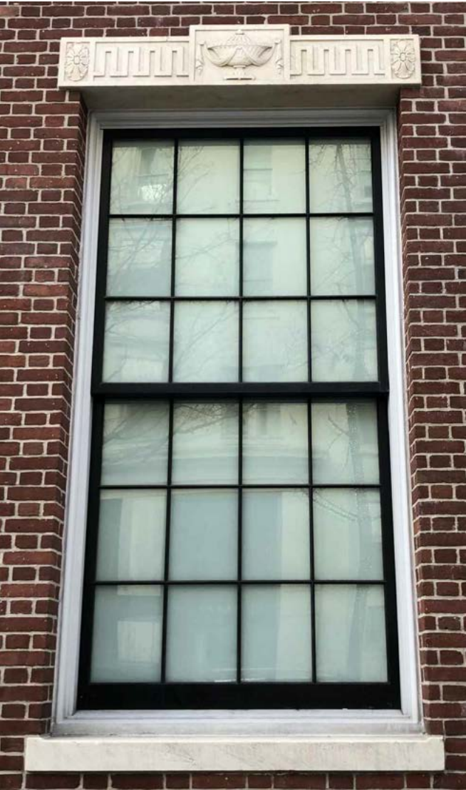
1 PHOTO - EXISTING WINDOW NTS
