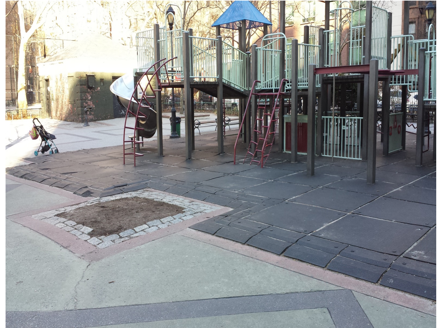
2) Tree Pit in Spray Area
