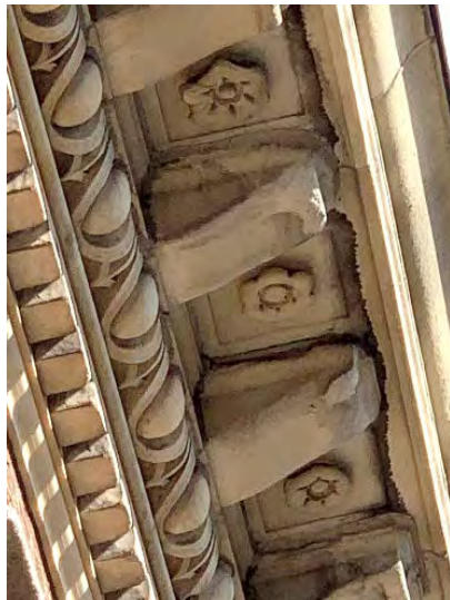
Severely eroded/deteriorated brackets at underside of top cornice.
