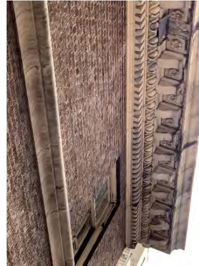
Severely eroded/deteriorated dentils at underside of top cornice.
