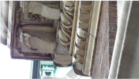
Badly eroded modillions East side on SE corner of cornice.
