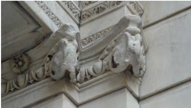
Severely eroded marble capitals at portico's left and right pilasters.
