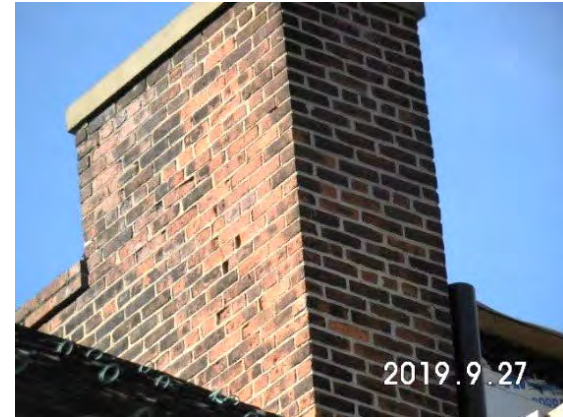
Delaminated brickwork on south face of NE party wall parapet
