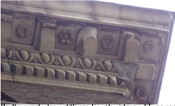
Badly eroded modillions South side on SE corner of cornice.
