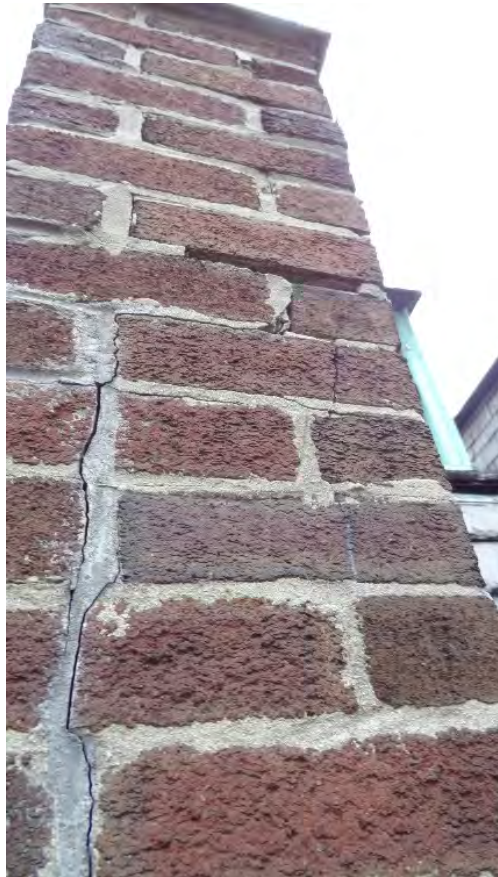
Cracked parapet at NE corner of setback roof
