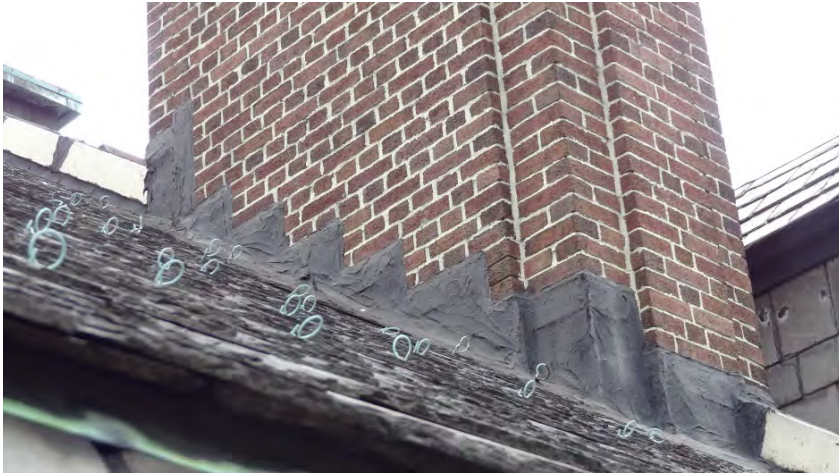
Leaking Roof at NE Chimney – Copper Step Flashing covered in Tar
