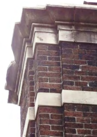
Deteriorated chimney capstone
