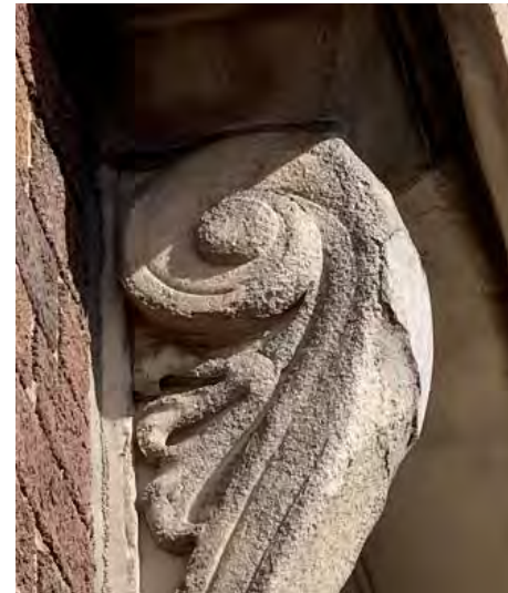
Eroded stone window scrolls at 68 th Street façade.
