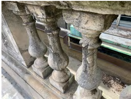
Severely eroded and deteriorated balusters at roof balustrade.
