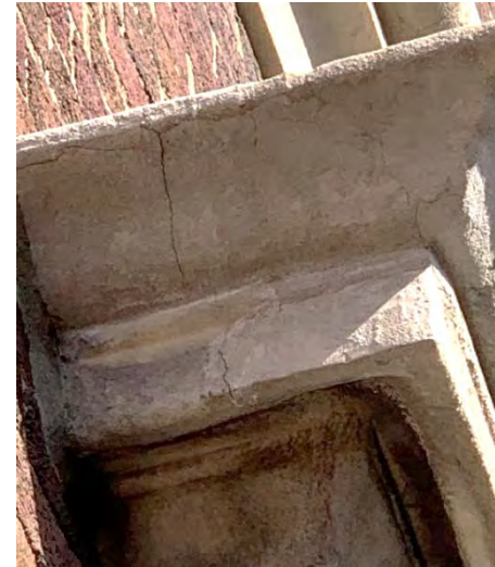
Cracked left side of stone window cornice at 68 th Street façade.
