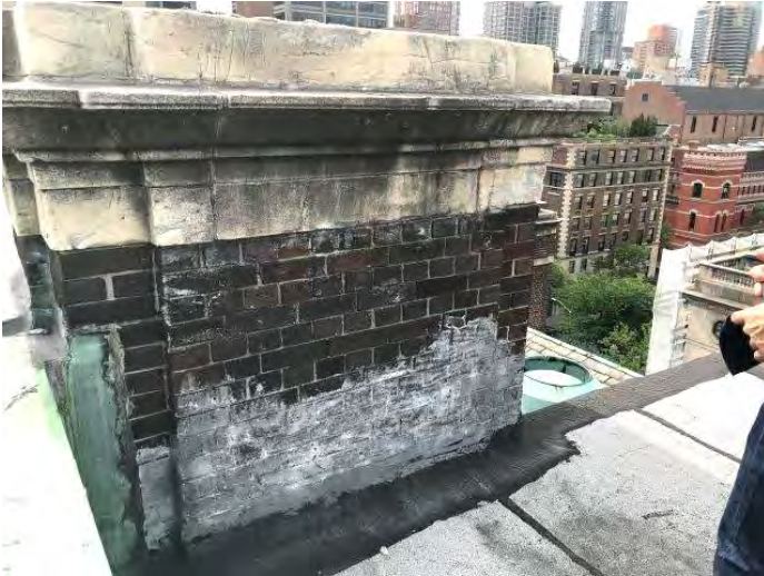
Tarred west face of chimney on east side of elevator bulkhead roof
