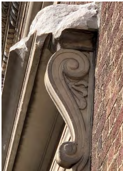
Broken right corner of stone window cornice at 68 th Street façade.
