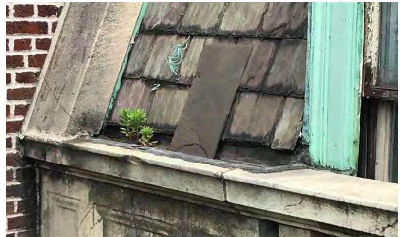
Slate tile fallen off & resting along stone balustrade
