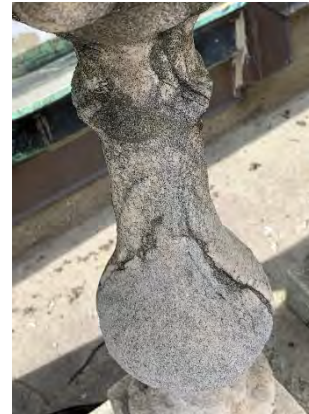
Severely eroded and deteriorated balusters at roof balustrade.
