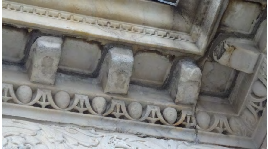
Severely eroded marble dentils at underside of portico cornice.
