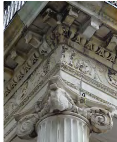
Severely eroded marble capitals at portico's left & right columns.
