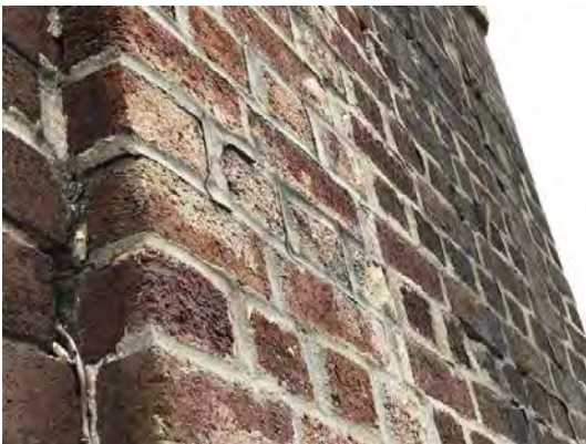
Eroded brickwork and efflorescence at chimney
