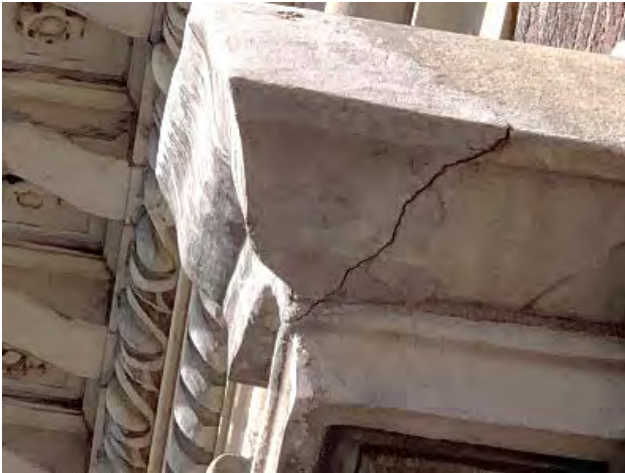
Cracked right corner at previously repaired window pediment at 68 th S façade.
