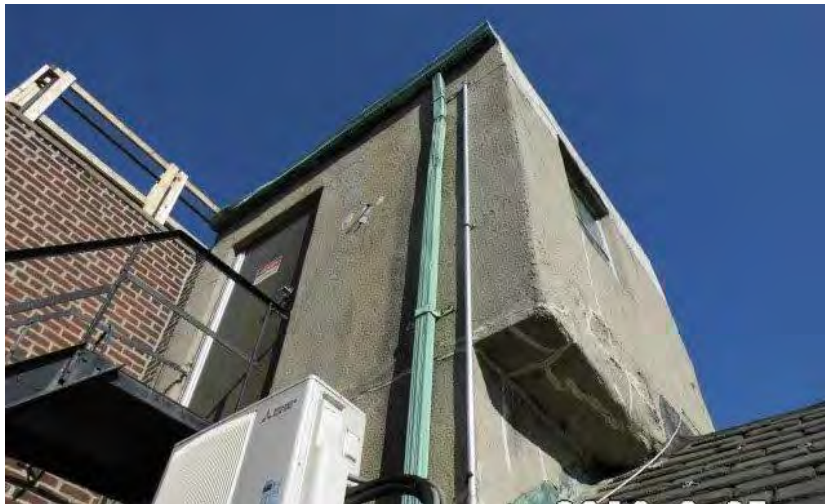
Caulked Cracked Stucco at West & South Walls of Elevator Bulkhead
