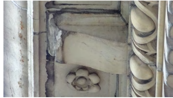
Typical eroded Modillion at cornice
