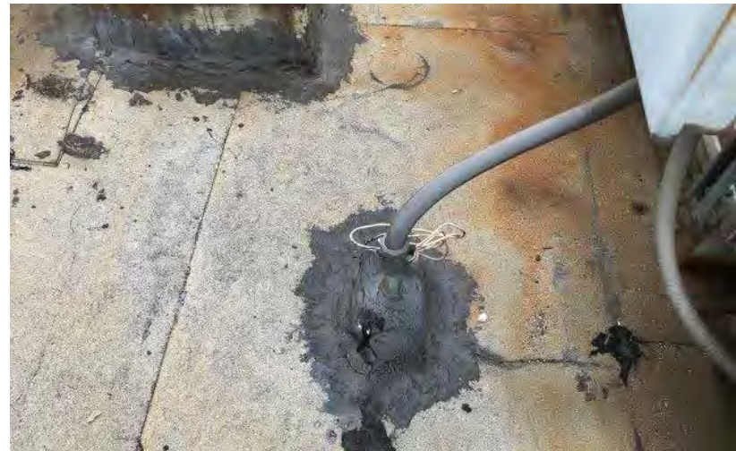
Conduits Penetrated Mechanical Roof
