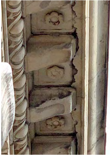
Severely eroded/deteriorated brackets at underside of top cornice.
