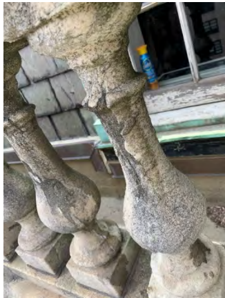
Severely eroded and deteriorated balusters at roof balustrade.
