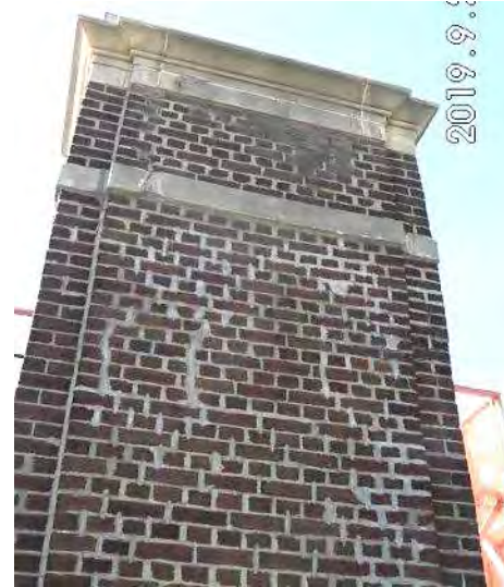
Cracks at chimney
