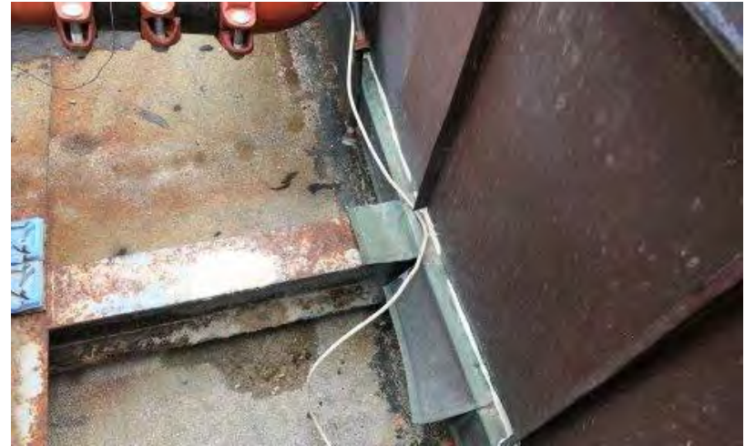
Rusted Damaged Beams at Mechanical Roof
