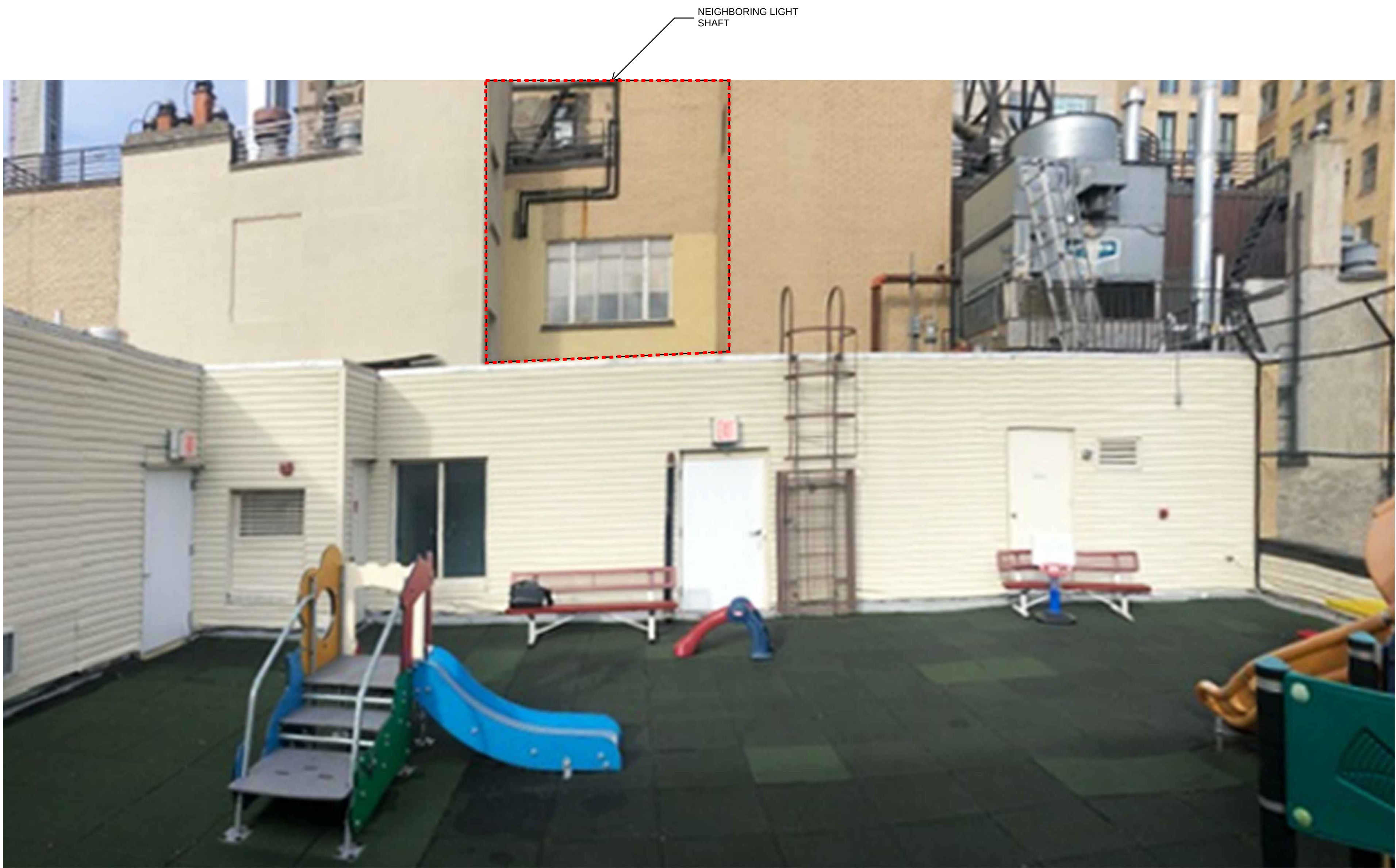
View at roof looking West
