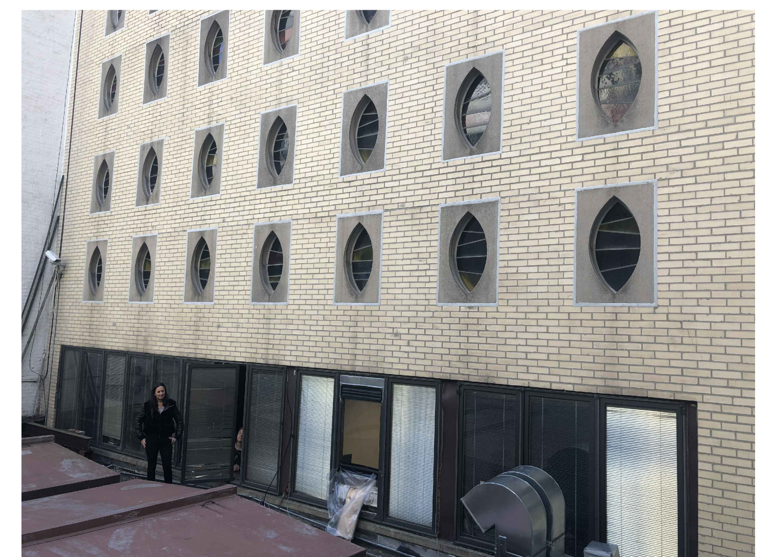
Existing North Elevation (from lower roof of building)
