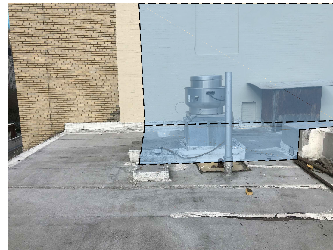
view of existing exhaust flue on roof with proposed footprint of elevator bulkhead
