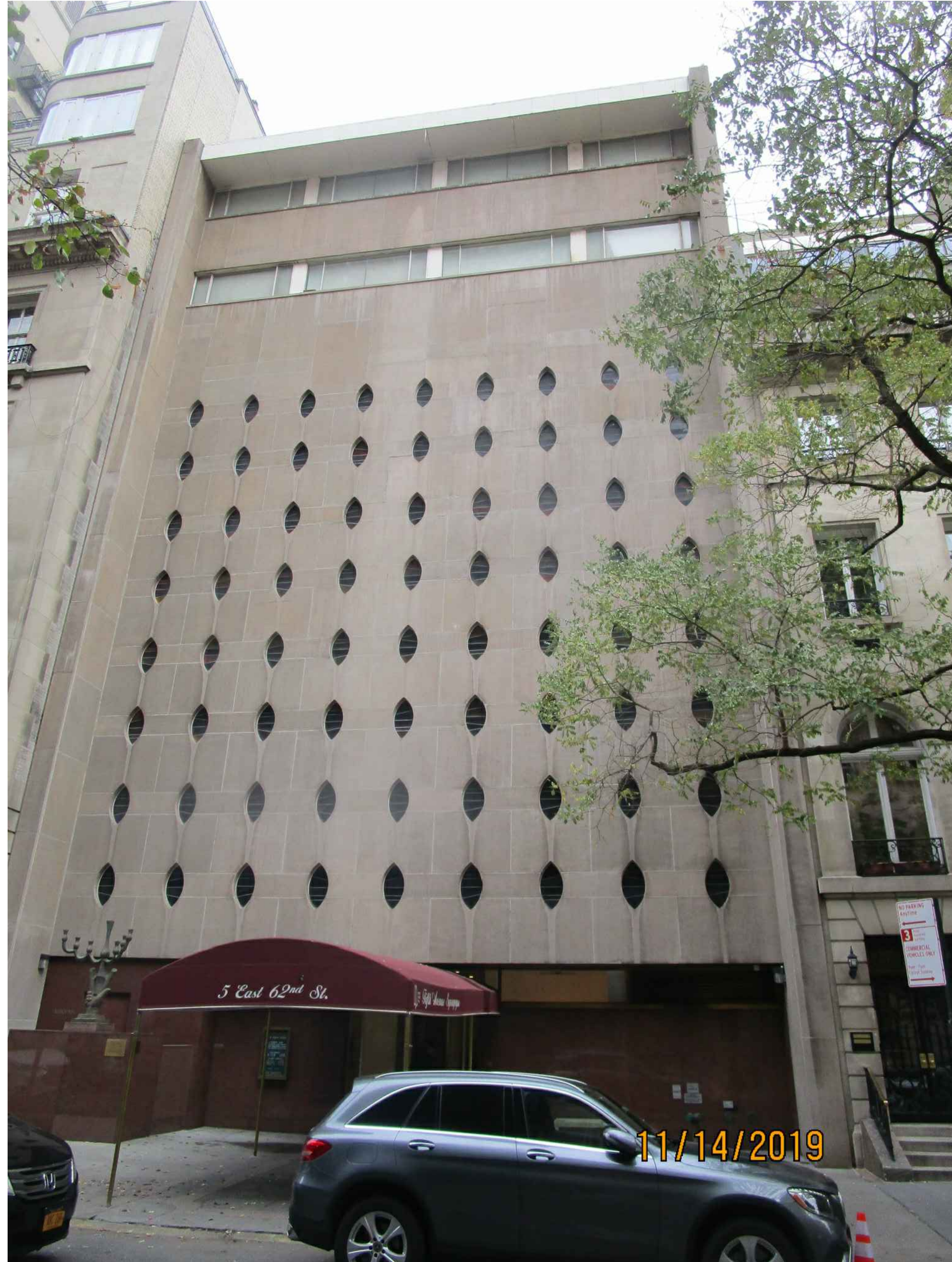
Existing South Elevation (from East 62nd Street)
