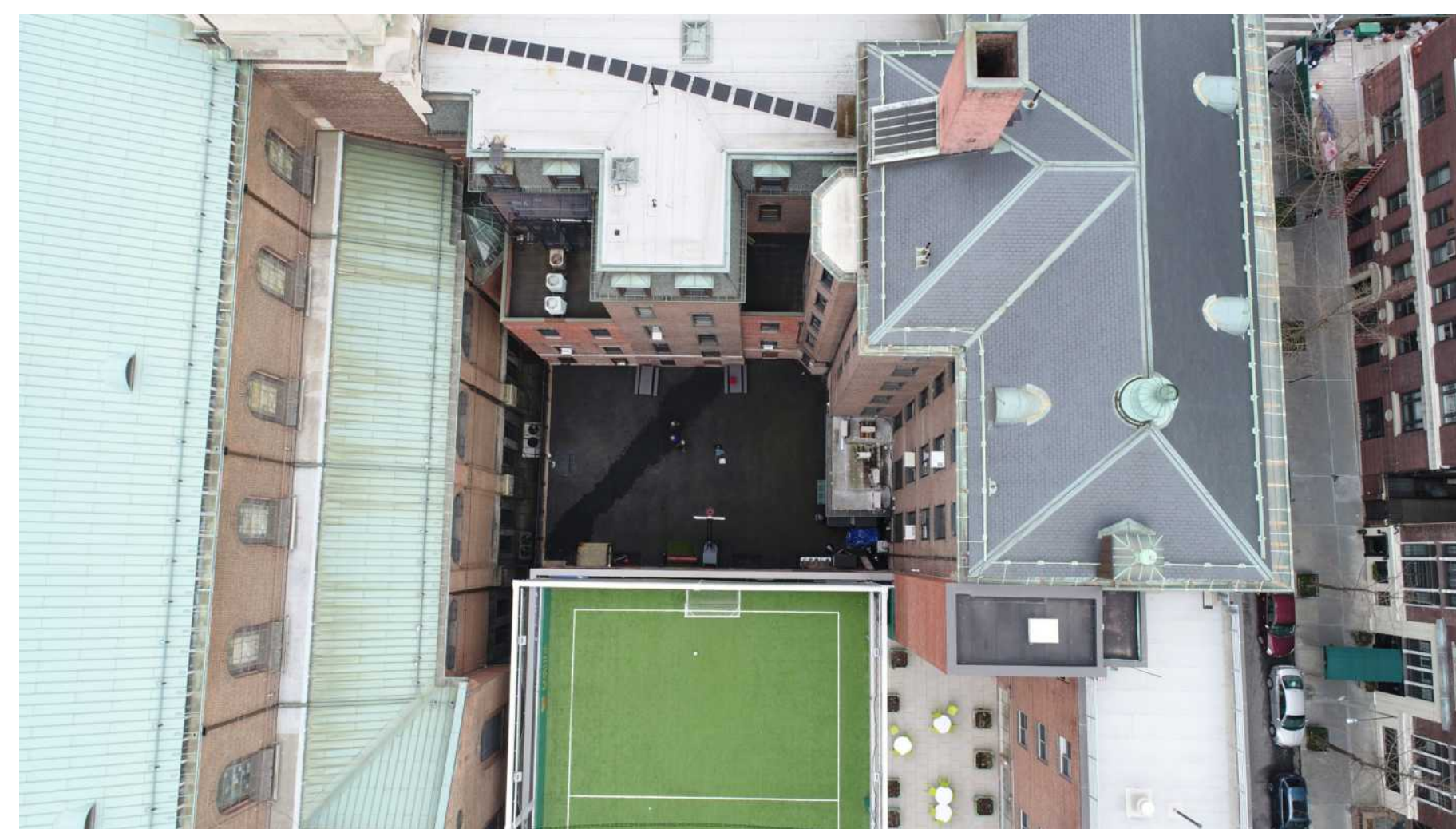
5 Jug Yard looking east
