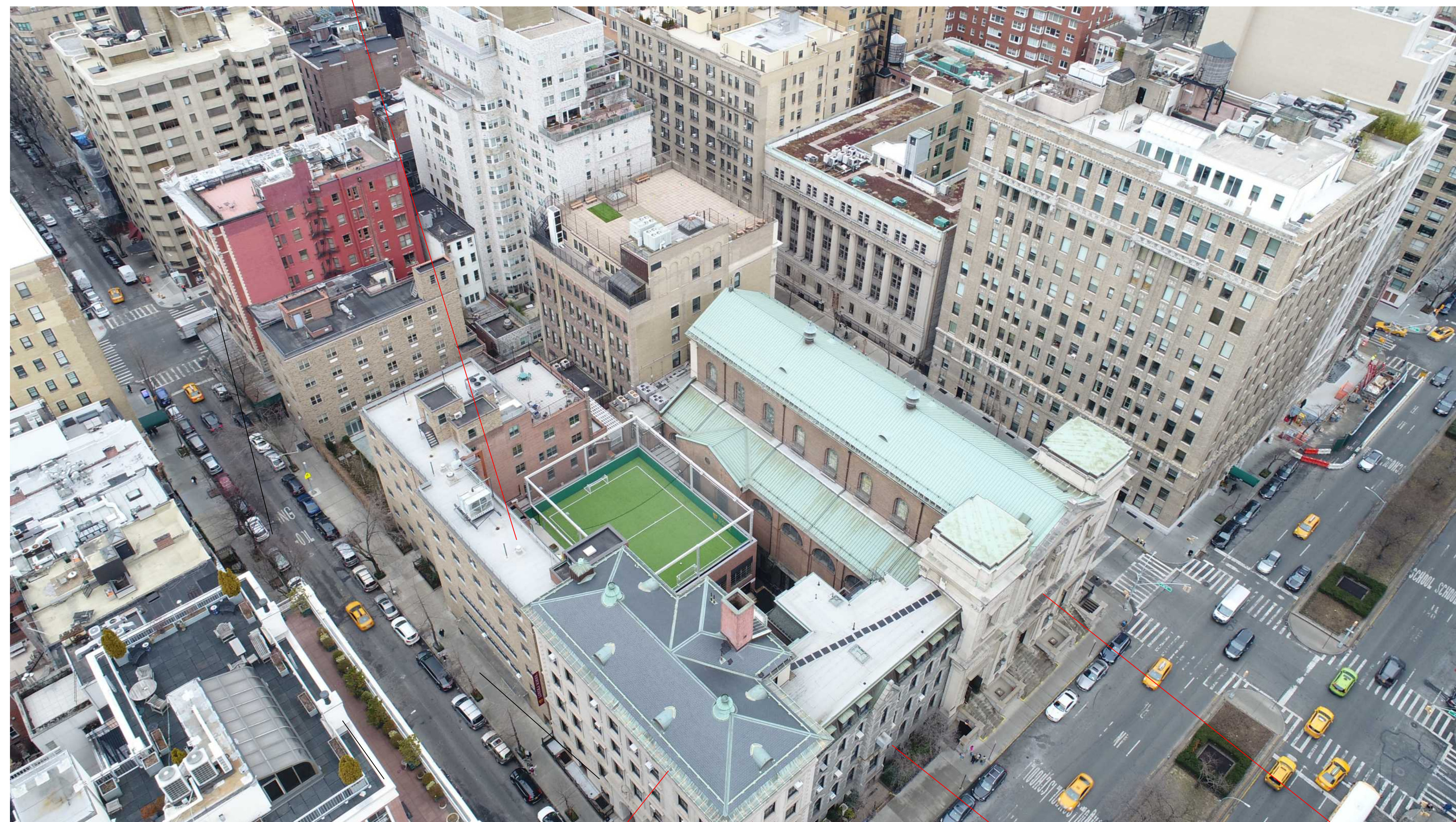
1 Photo looking northwest
