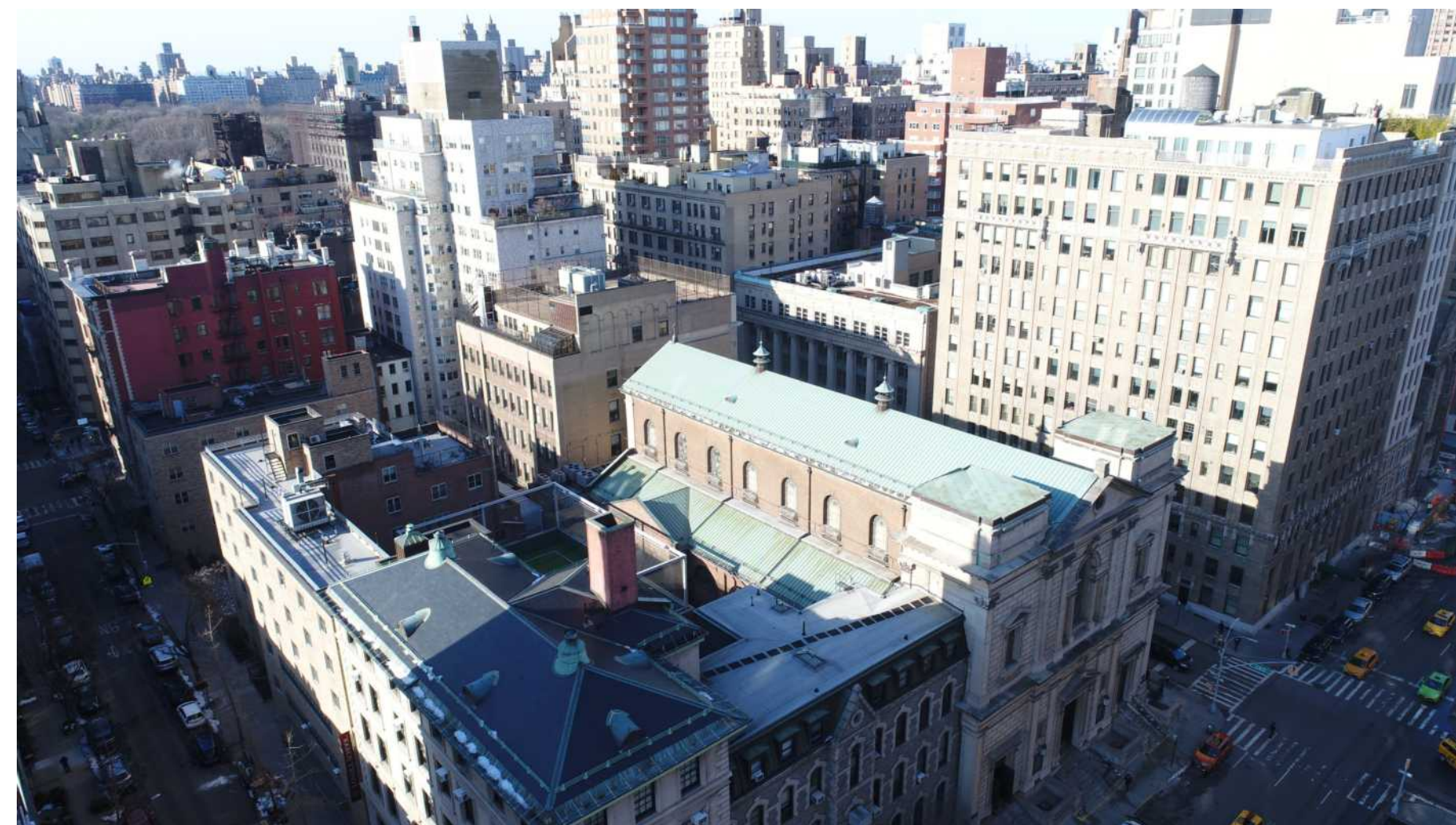
2 Photo looking northwest
