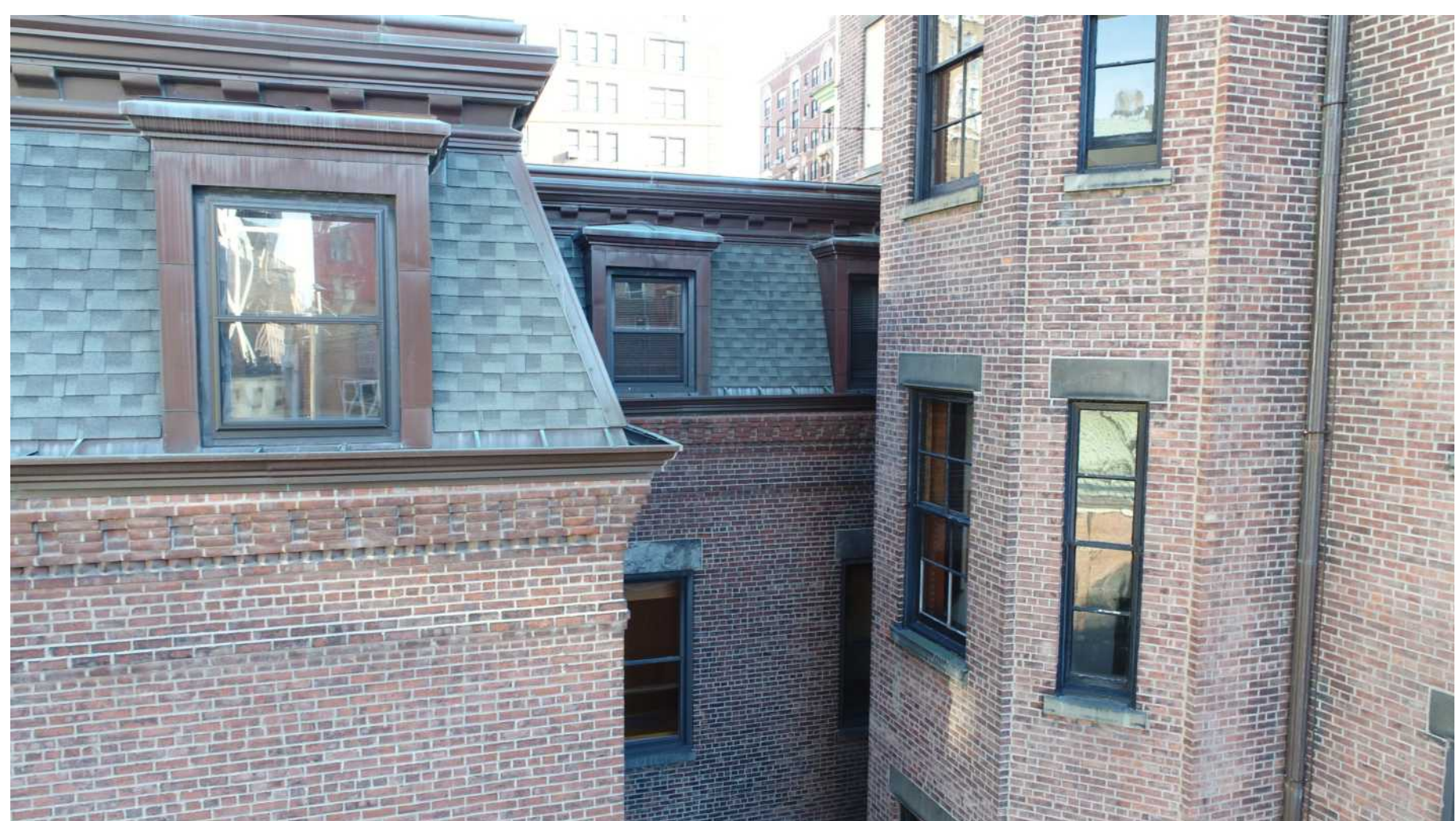
9 Parish House 4th floor window
