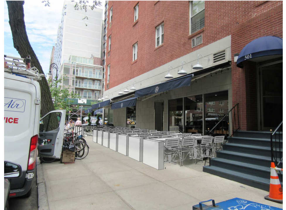
East 86th Street facing west (Site at right)
