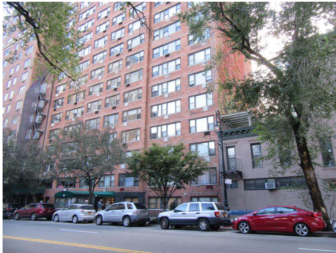
6. View of the south side of East 86th Street facing south (Affected Area at right).
