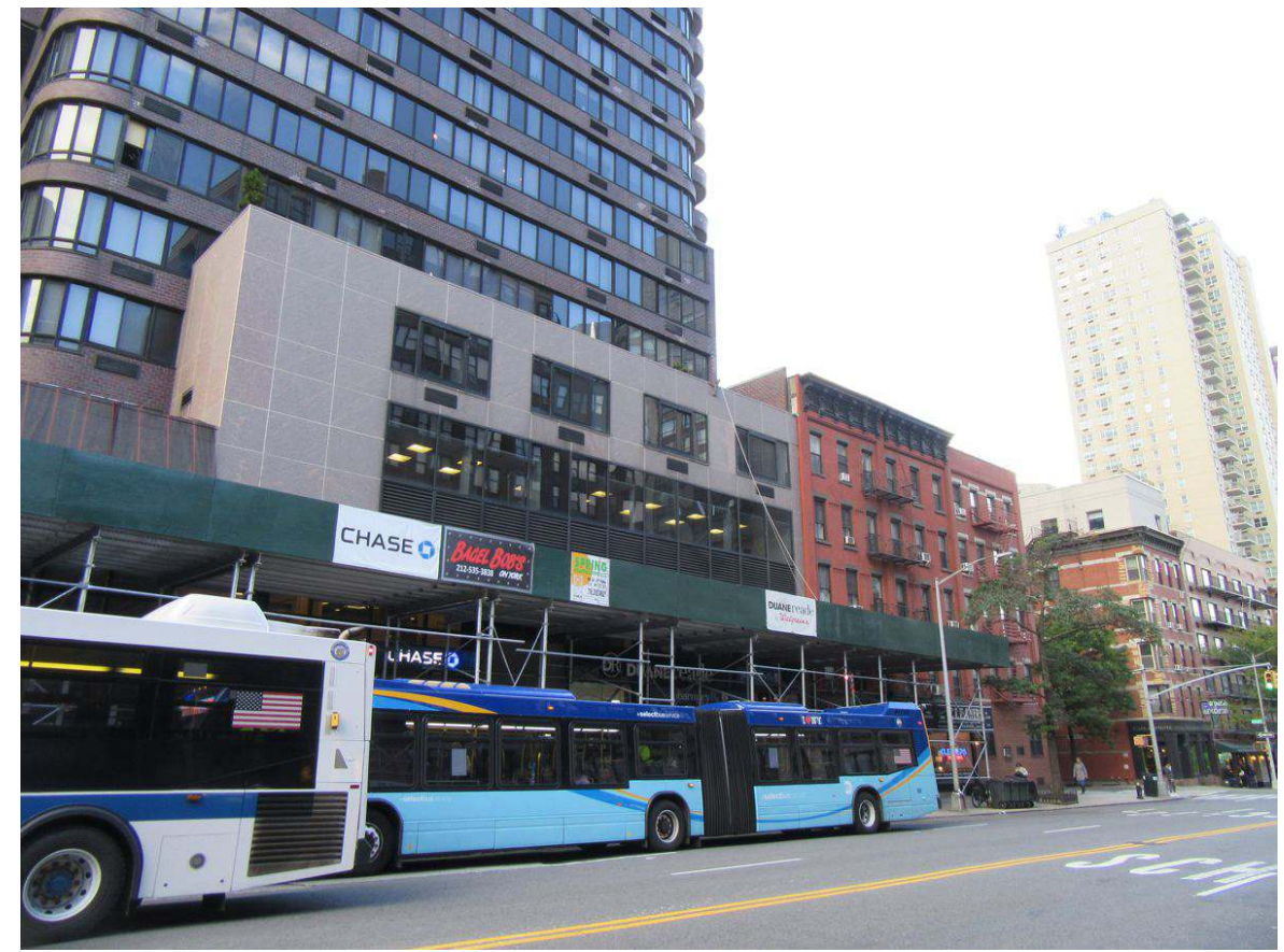
8. View of the west side of York Avenue facing northwest.
