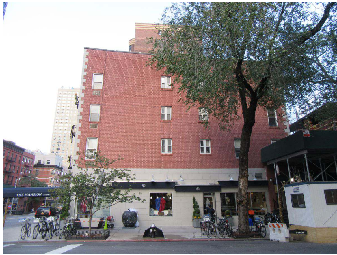
4. View of the Affected Area facing northeast from East 86th Street.
