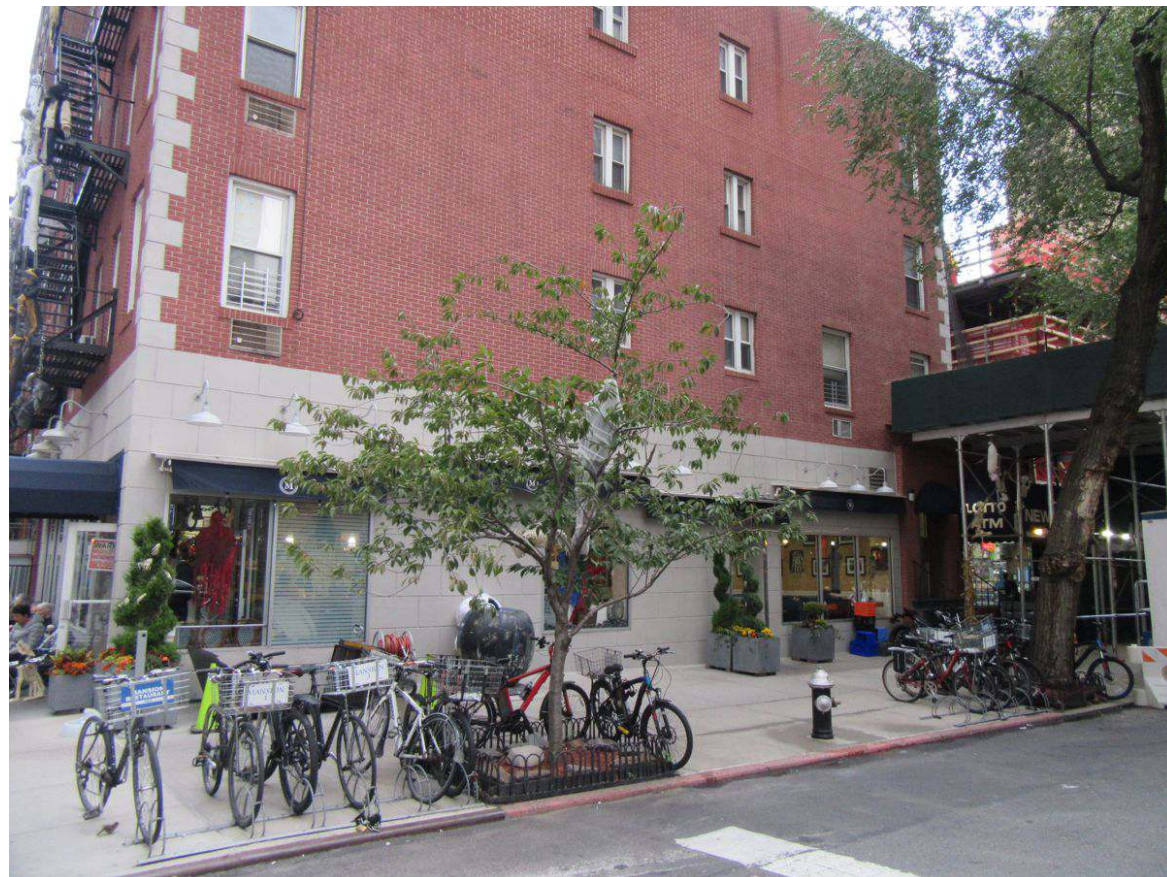
18. View of the Affected Area facing northeast from East 86th Street.
