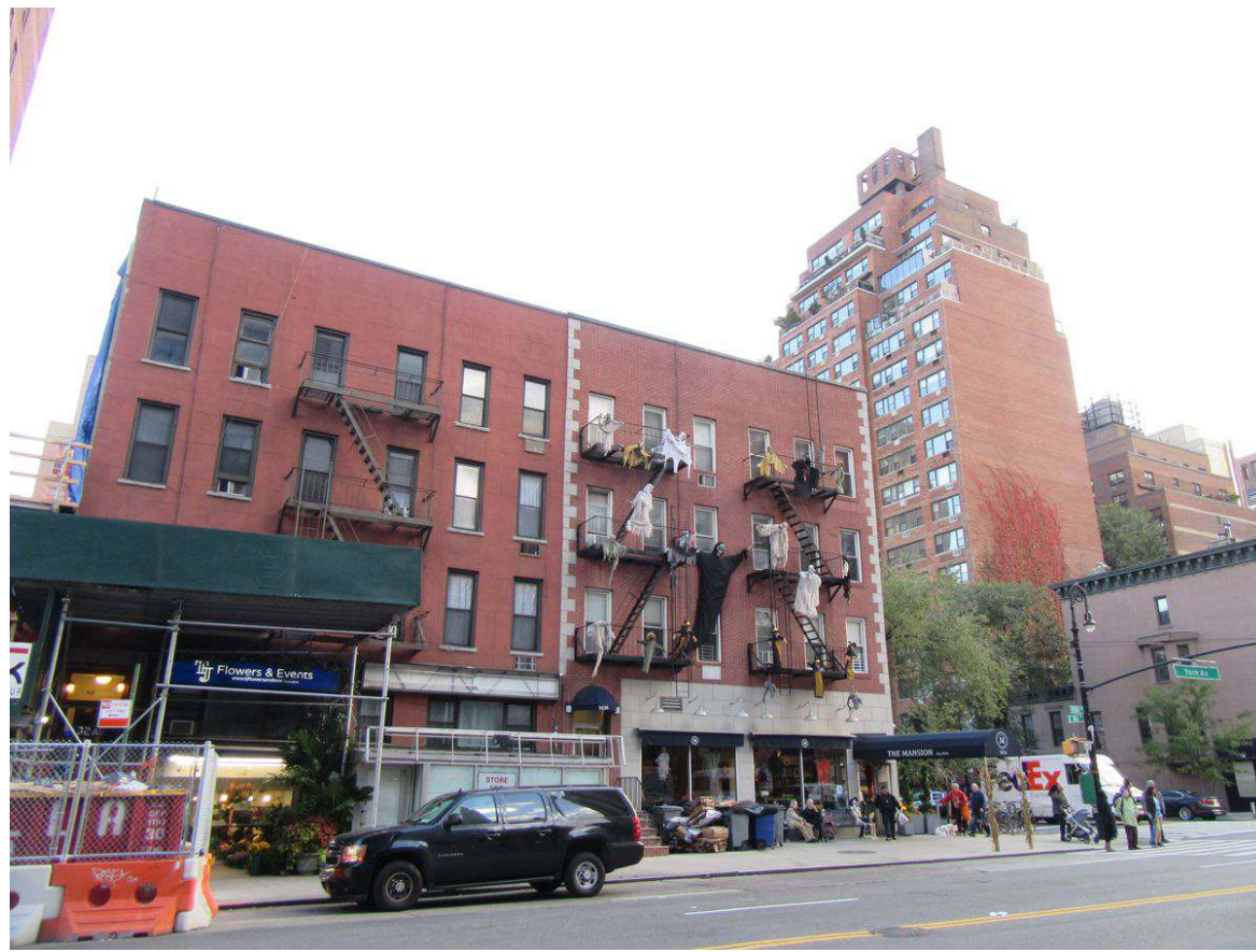
1. View of the east side of York Avenue facing south.
