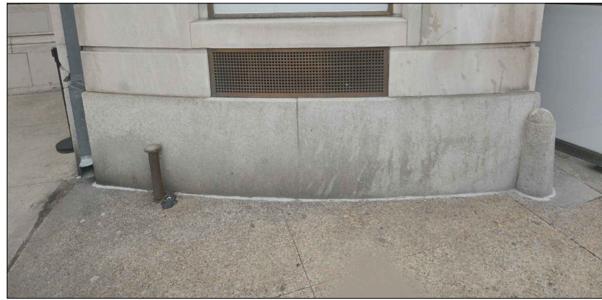
1b PHOTO OF EXISTING SIDEWALK AT FRONT FACADE Scale: 1/2" = 1'-0"
