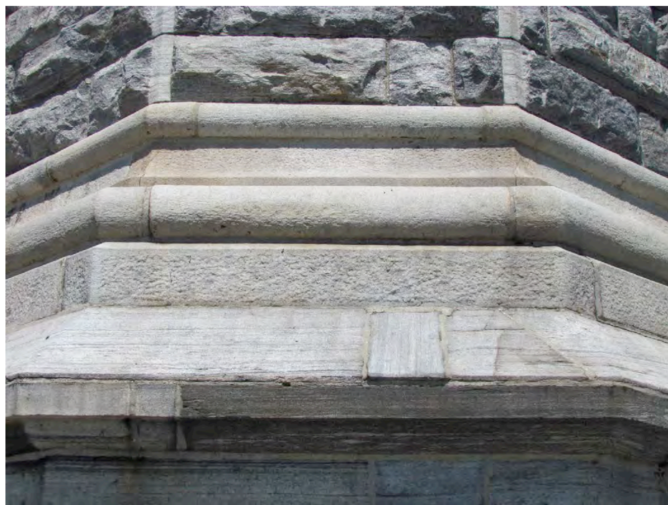
3 STONE CRACKING at MOLDING BASE at DISPARATE LOCATIONS
