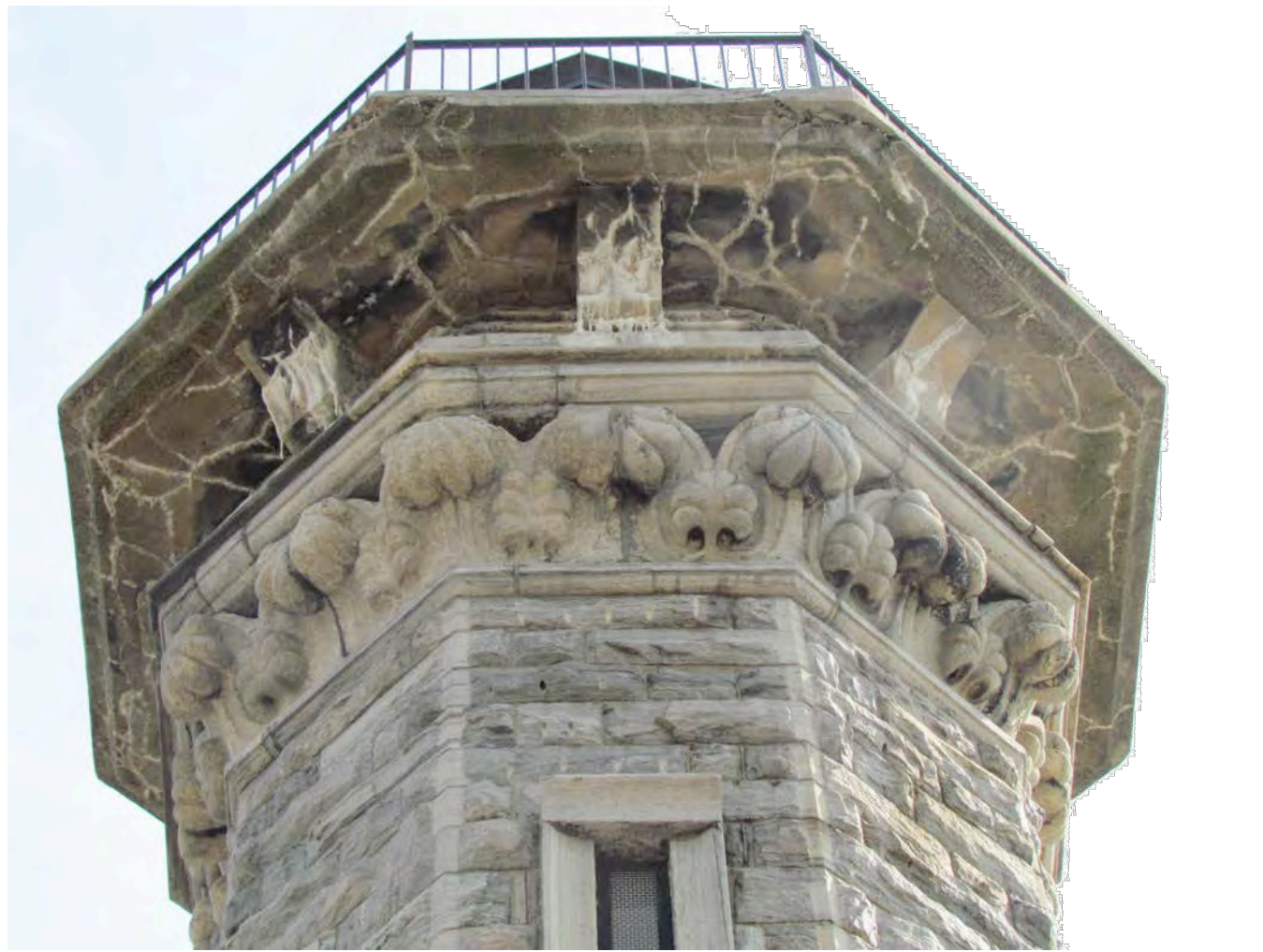
6 DETERIORATED, NON-ORIGINAL CONCRETE DECK ALL ELEVATIONS, TYPICAL CONDITION
