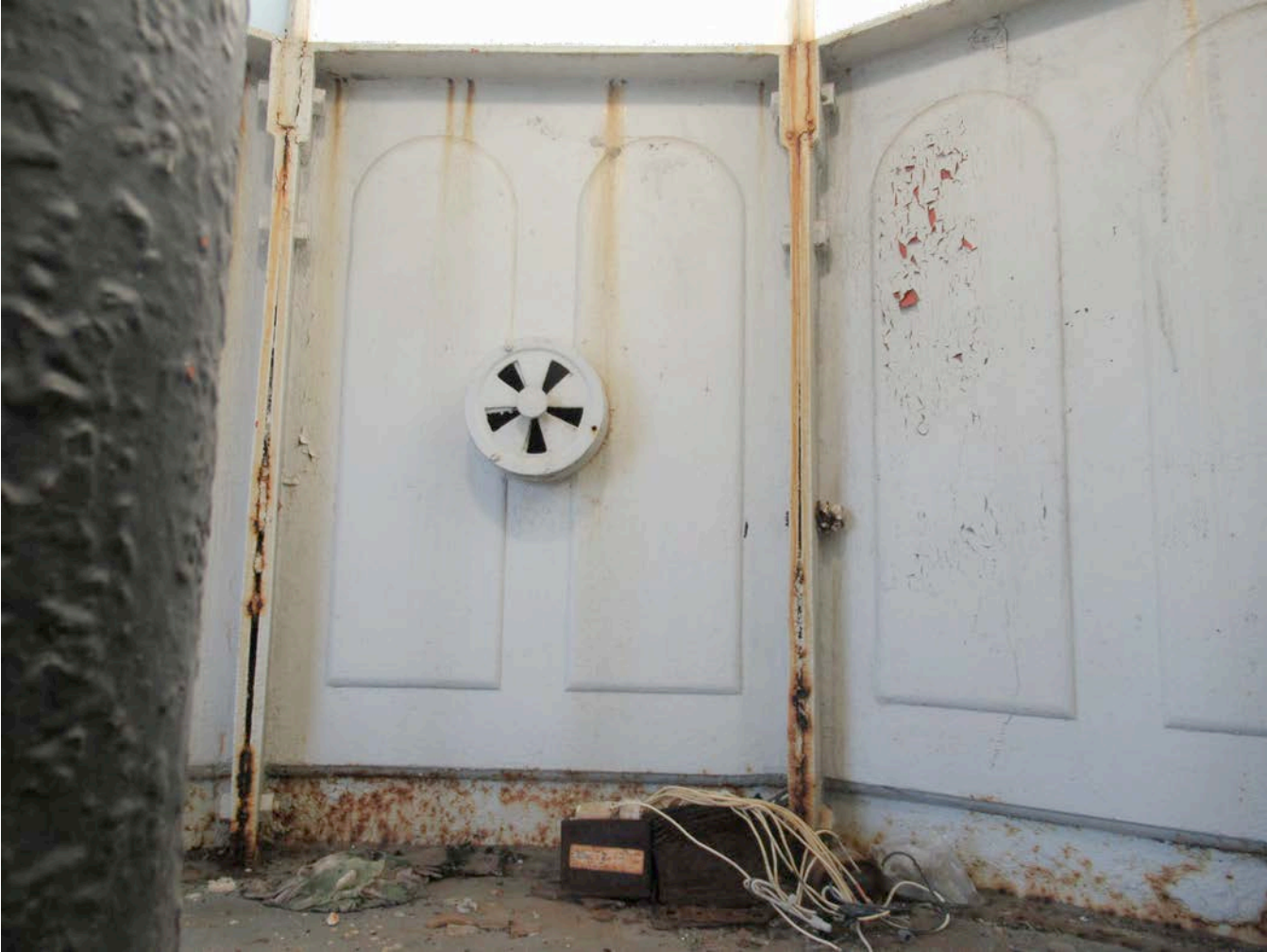
10 PAINT FAILURE & GALVANIC CORROSION LANTERN PARAPET WALL
