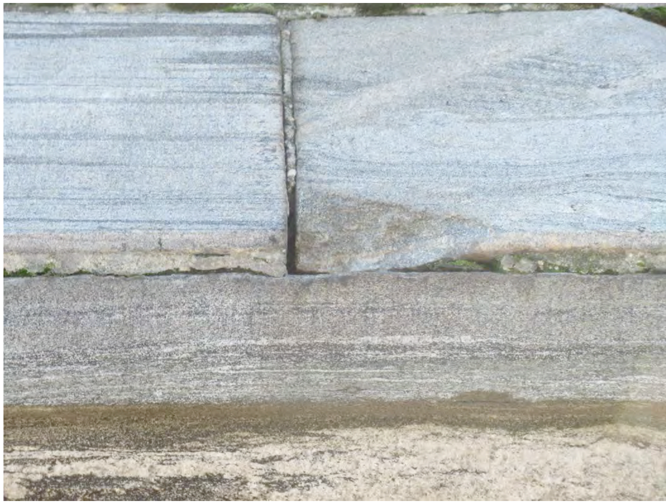
5 STONE SPALL at MOLDING BASE at DISPARATE LOCATIONS
