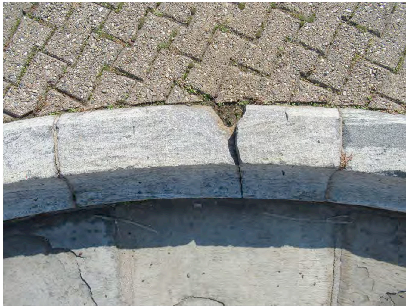
15 CRACK at STONE CURB DEPRESSED PAVED AREA
