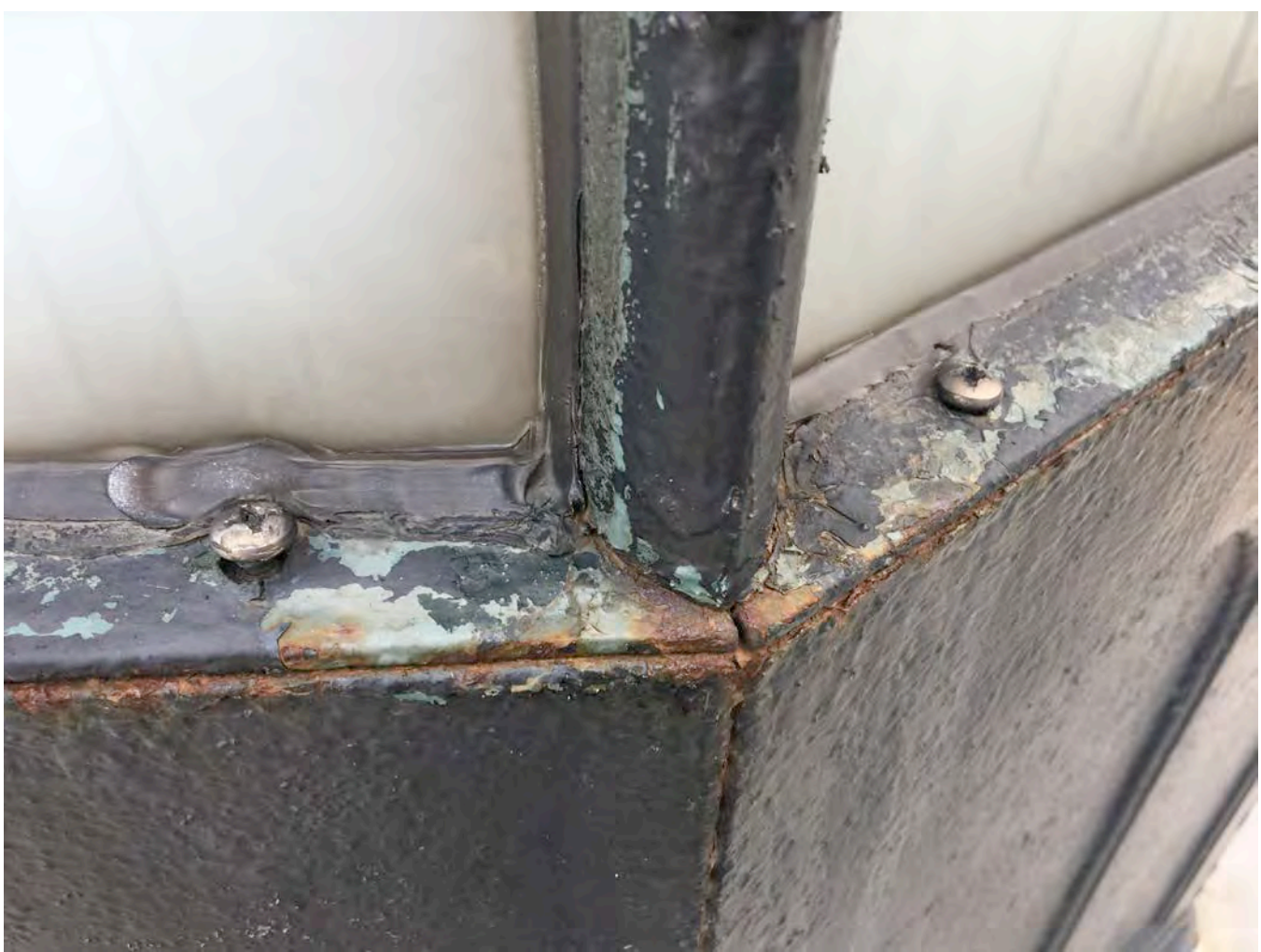
3 PAINT FAILURE, CORROSION OF UNDERLYING METAL & LOOSE FASTENERS LANTERN PARAPET WALL TOP
