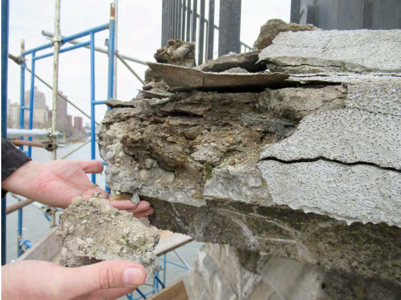
12 SEVERELY CRACKED, SPALLED CONCRETE & DELAMINATED TRAFFIC SURFACE OBSERVATION DECK
