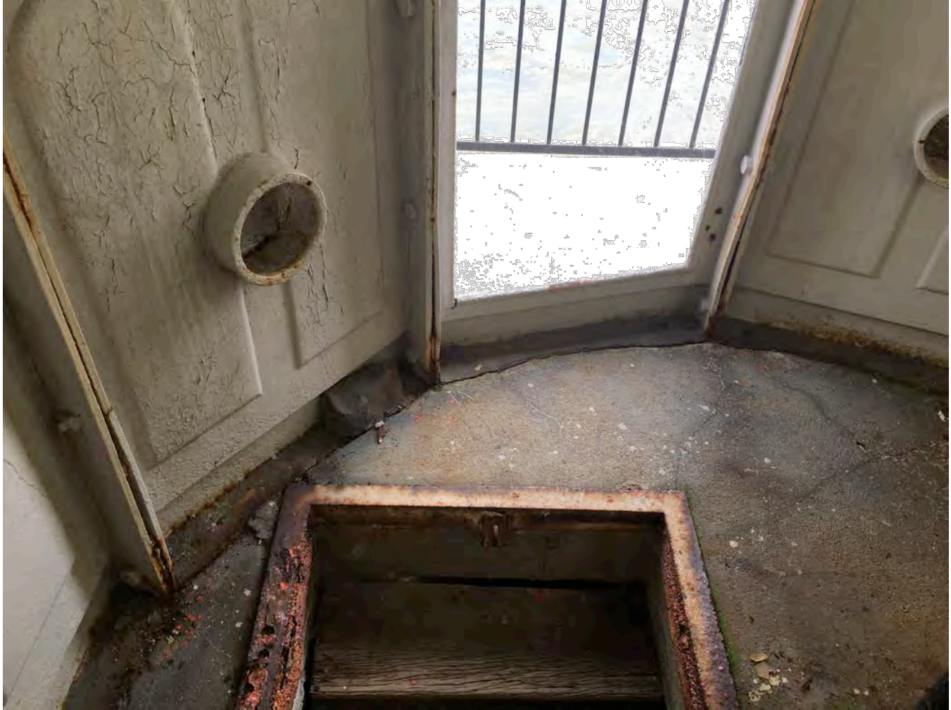
11 PAINT FAILURE, CORROSION OF UNDERLYING METAL & SEPARATION B/N LANTERN & DECK LANTERN PARAPET WALL & OBSERVATION DECK HATCH
