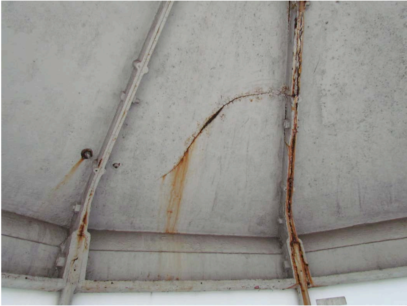
8 CRACKED CAST IRON PANEL, PAINT FAILURE & GALVANIC CORROSION LANTERN ROOF
