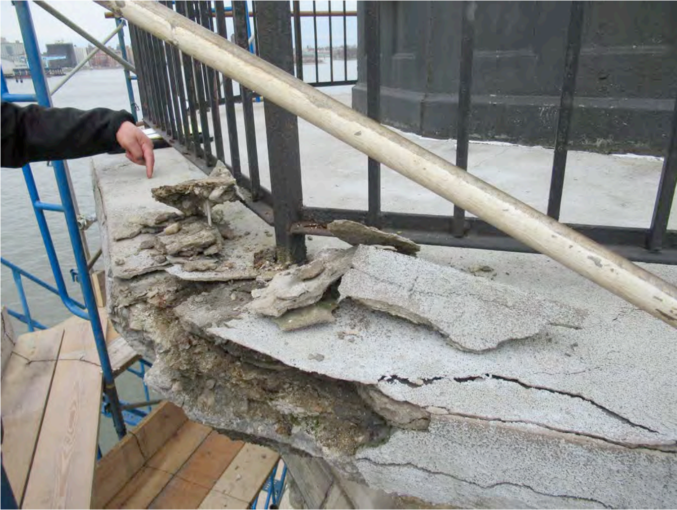
14 SEVERELY CRACKED, SPALLED CONCRETE & DELAMINATED TRAFFIC SURFACE OBSERVATION DECK
