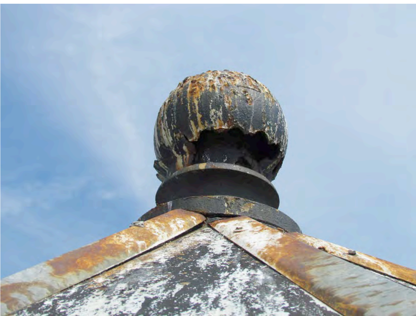
2 FRACTURED CAST IRON VENTILATOR ORB LANTERN ROOF
