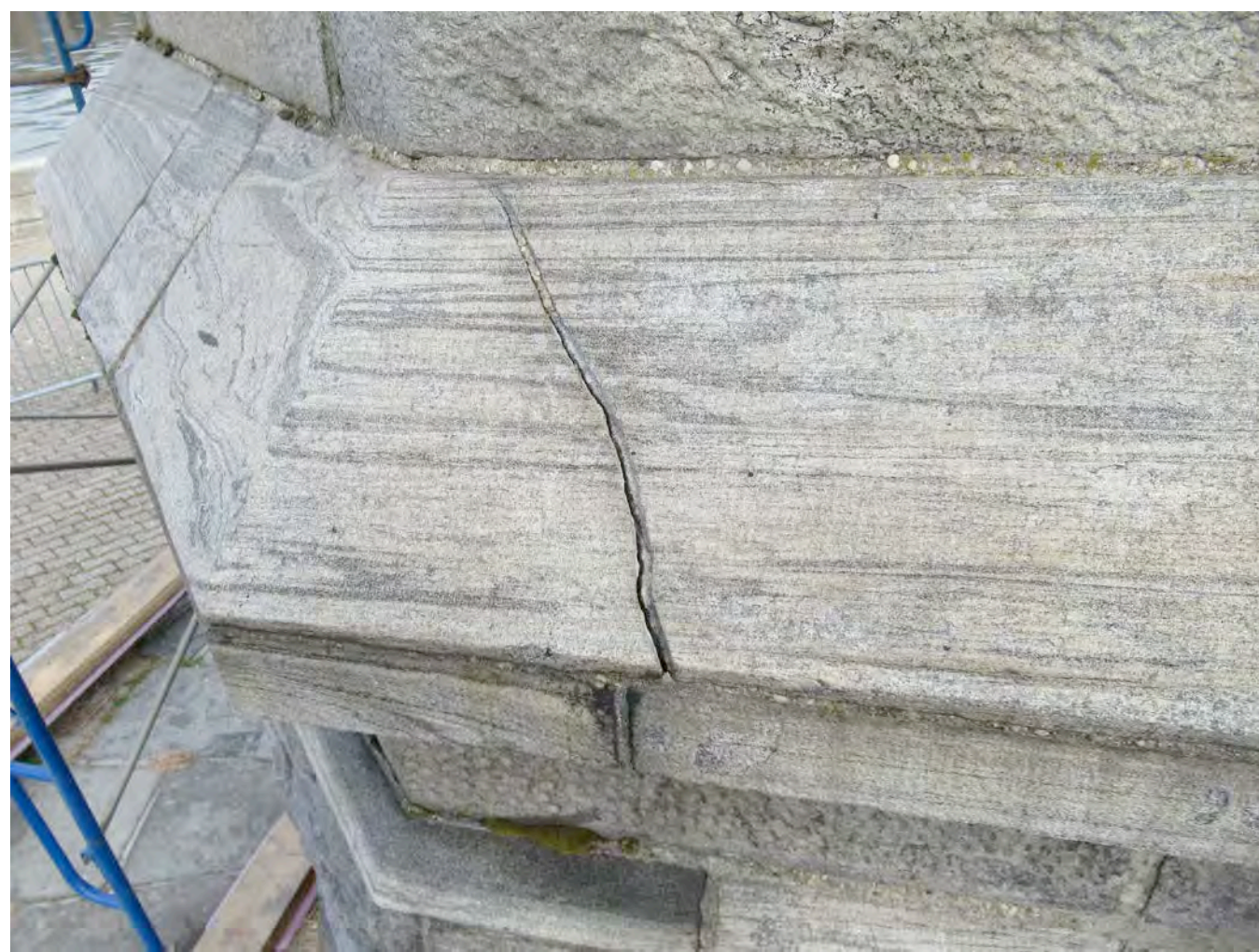
4 STONE CRACKING at MOLDING BASE at DISPARATE LOCATIONS
