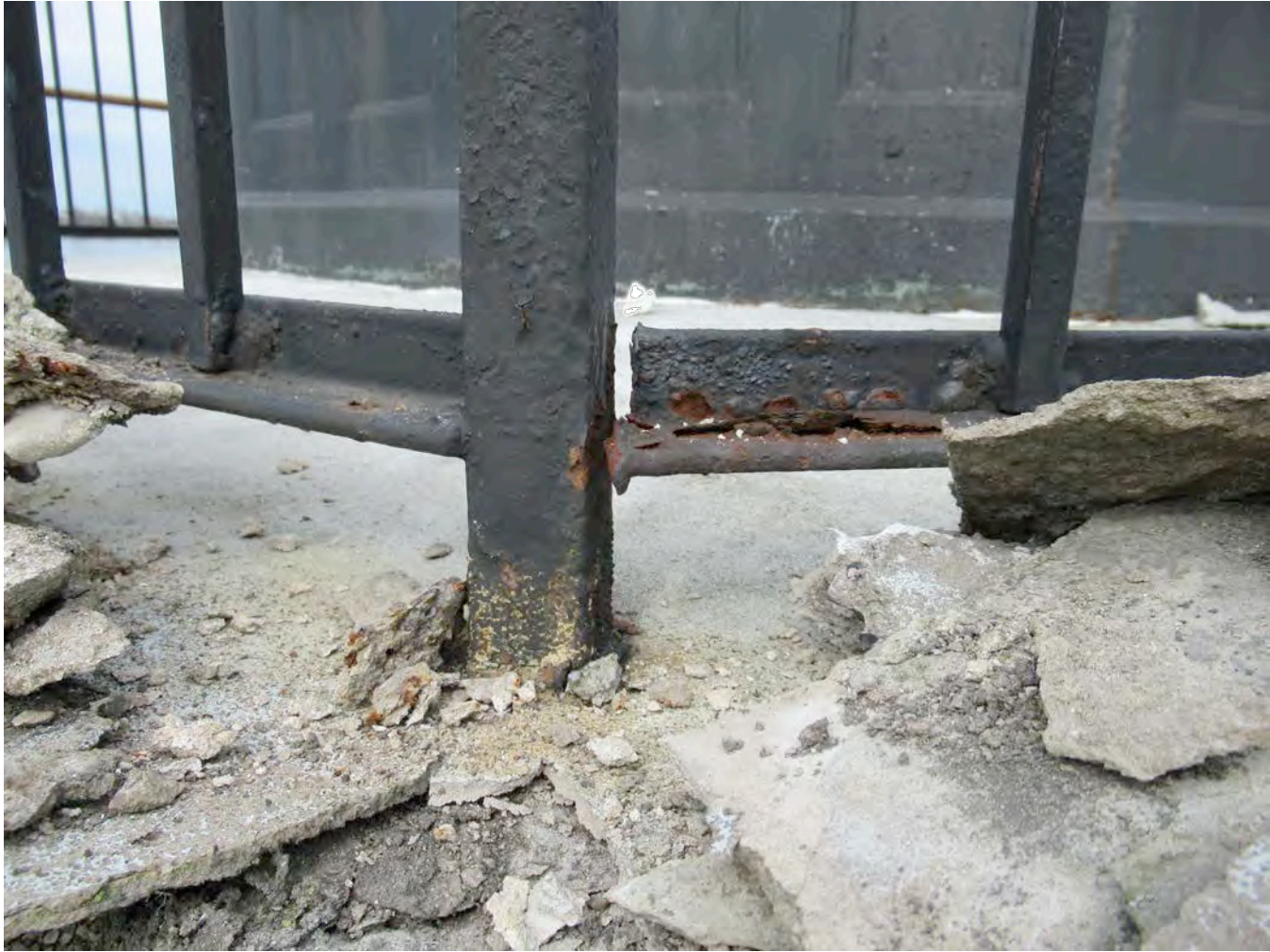
16 PAINT FAILURE, CORROSION OF UNDERLYING METAL & CONNECTION FAILURE METAL RAILING
