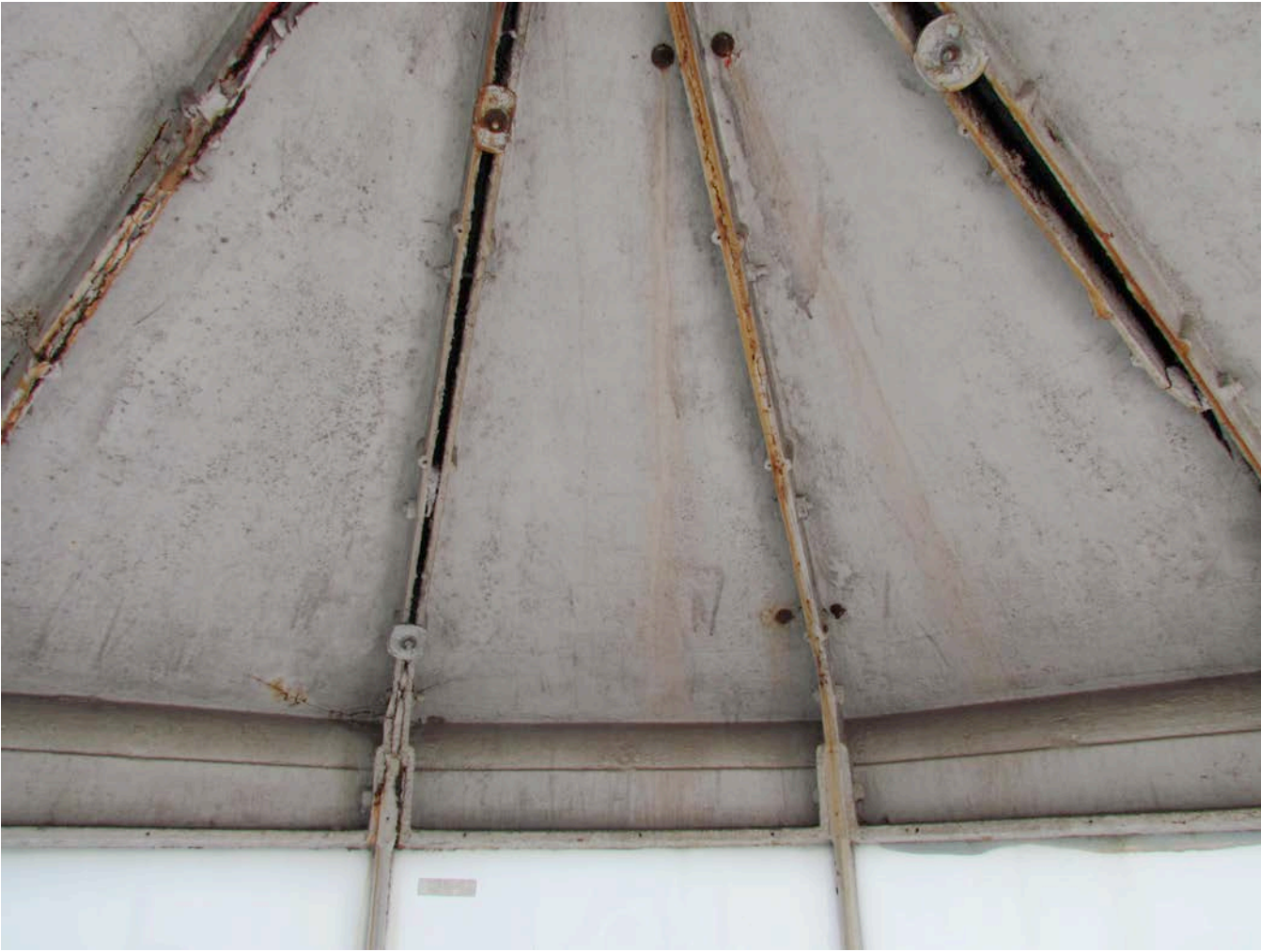
6 CAST IRON PANEL SEPARATION, PAINT FAILURE & GALVANIC CORROSION LANTERN ROOF
