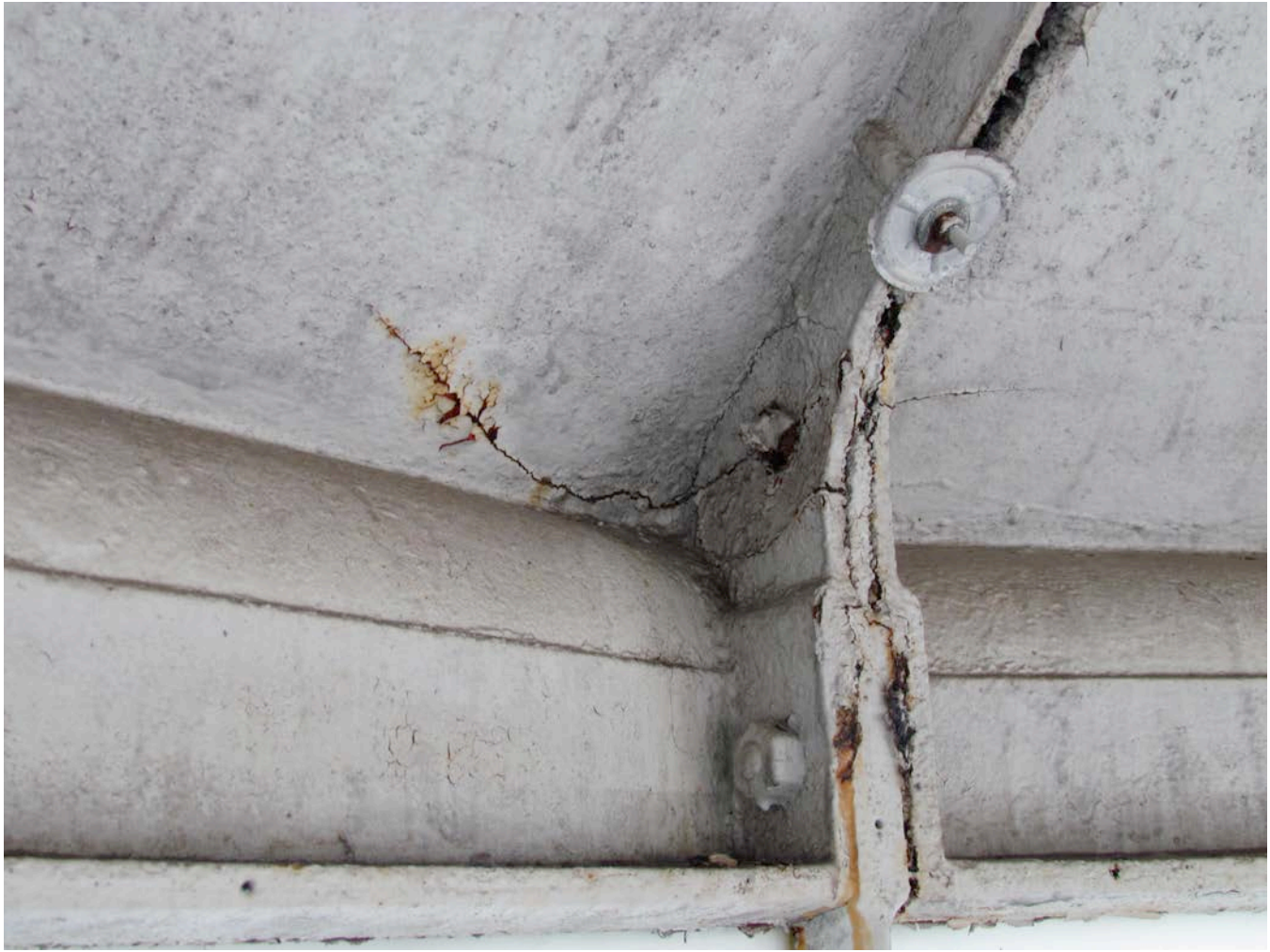
7 CRACKED CAST IRON PANEL, PAINT FAILURE & GALVANIC CORROSION LANTERN ROOF
