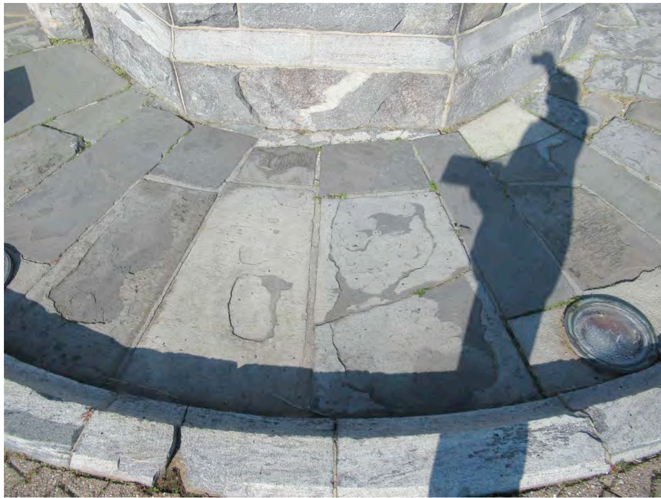
14 DISPLACED, SKEWED, ERODED & SPALLED FLAGSTONES / INCOMPATIBLE PATCHING MATERIAL DEPRESSED PAVED AREA
