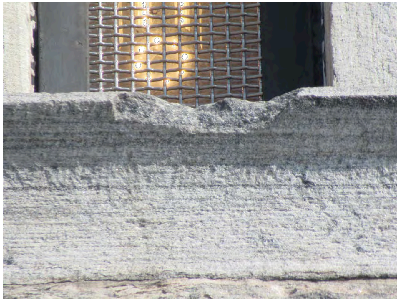
12 STONE SPALL WINDOW SURROUND, TYPICAL CONDITION
