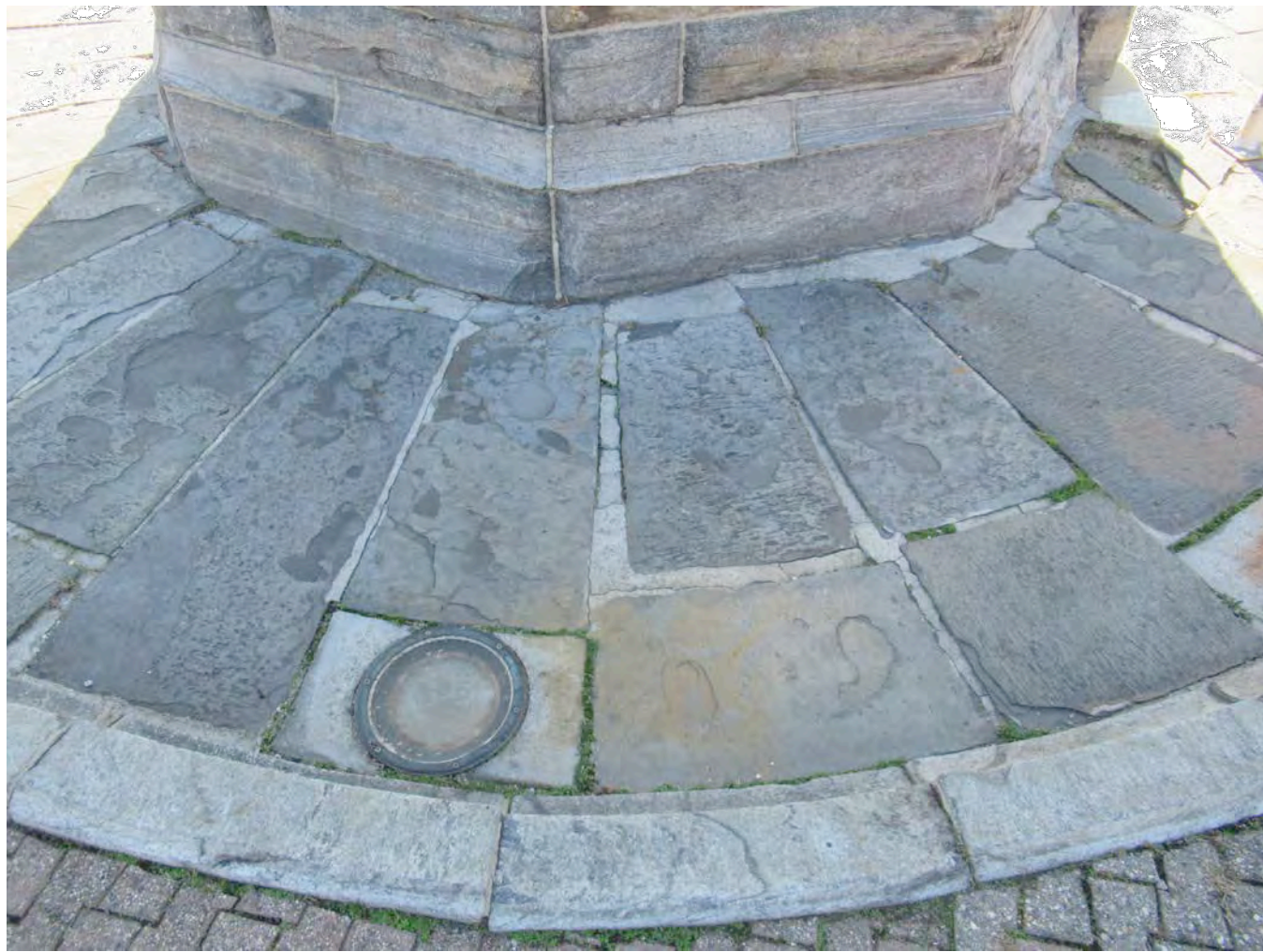
13 DISPLACED, SKEWED, ERODED & SPALLED FLAGSTONES / INCOMPATIBLE PATCHING MATERIAL DEPRESSED PAVED AREA
