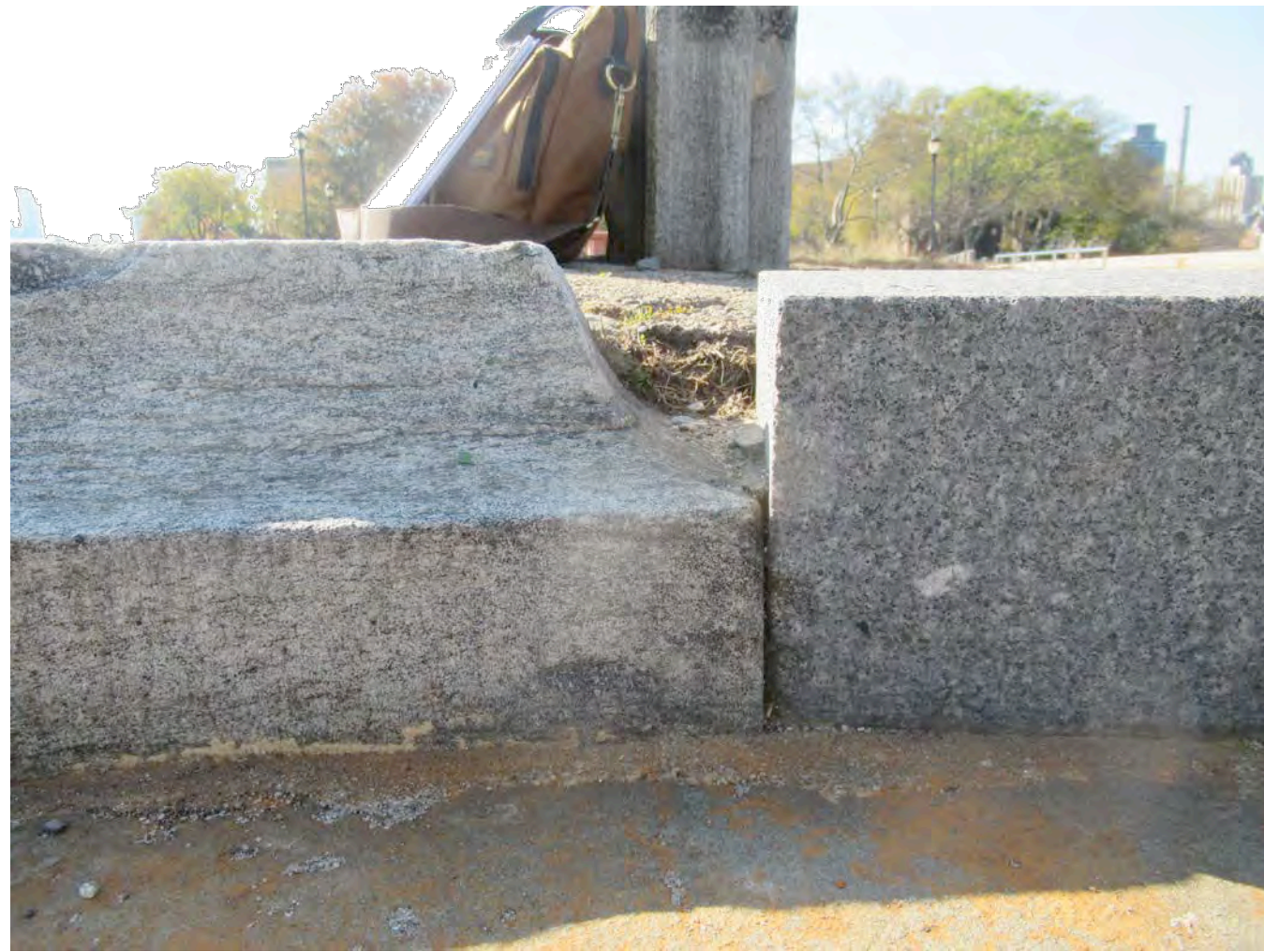
16 DETAIL VIEW OF STONE CURB END UNIT w/ NON-ORIGINAL STONE STEP at RIGHT DEPRESSED PAVED AREA
