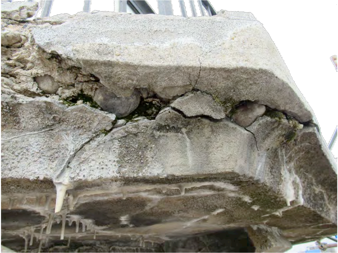
15 DETERIORATED MASONRY MORTAR JOINTS OBSERVATION DECK
