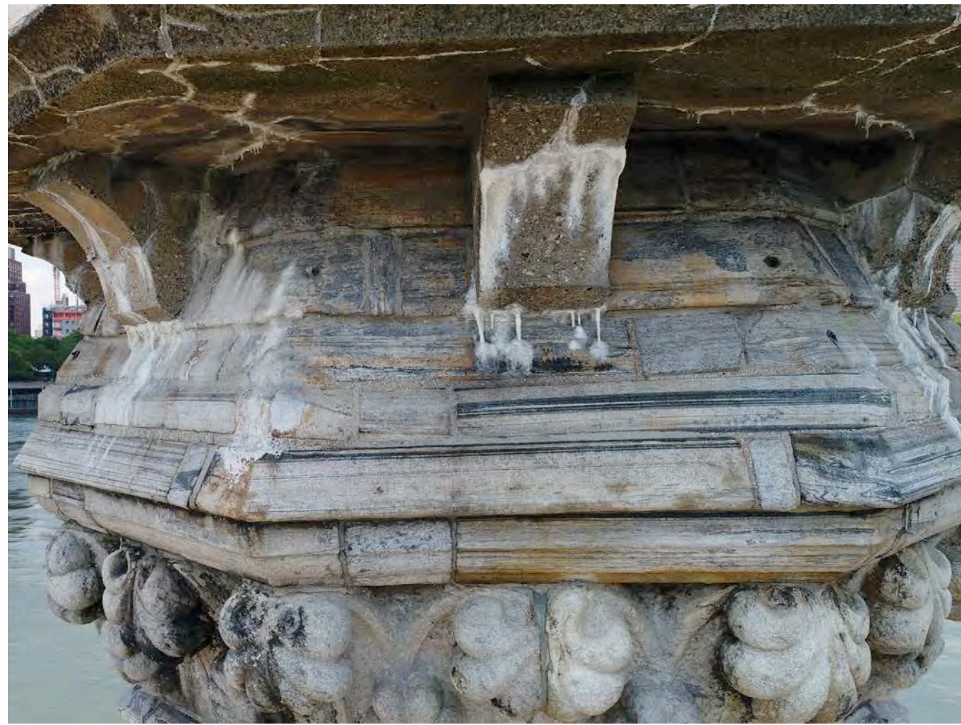
8 REMNANT OF METAL BRACKET ANCHORAGE STEPPED STONE PROFILE at CAPITAL, EACH OUTSIDE CORNER OF THE OCTAGONAL TOWER
