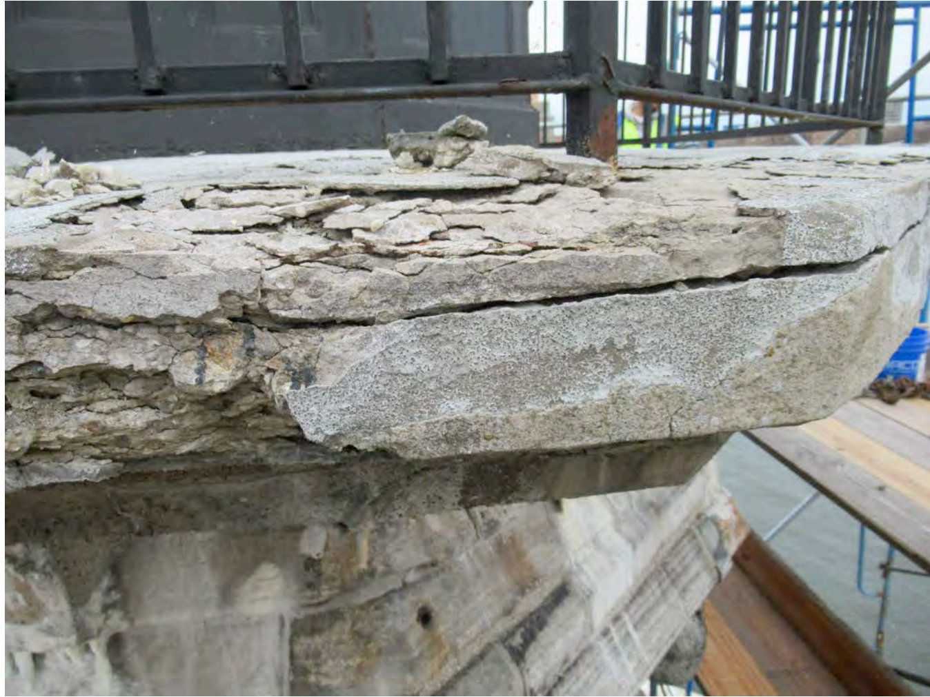
13 SEVERELY CRACKED, SPALLED CONCRETE & DELAMINATED TRAFFIC SURFACE OBSERVATION DECK
