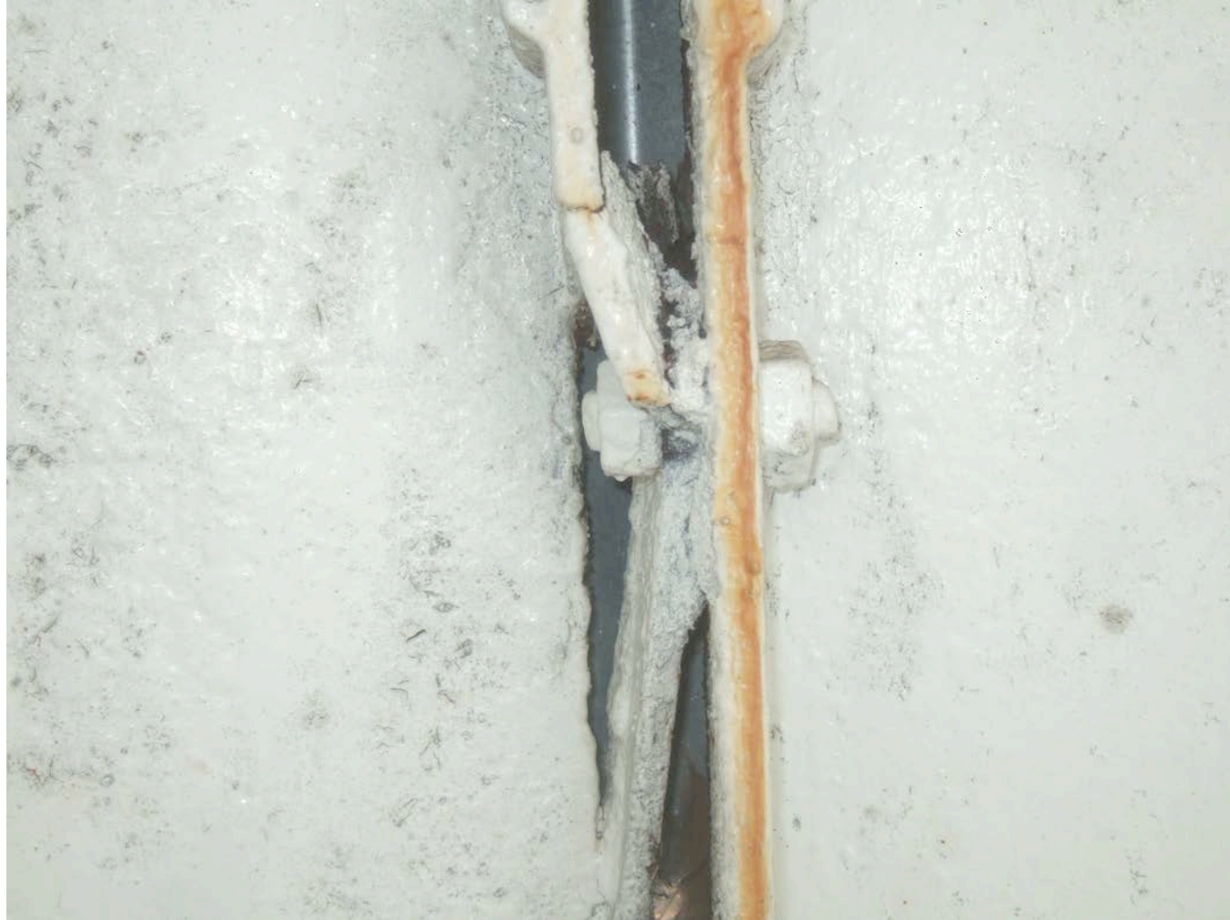
9 CAST IRON PANEL SEPARATION & DEFORMATION LANTERN ROOF
