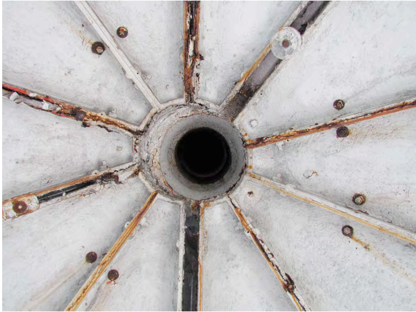
5 CAST IRON PANEL SEPARATION, PAINT FAILURE & GALVANIC CORROSION LANTERN ROOF
