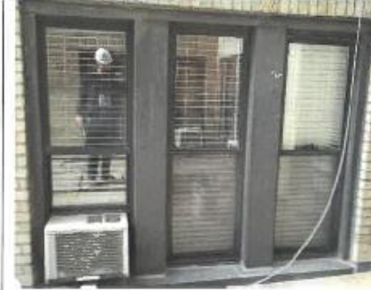
Typical Ganged (triple) window
