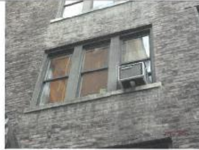
Ganged Windows (triple equal width)
