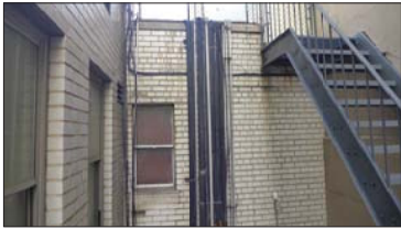
PHOTO OF EXISTING WEST ELEVATION
