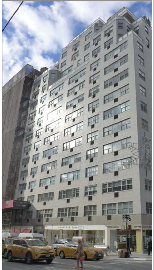
PHOTO OF EXISTING EAST ELEVATION (W/ADJACENT BUILDING)
