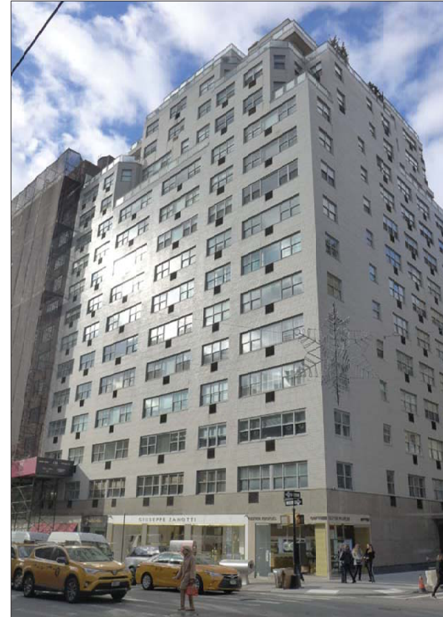
PHOTO OF NORTHEAST CORNER OF 20 EAST 68TH STREET
