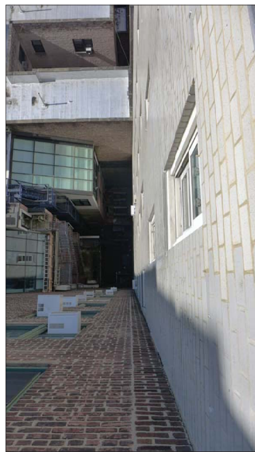
PHOTO OF EXISTING SOUTH ELEVATION
