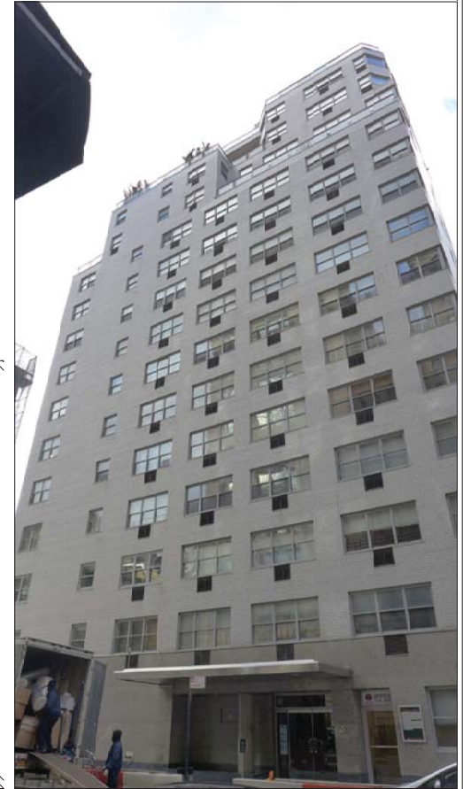
PHOTO OF EXISTING NORTH ELEVATION 300' WEST STREET
