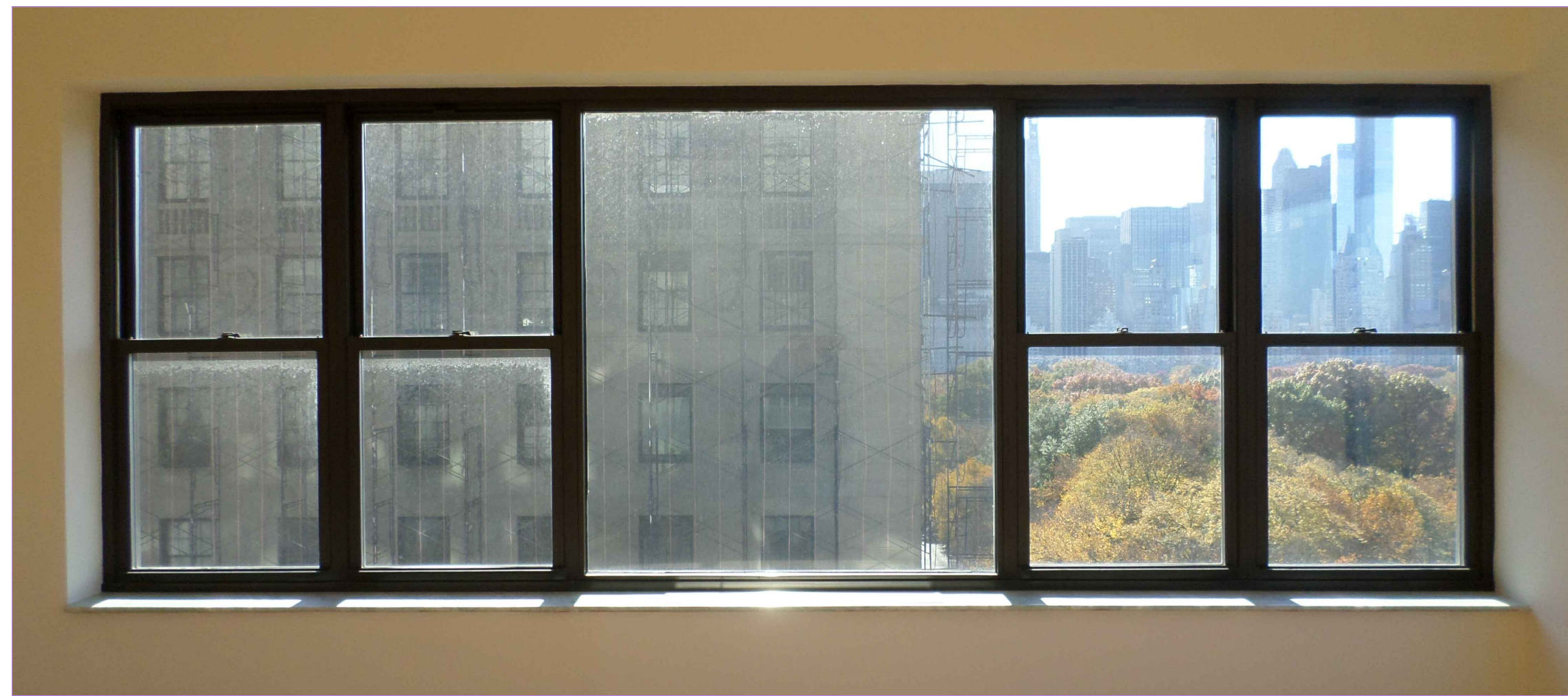
Existing Window Opening '1' - Interior View N.T.S. (South Facade)
