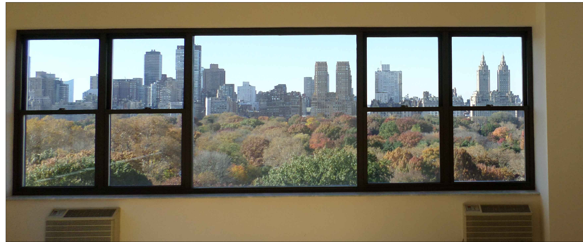
Existing Window Opening '1' - Interior View N.T.S. (West Facade)
