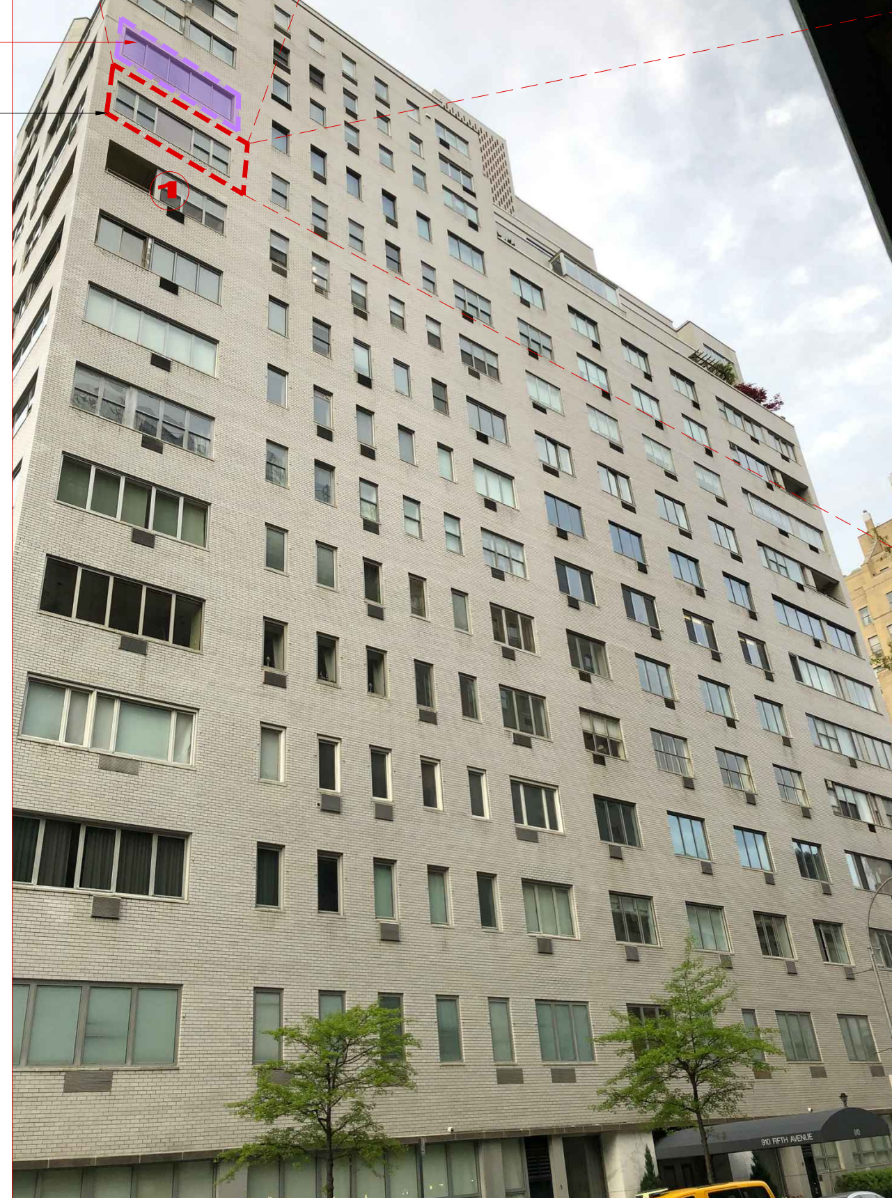
910 Fifth Avenue Apt. 11A - Existing South Facade N.T.S.
