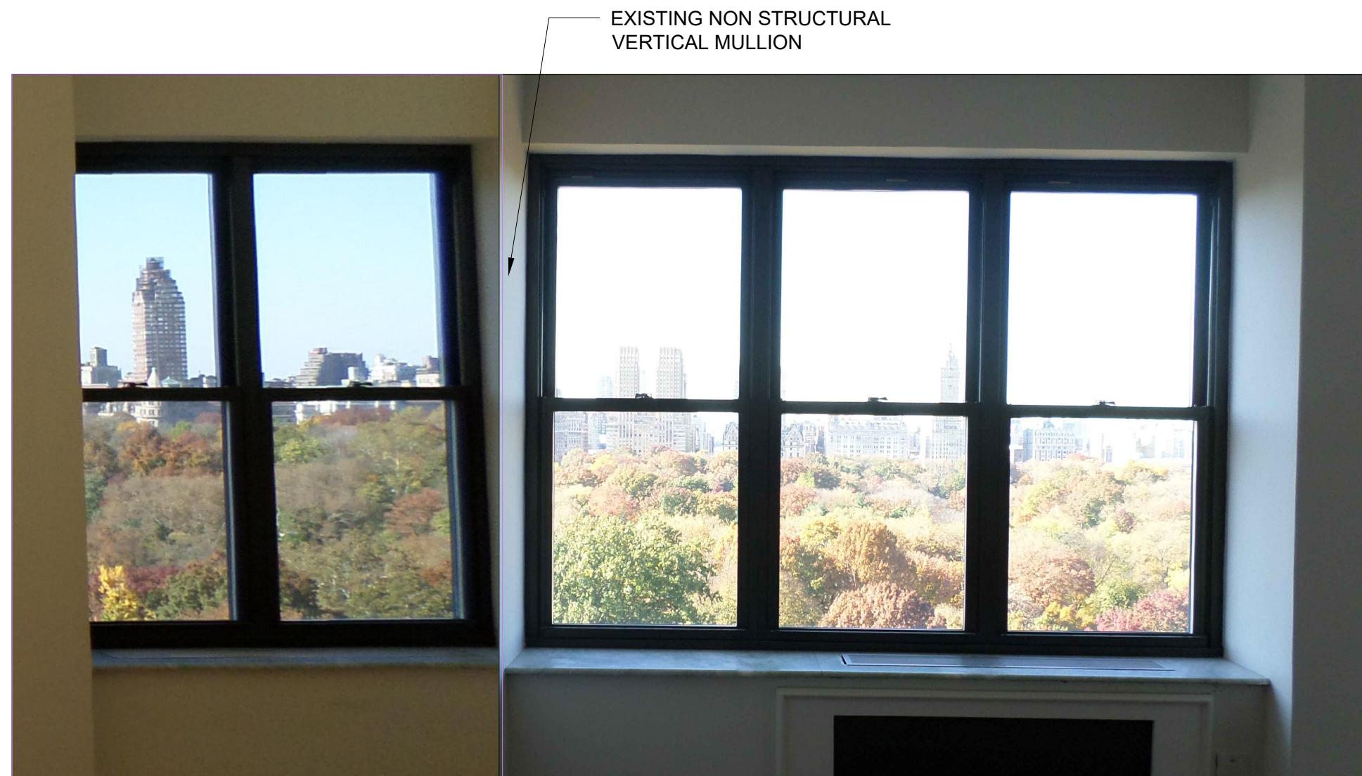
Existing Window Opening '1' - Interior View N.T.S. (West Facade)
