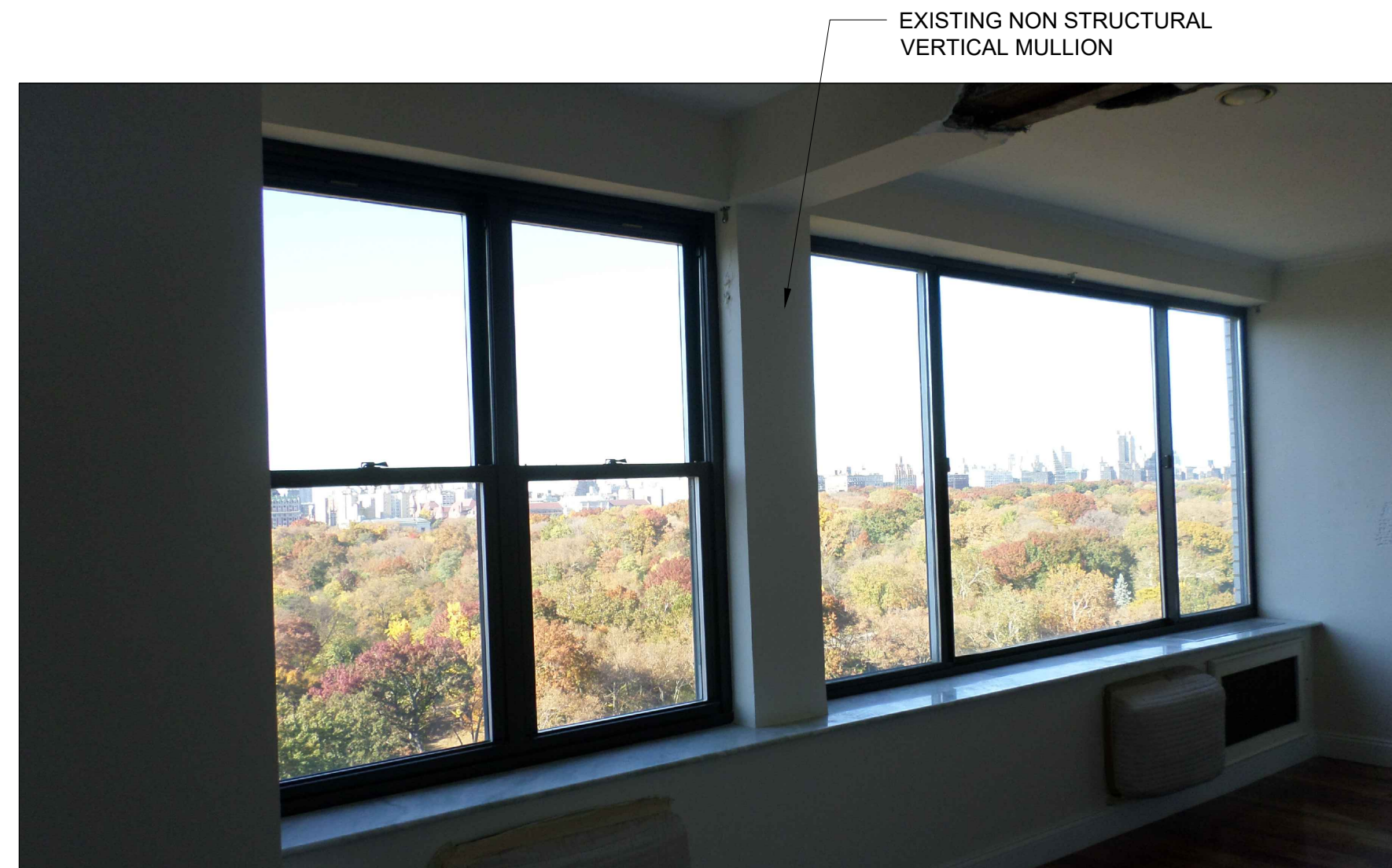
Existing Window Opening '1' - Interior View N.T.S. (West Facade)
