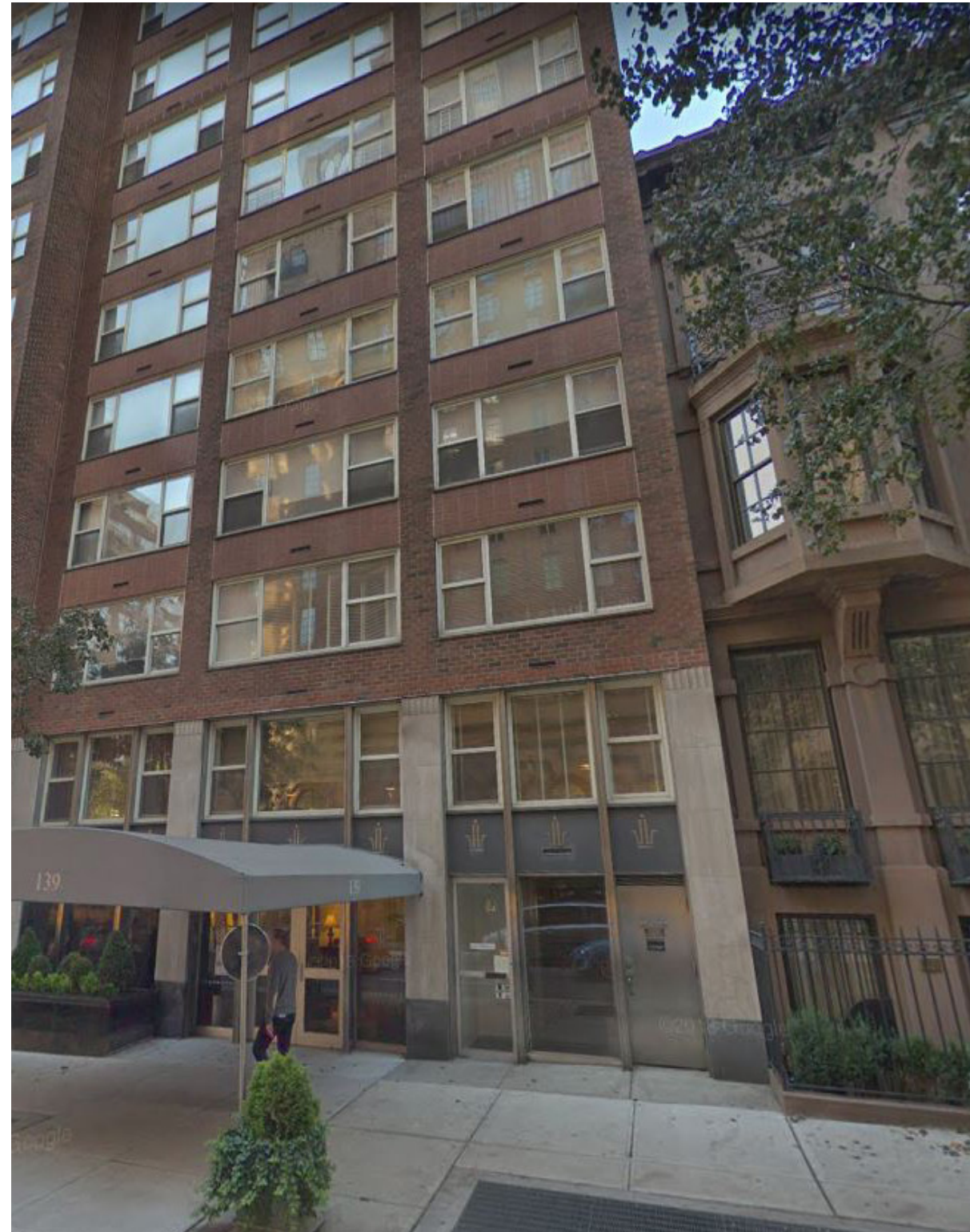
ADJACENT BUILDING FROM 63RD ST.
