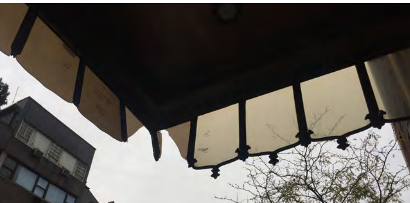
DETAIL PHOTOS: EXISTING DAMAGE TO MARQUEE ON MADISON AVE.
