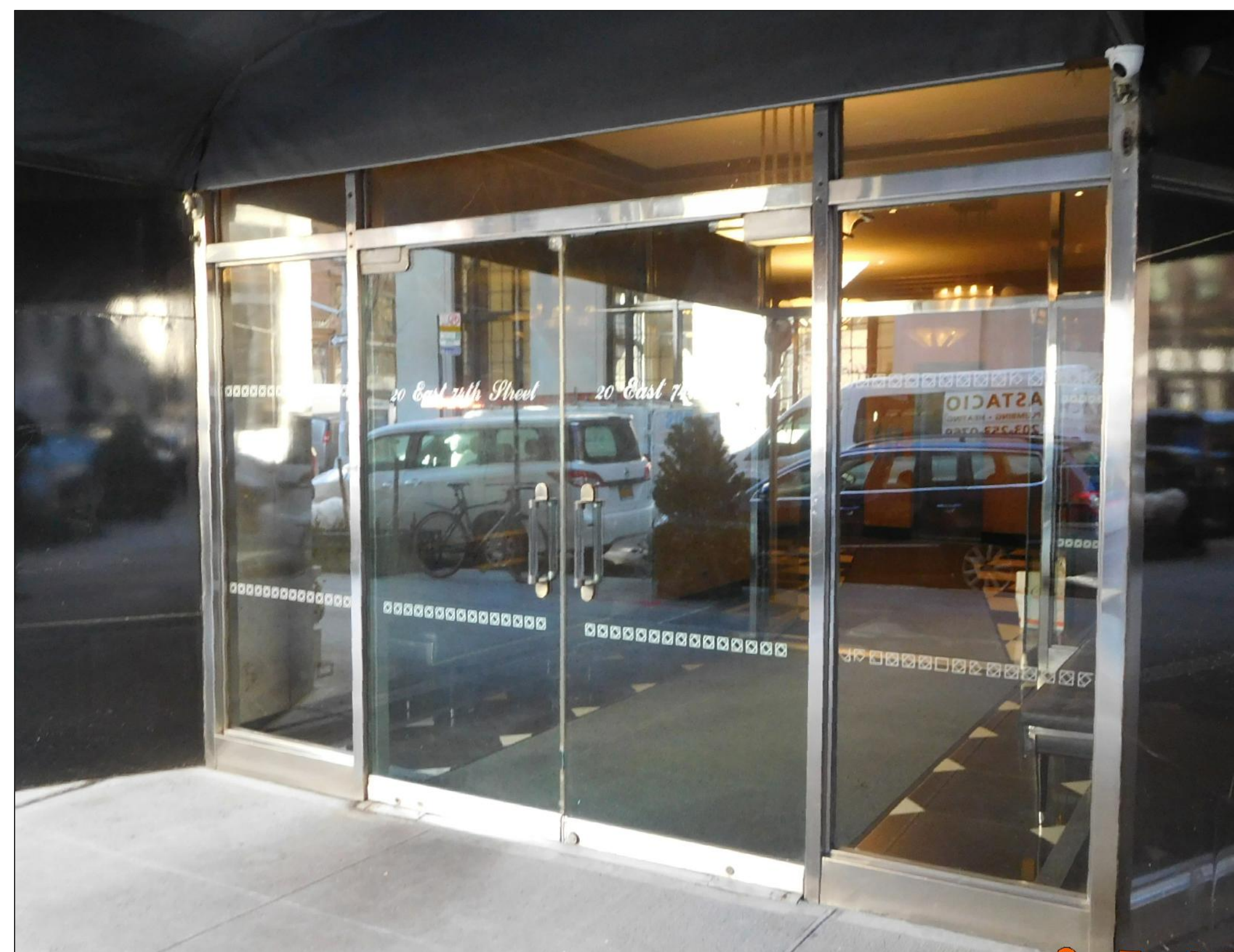
2.1 PHOTO OF EXISTING BUILDING ENTRANCE
