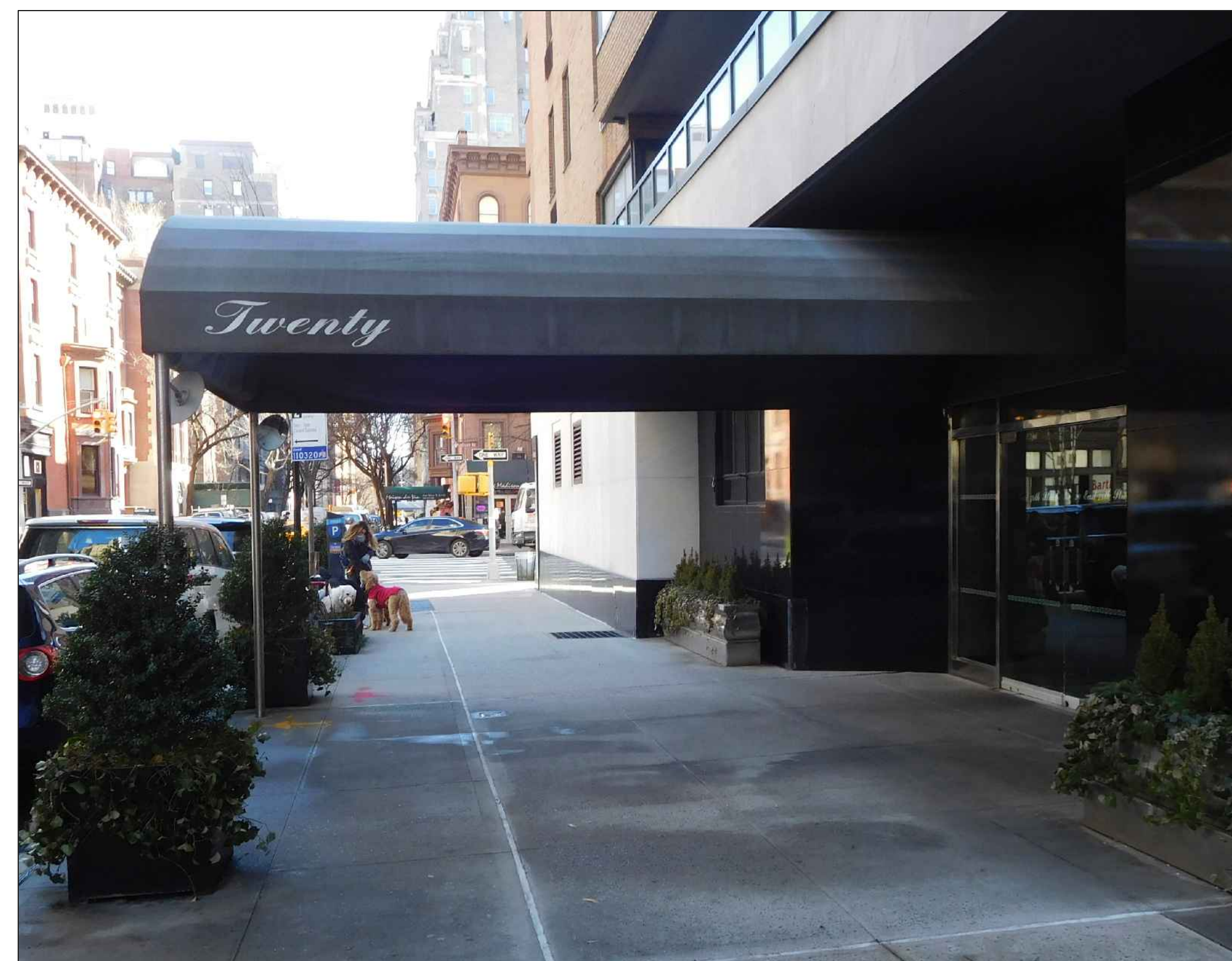
1.2 PHOTO OF ENTRANCE, LOOKING EAST TO MADISON AVENUE
