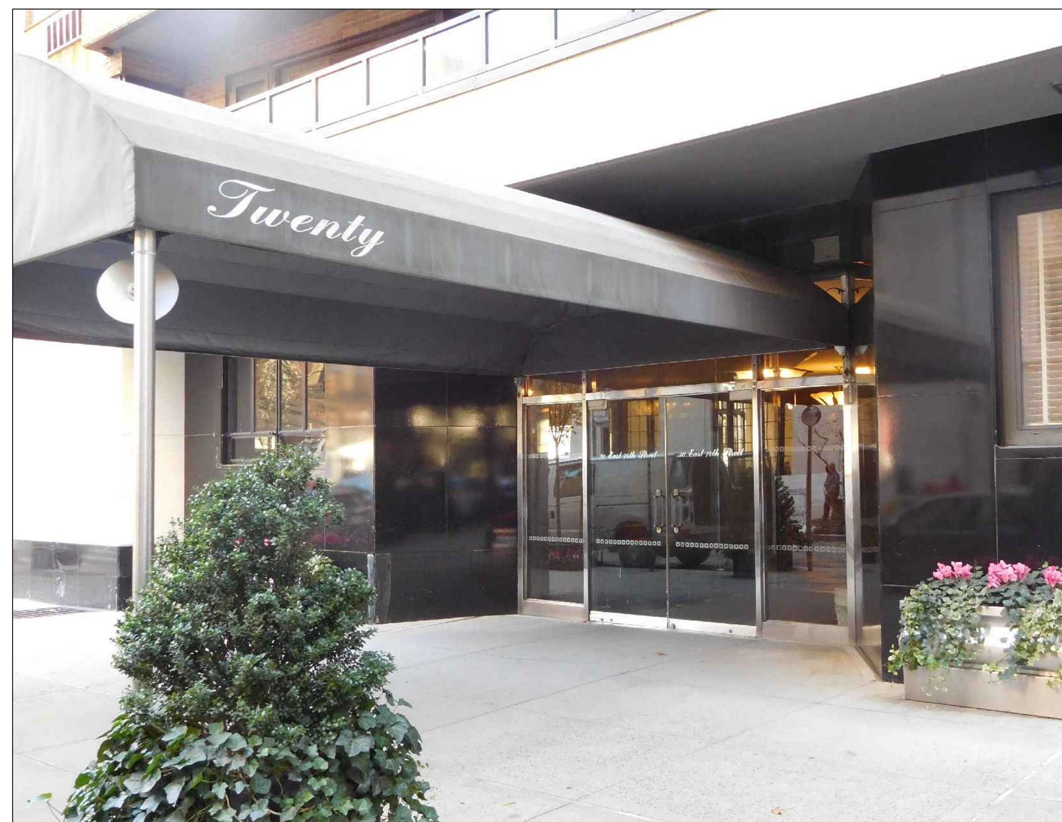
1.1 PHOTO OF EXISTING BUILDING ENTRANCE & AWNING
