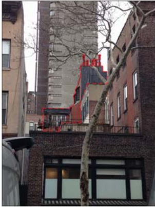
6. VIEW OF PARTIAL SOUTH AND EAST FACADE FROM LEXINGTON AVENUE
