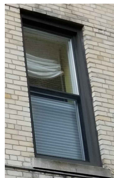
EXISTING WINDOW (E1)
