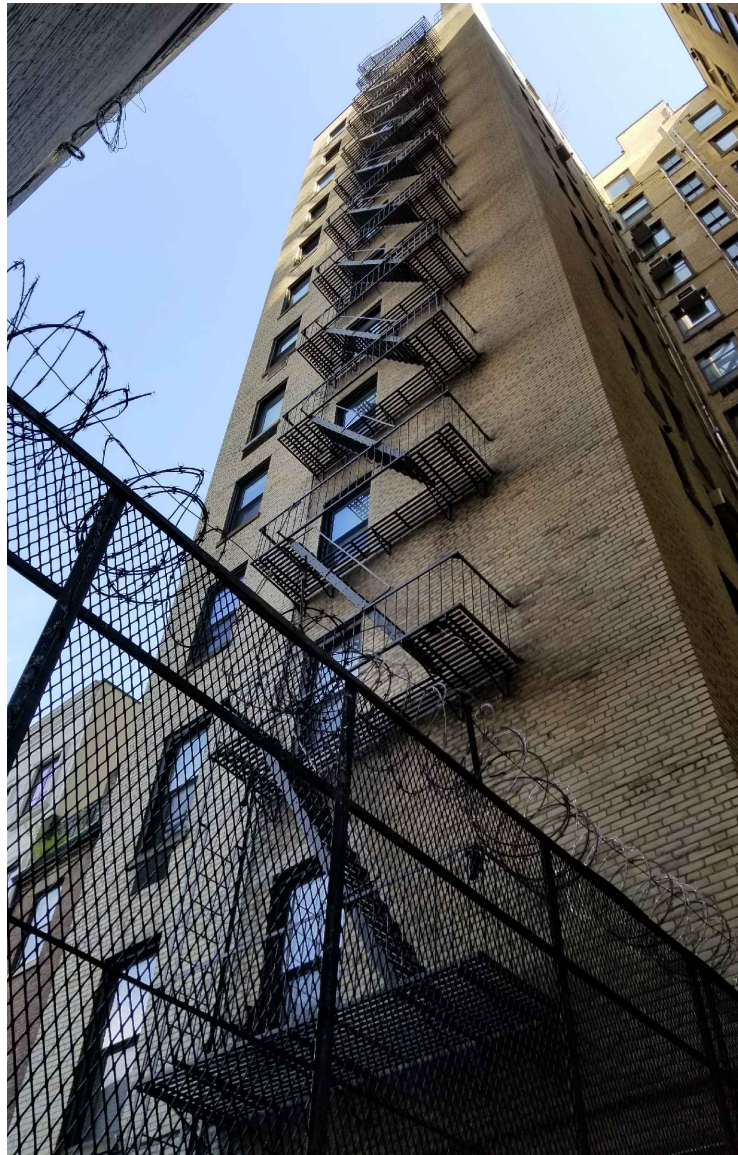
4 Existing Building - South Facade (Inner Courtyard)
