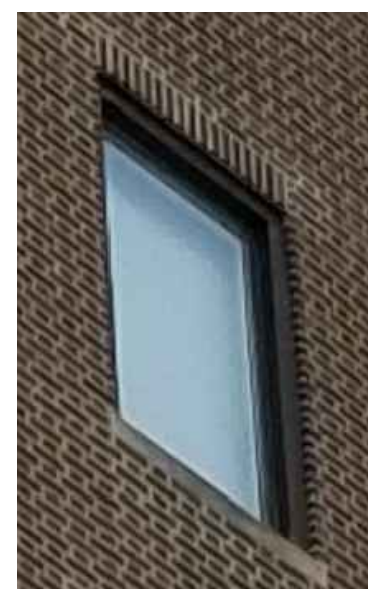
EXISTING WINDOW (E3)
