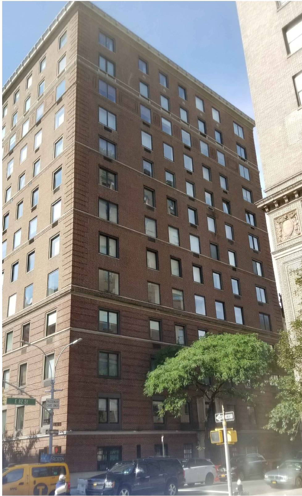
2 Existing Building - North Facade (From Park Avenue & 82nd Street Corner)
