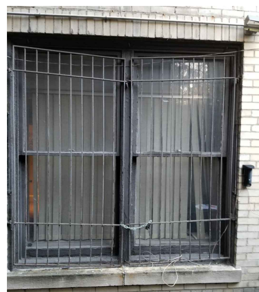
EXISTING WINDOW (E2)
