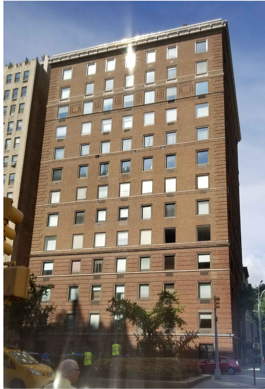
3 Existing Building - East Facade (From Park Avenue)
