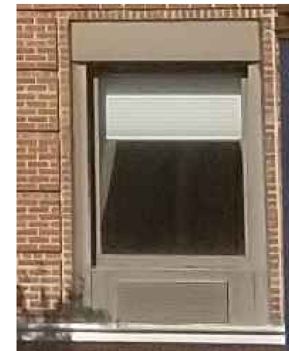
EXISTING WINDOW E5
