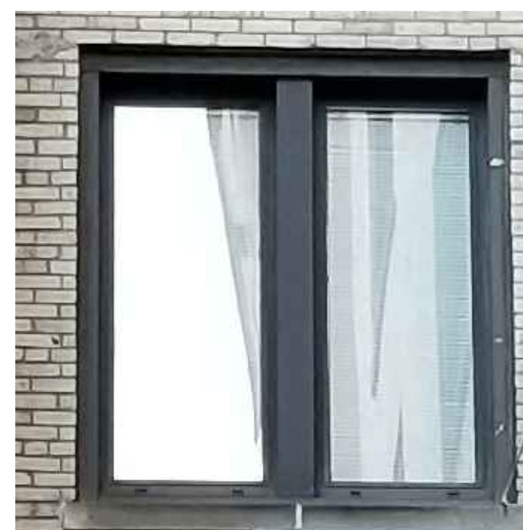
EXISTING WINDOW (E4)
