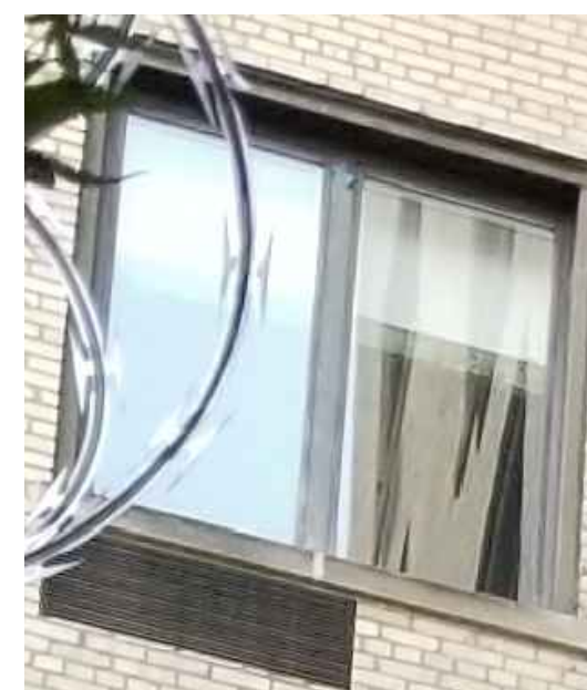
EXISTING WINDOW E4
