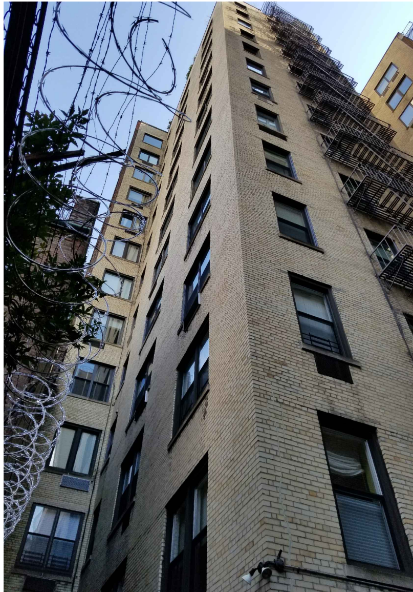
5 Existing Building - South / West Facade (Inner Courtyard)
