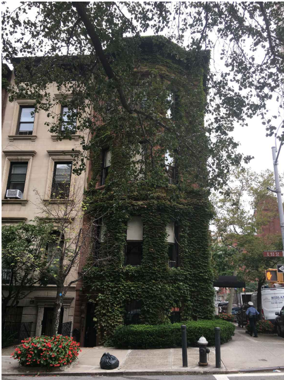
2 EXISTING PHOTO - EAST 93RD STREET FACADE
