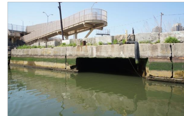
Combined sewer outfall located on Harlem River
