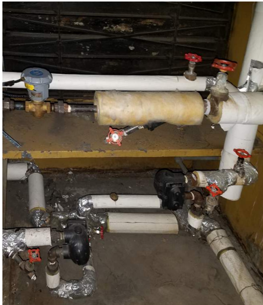
PIPING AND FITTINGS FAILING
