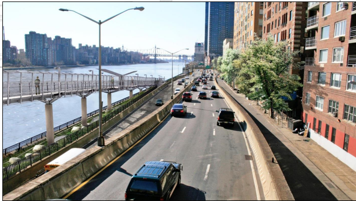
Install New Bridge and Ramp
