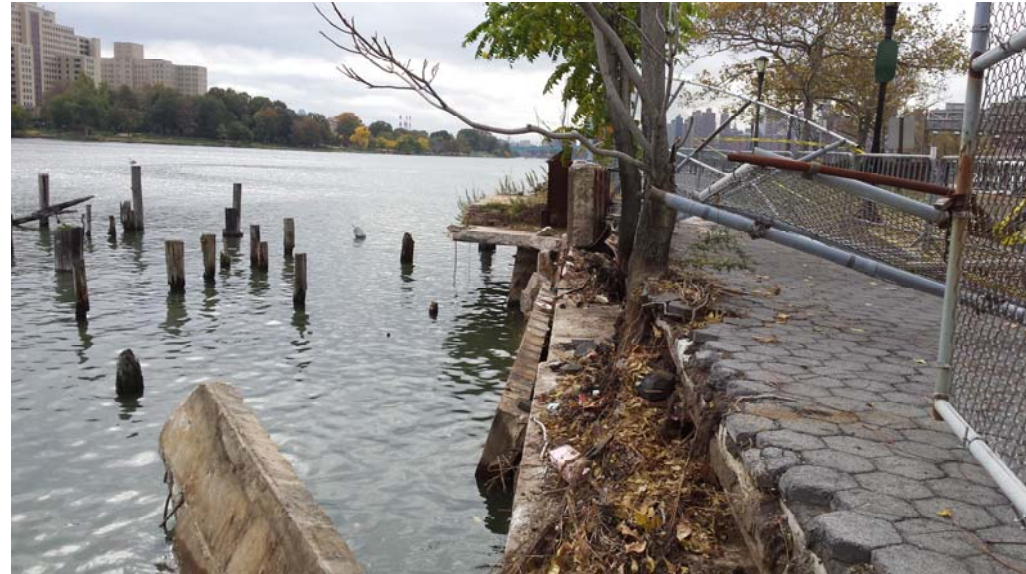
Partial collapse and loss of bulkhead
