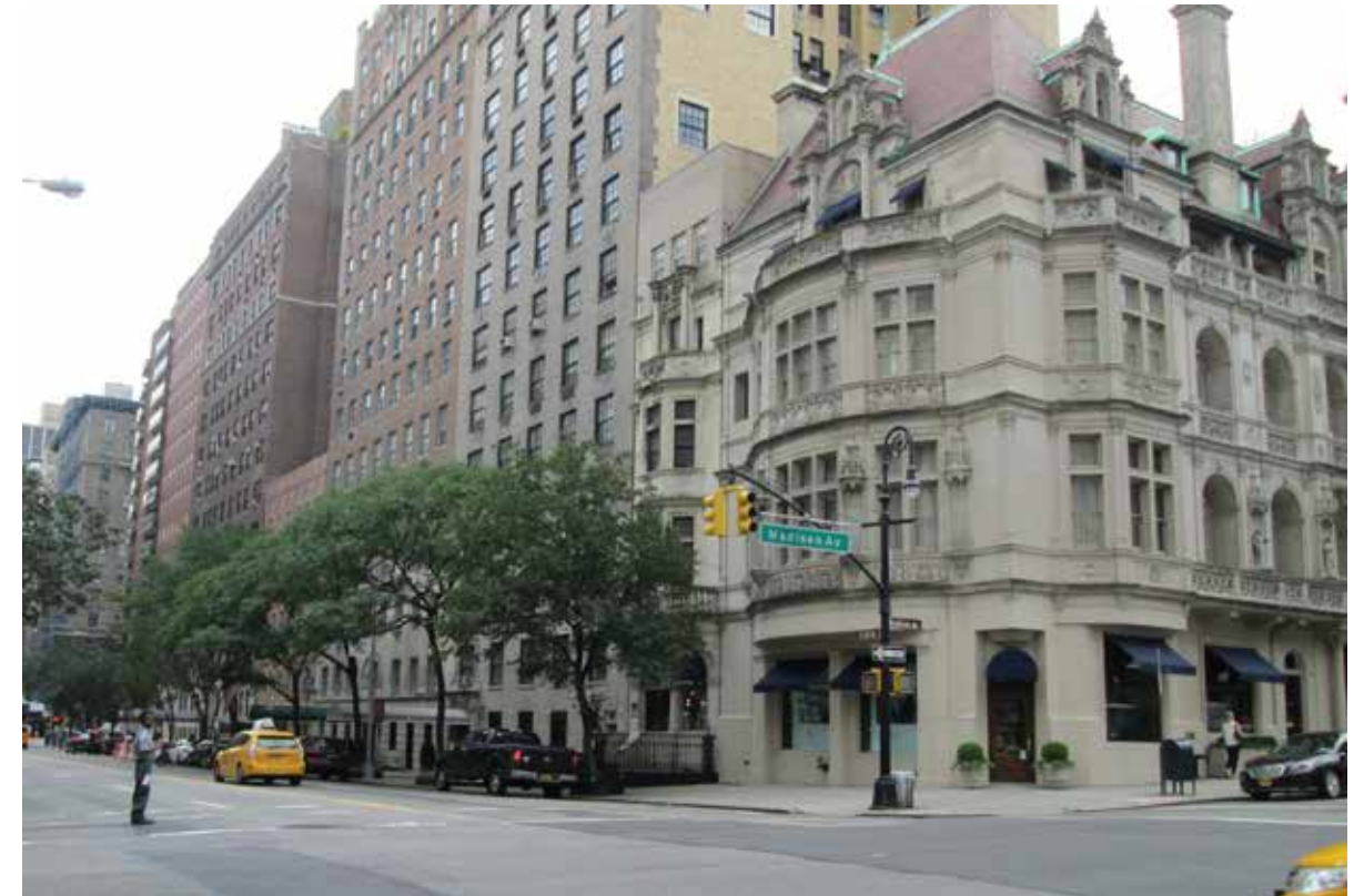
SOUTHEAST CORNER - RHINELANDER MANSION
