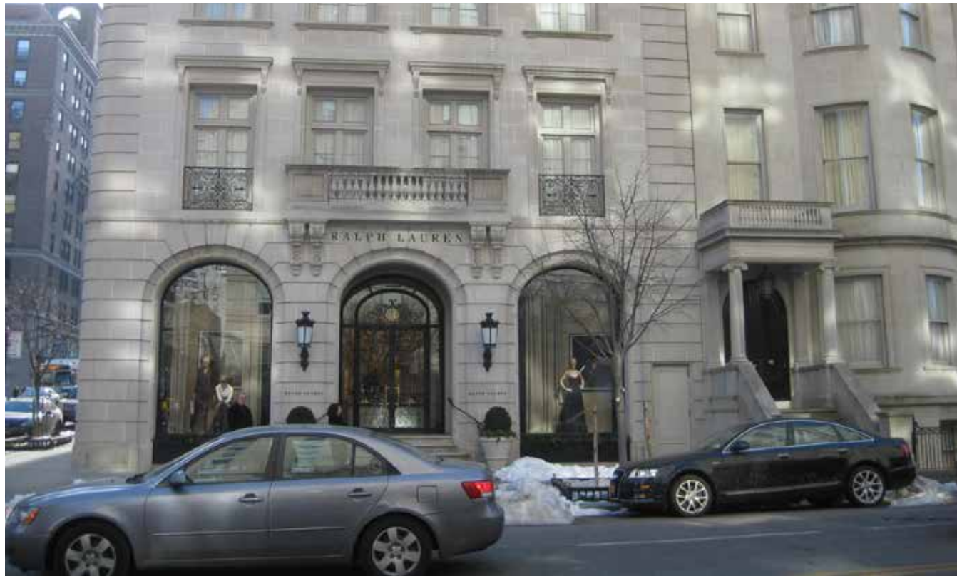
SOUTHWEST CORNER - RALPH LAUREN
