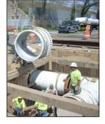
coating in the factory. The interior of the pipe is factory coated with a concrete lining.
