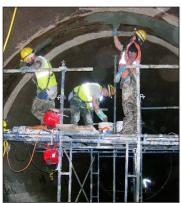
The South Connecting Conduit, put into service in the 1930s, is a critical component of the operational system at Hillview. It provides a hydraulic balance between reservoir storage and tunnel demand. It is a 736-foot-long, 14'6"-diameter reinforced concrete conduit. Since redundancy is built into the system, other infrastructure was used while the South Connecting Conduit was being repaired.
