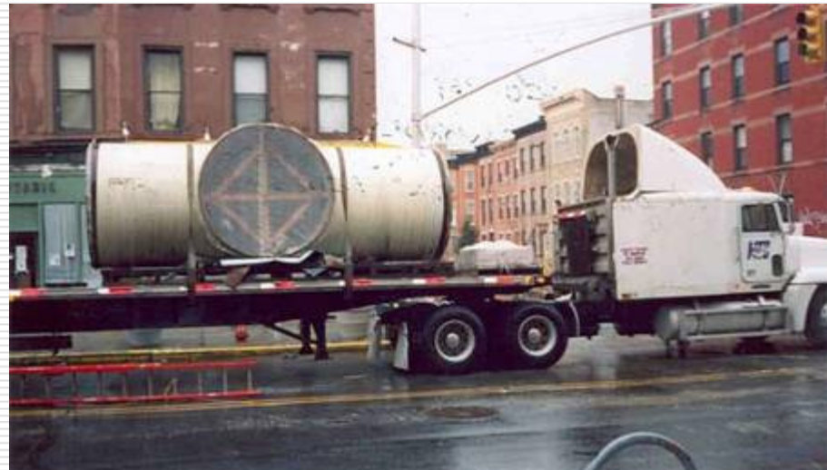
TRUNK WATER MAIN BEING DELIVERED TO SITE
