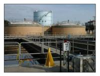
gas is flared through a burner. Unlike the 1950s, when sewage sludge was just dumped in the ocean, DEP vessels now pick up Rockaway's digested sludge and take it to a dewatering facility for further processing and finally land application.
