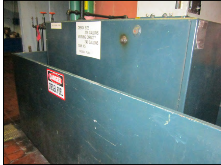
Photograph 6. A 275-gallon diesel aboveground storage tank (AST) in the Hospital Building west-adjacent to the eastern portion of the Property.
