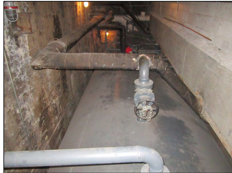
Photograph 8. An 18,500-gallon fuel oil AST in the Power House, west of the Property.
