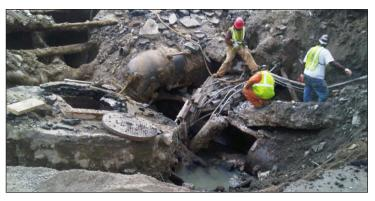
**REPAIR AND RESTORE:** Site of Jerome Avenue 36-inch water main break after the water was pumped out. Beneath New York City streets is a maze of water, sewer, electrical and gas pipes.
