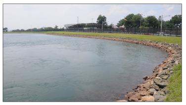
a reserve tank to supply the three city water tunnels with the water they need to meet the day's demand. And as demand decreases during the night, water from the upstate aqueducts refills the depleted reservoir to ensure that it is fully stocked for the next morning. As a result, reservoir levels are constantly fluctuating.
