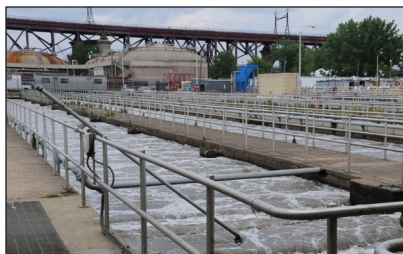
Aeration tanks at the Wards Island plant
