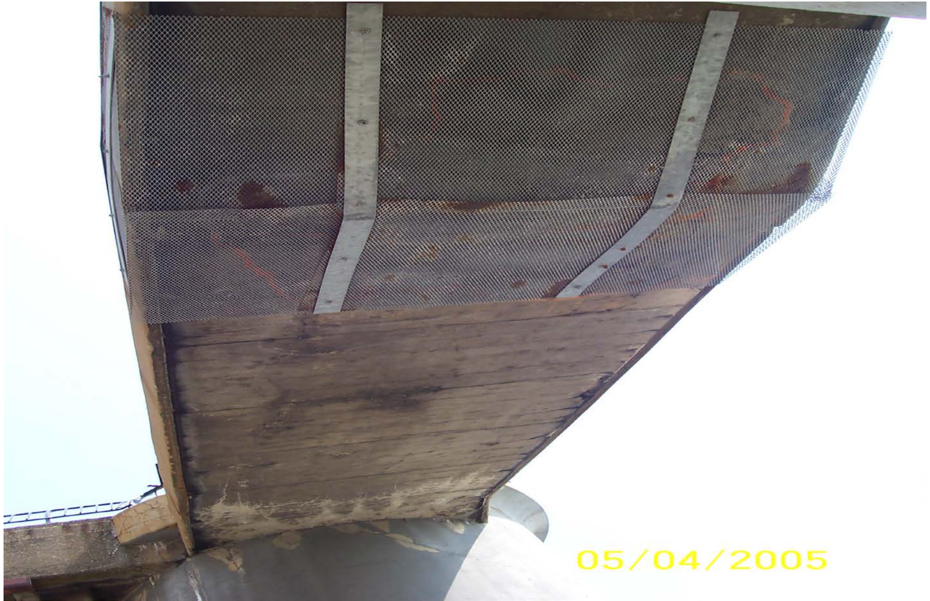
E 81st STREET BRIDGE – UNDER DECK DETERIORATION
