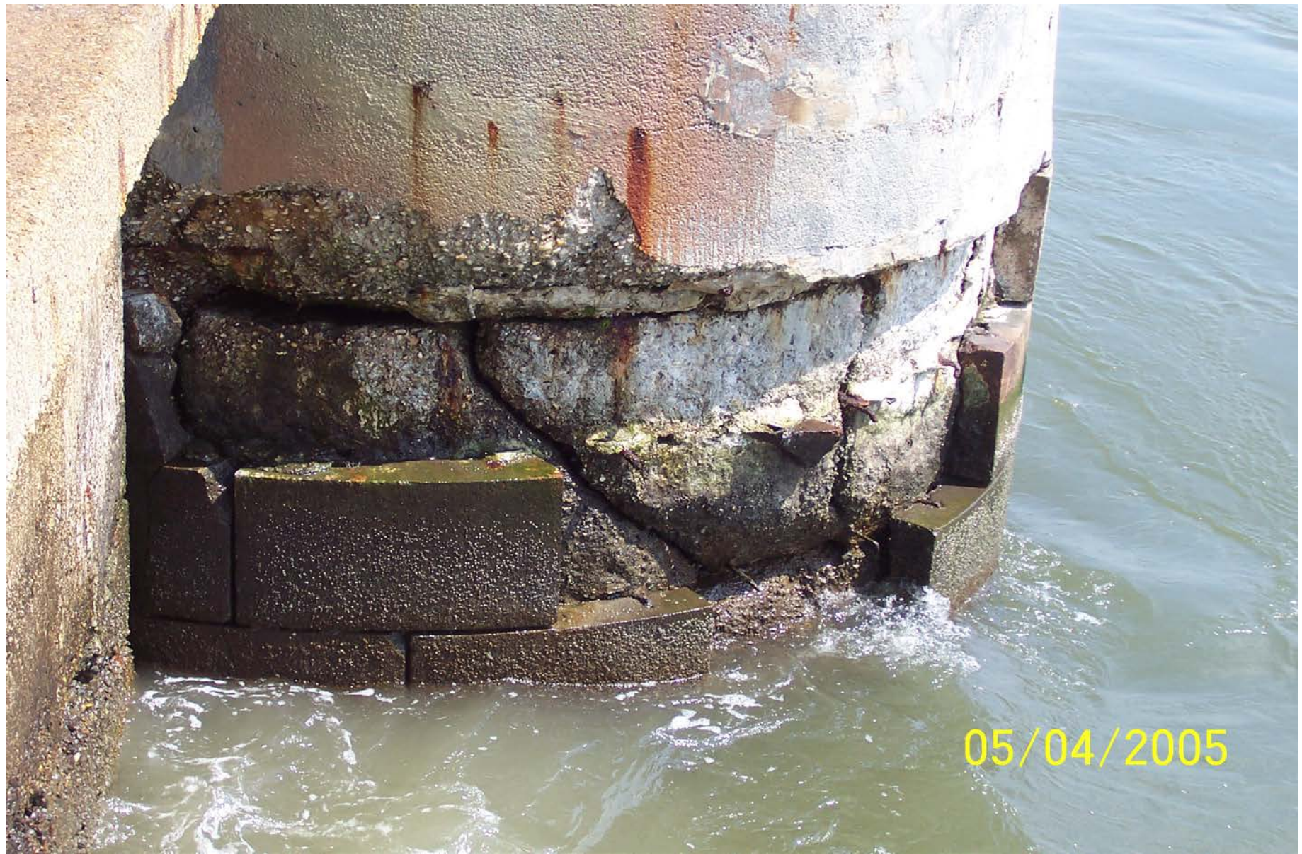
E 81st STREET BRIDGE – FOUNDATION DETERIORATION
