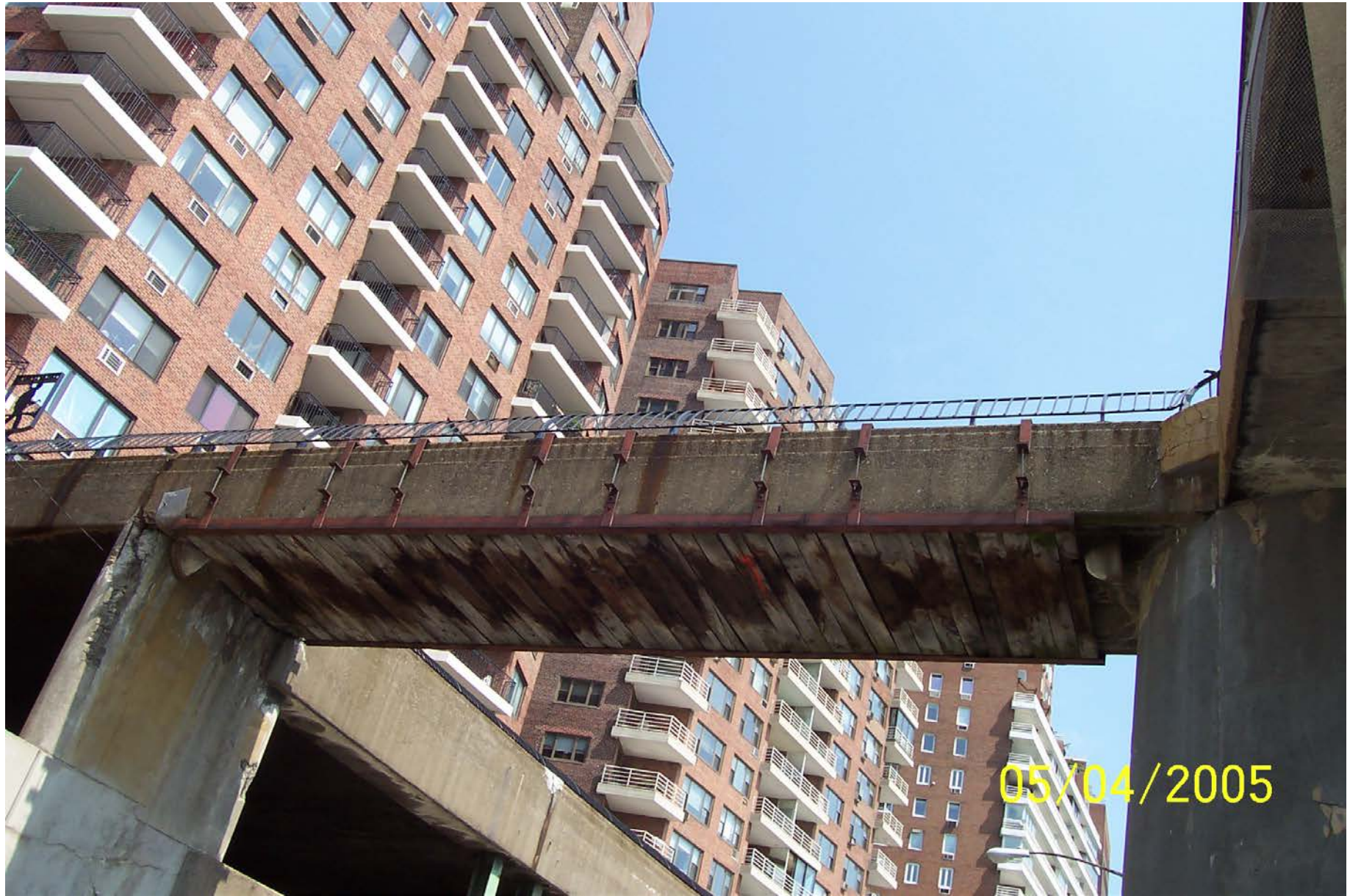
E 81st STREET BRIDGE – UNDERDECK SHIELD
